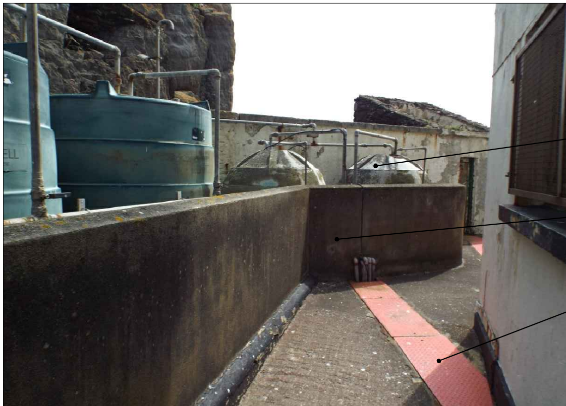
03 012 View of existing oil tanks & bund walls
