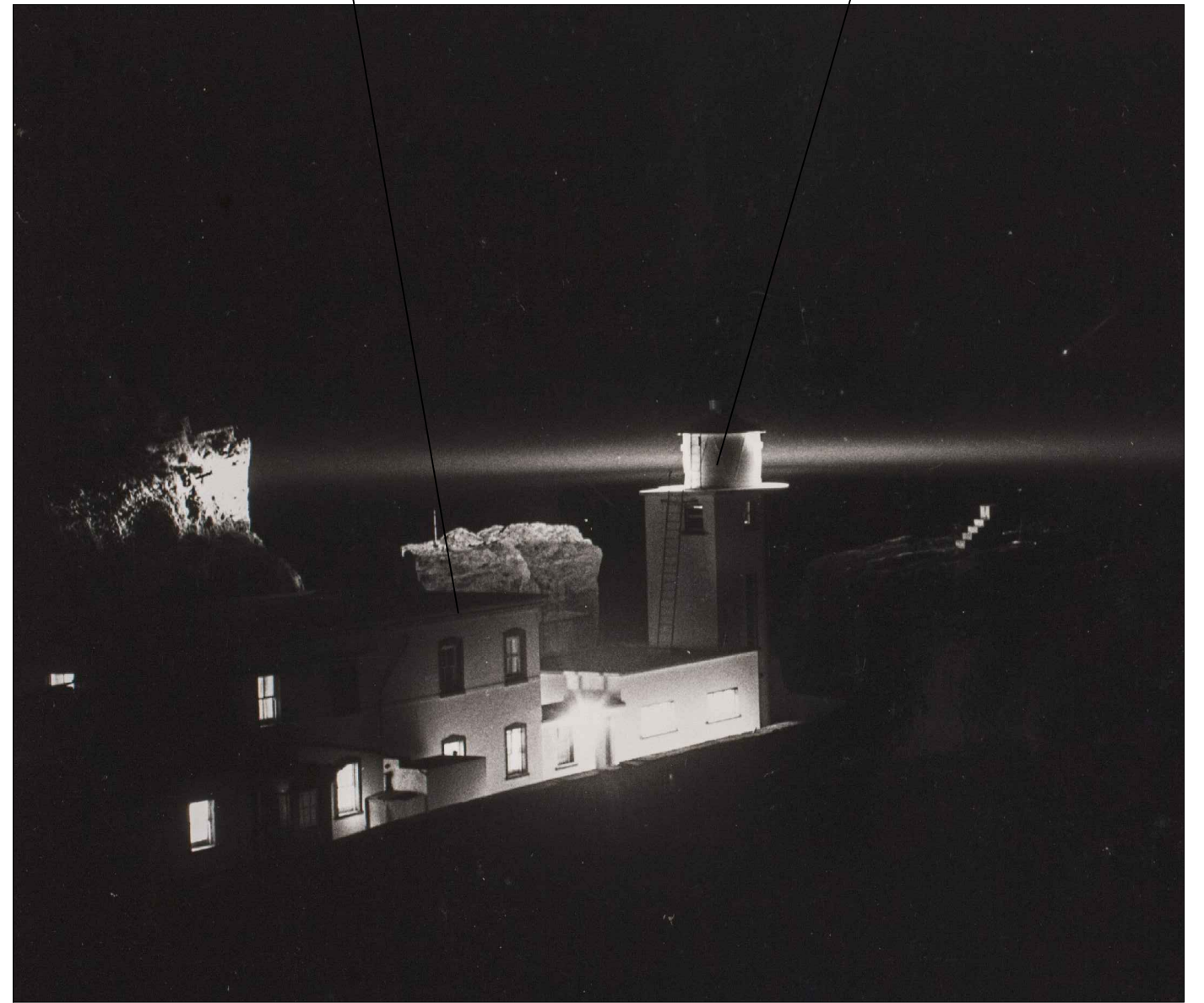
Archival image showing the renovated lighthouse at night time (1926-1949)
