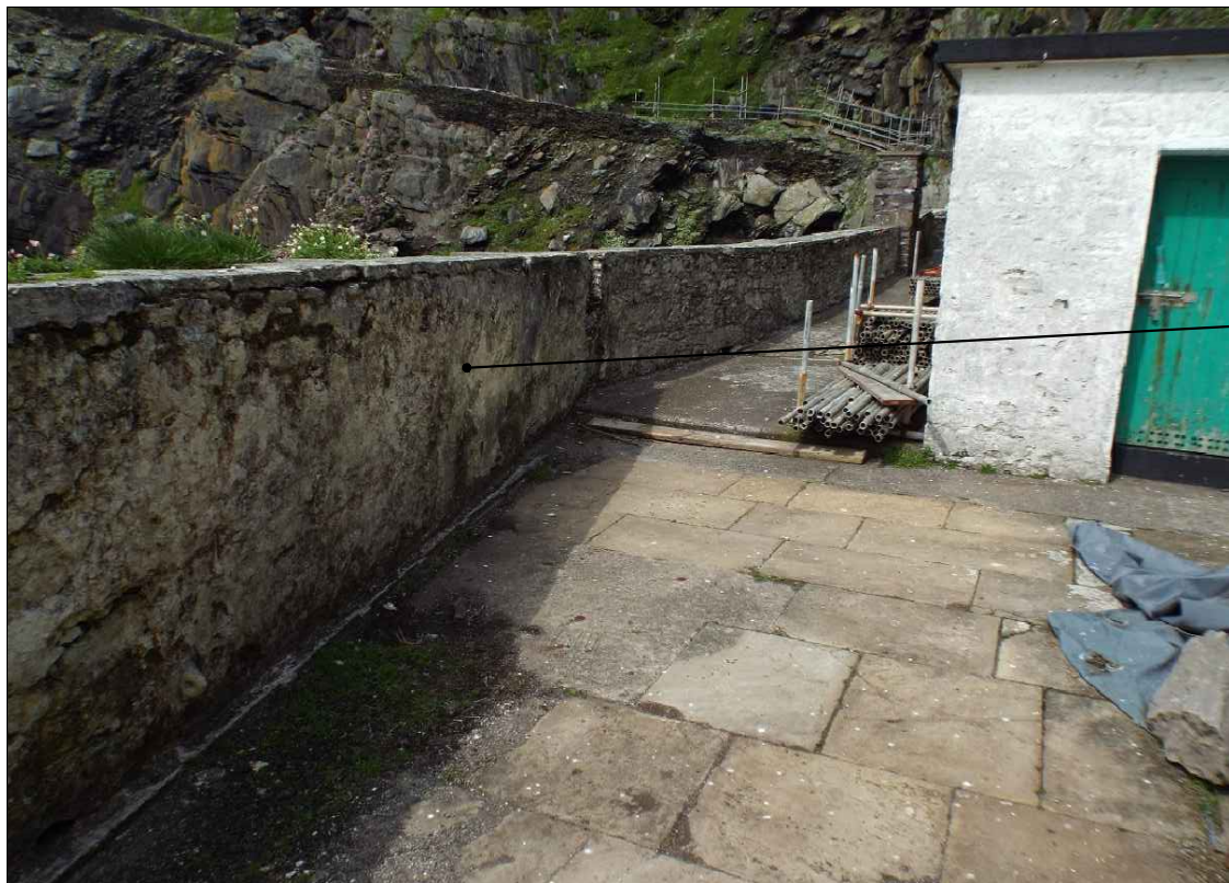
03 014 View of existing sea wall
