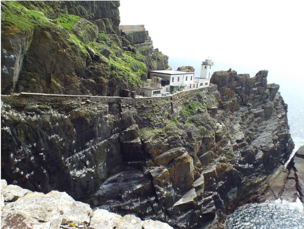
Figure 2: Image showing the lower lighthouse building from the upper lighthouse road
