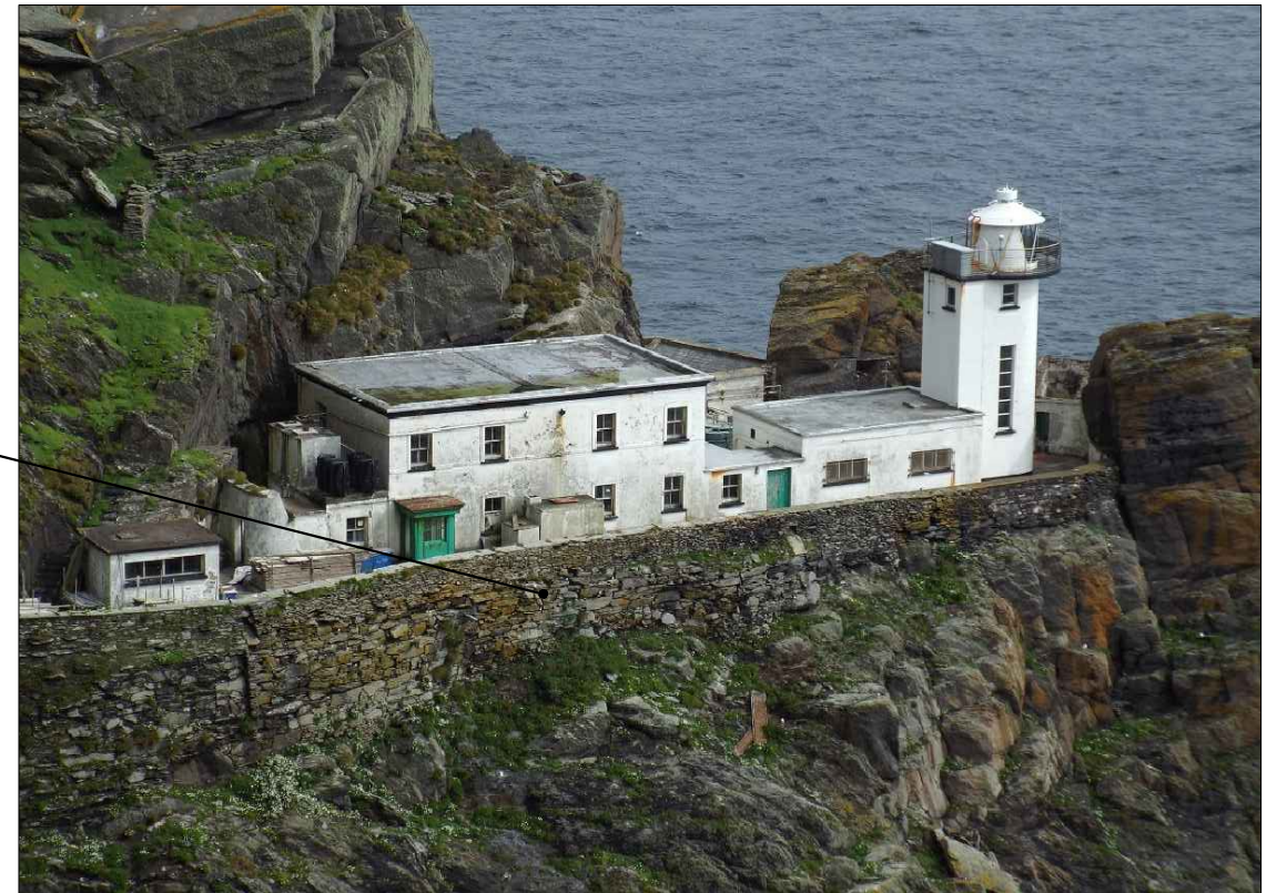
02 013 View of lower lighthouse & existing sea wall
