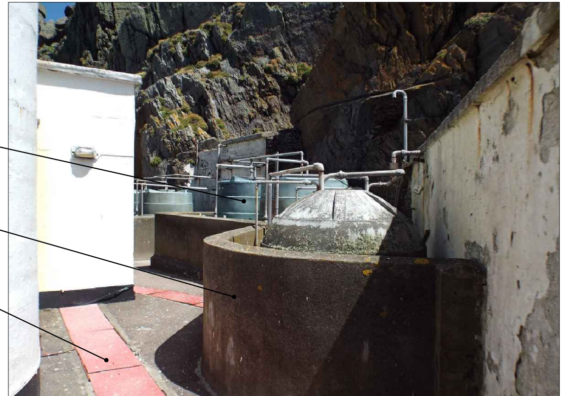
04 012 View of existing oil tanks & bund walls
