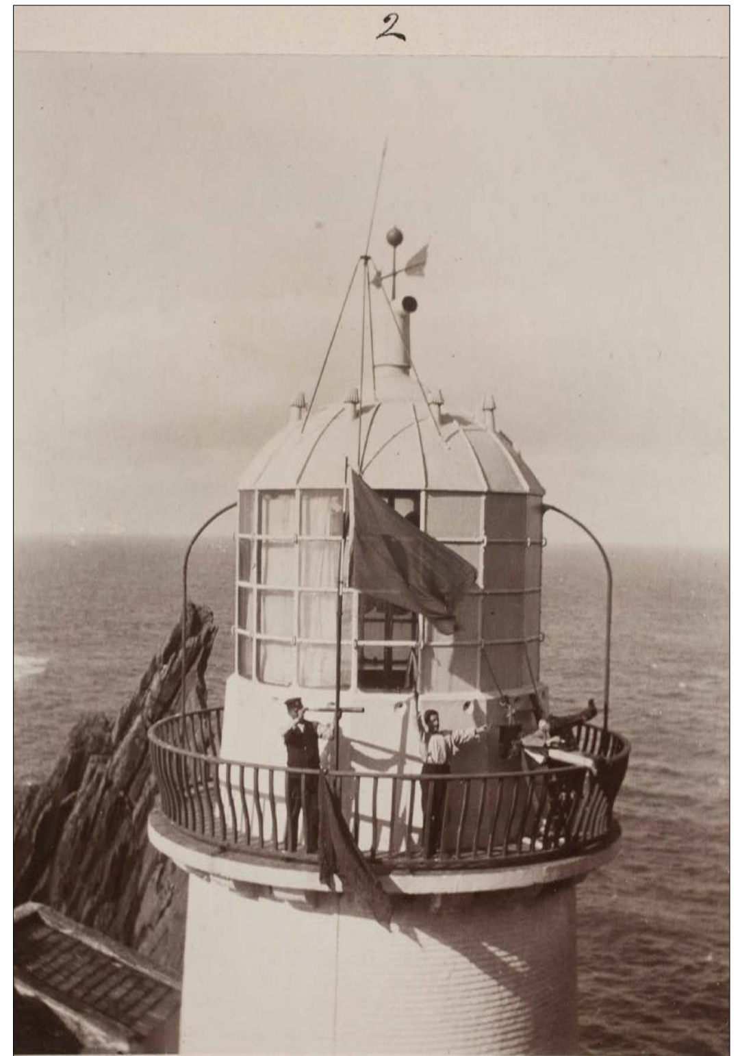
02 012 Archival image showing the lantern and keepers on the lower lighthouse (1905)
