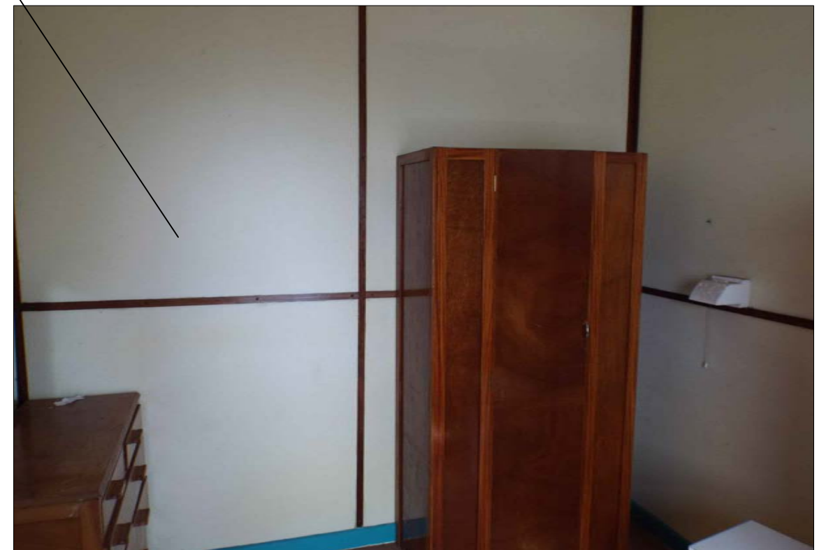
03 018 Internal image showing the existing dry lining
