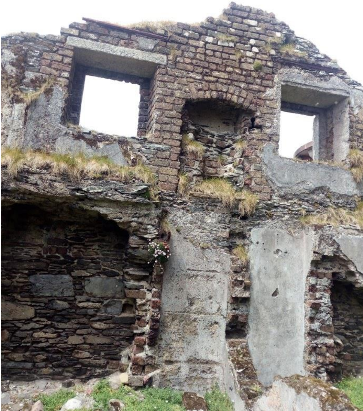
Fig. 4 – View of interior of lighthouse cottage.
