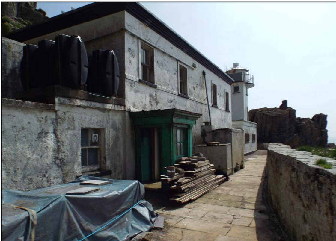
01 Image showing the main entrance to the lower lighthouse
