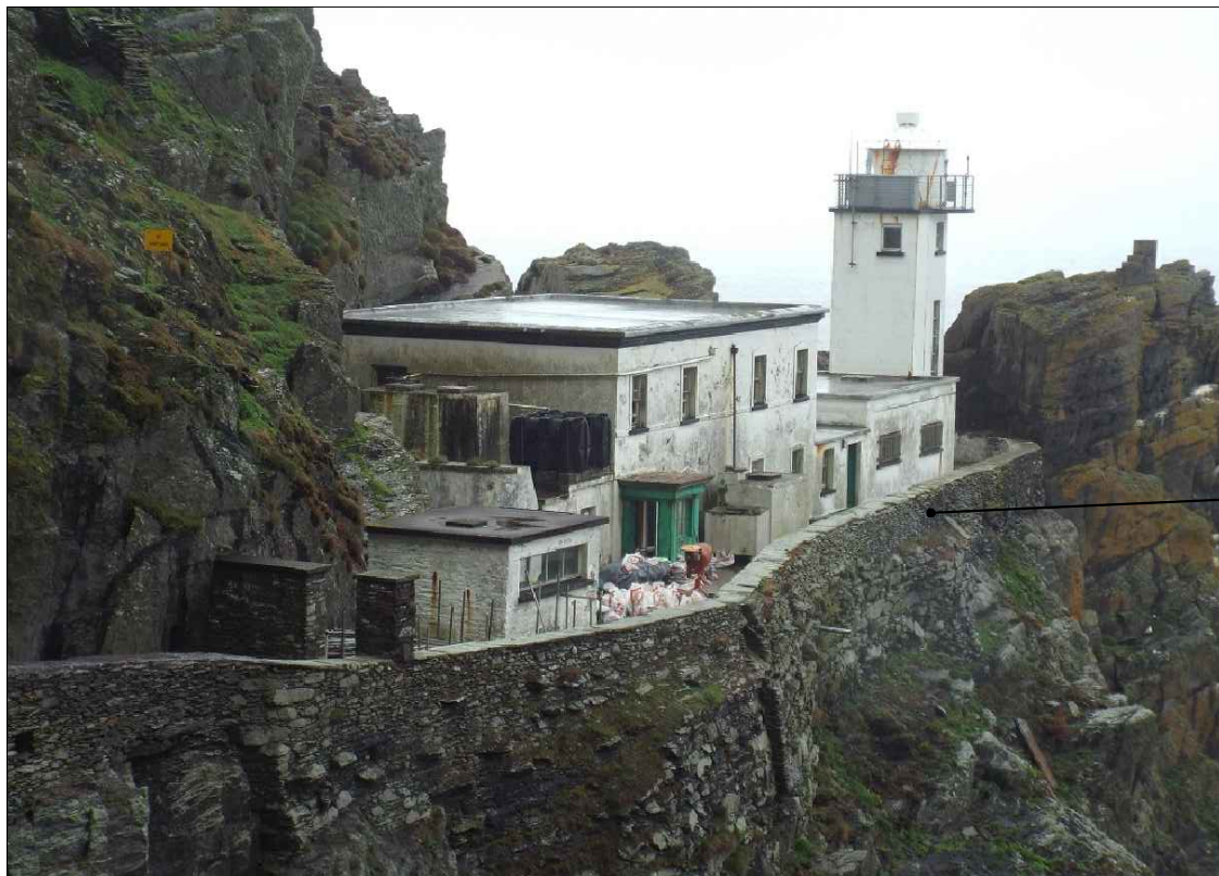
03 013 View of lower lighthouse & existing sea wall
