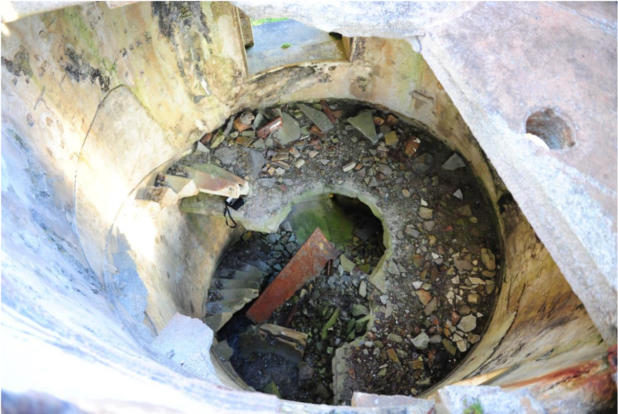
Fig. 8 – Interior view of ruined granite staircase from lantern room in 2012.
