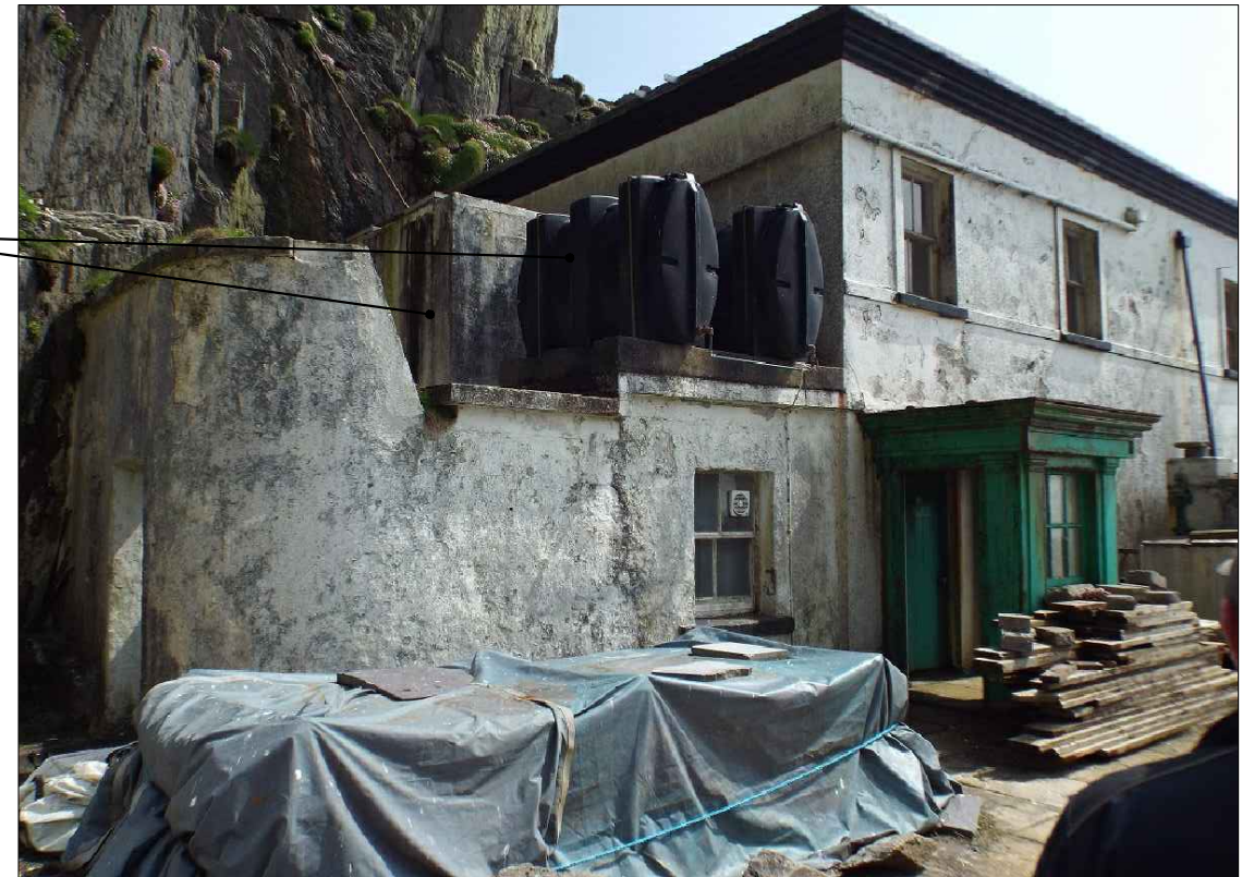
02 014 View of existing tanks on first floor
