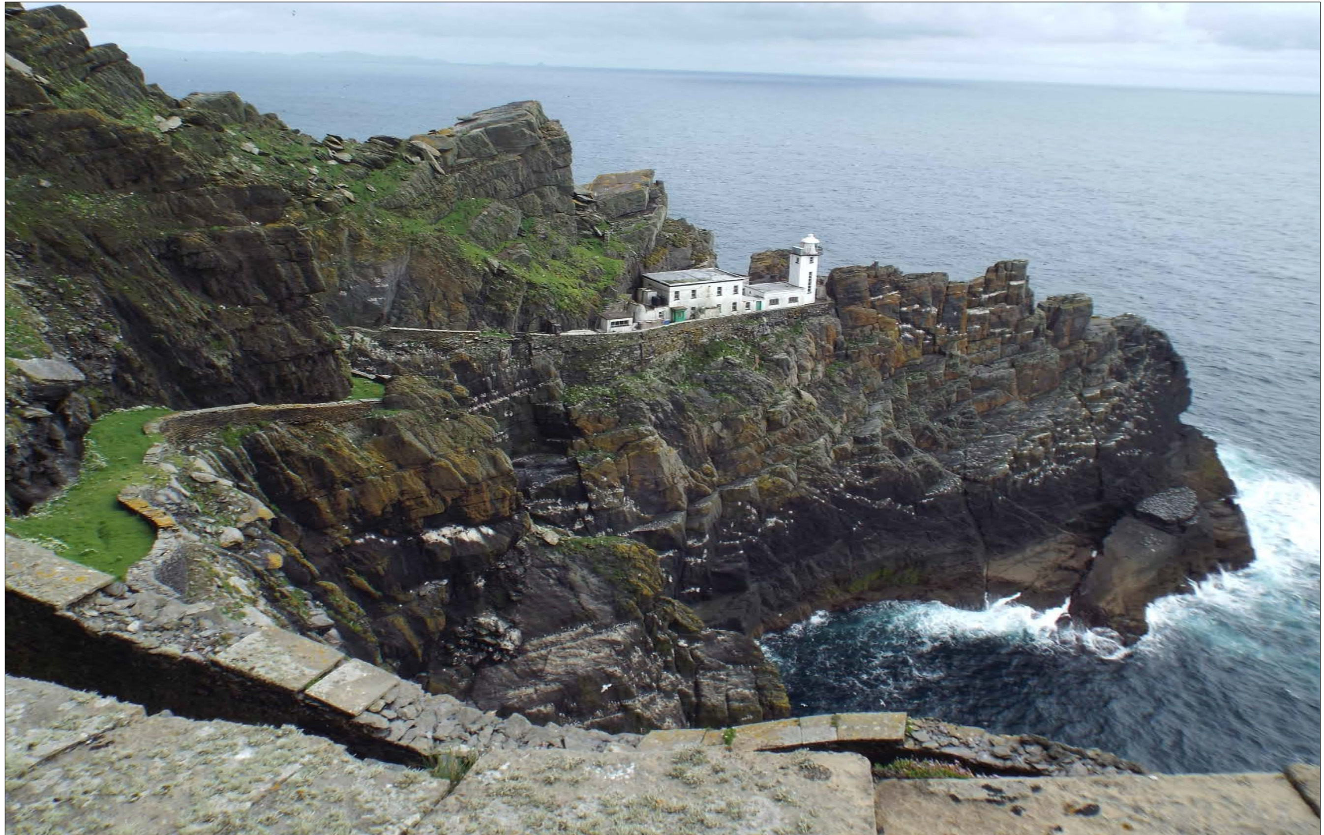
01 032 Image showing the existing lower lighthouse compound from the upper lighthouse road
