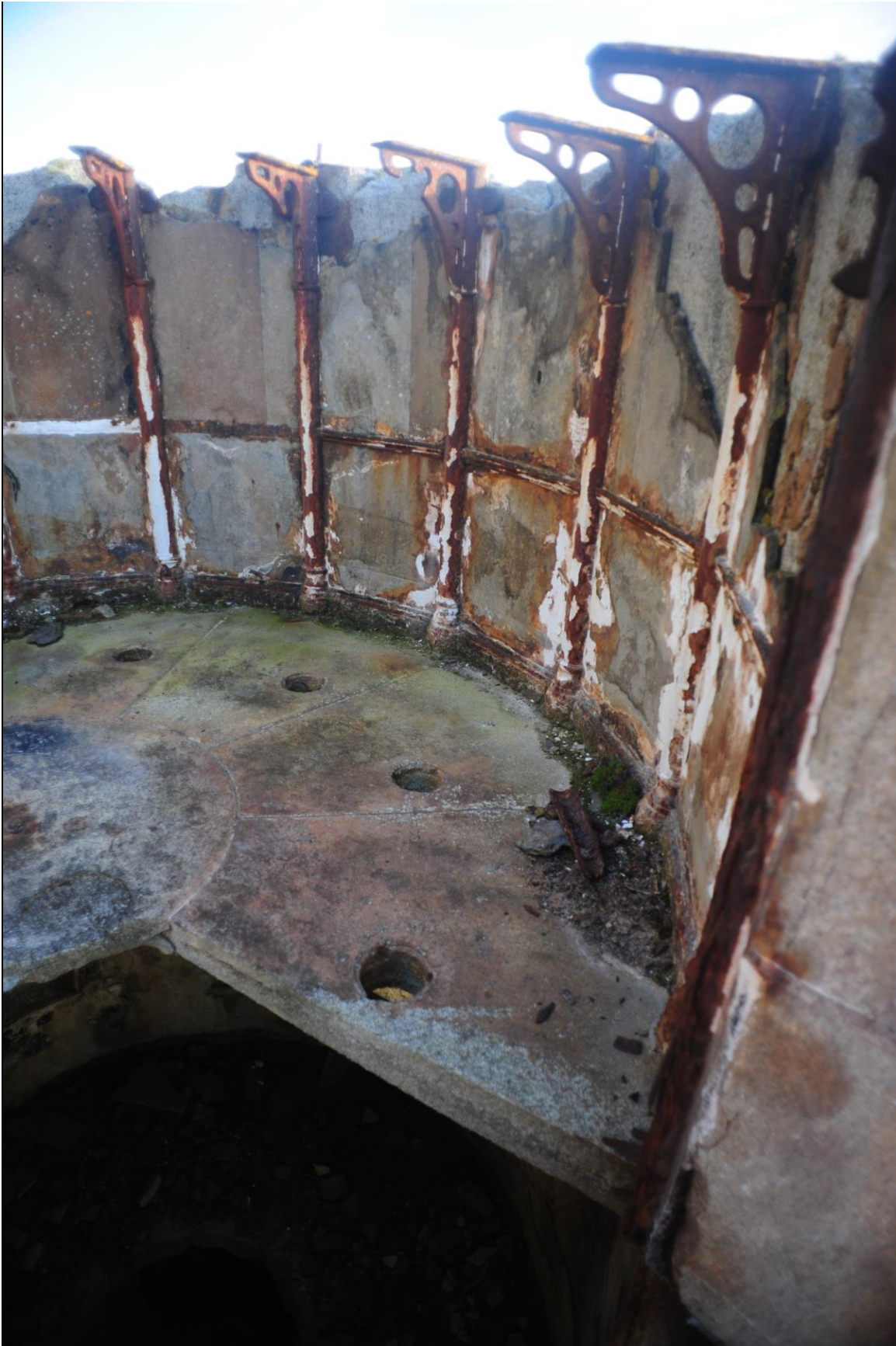
Fig. 11 – View of remains of lantern room of lighthouse tower in 2012.
