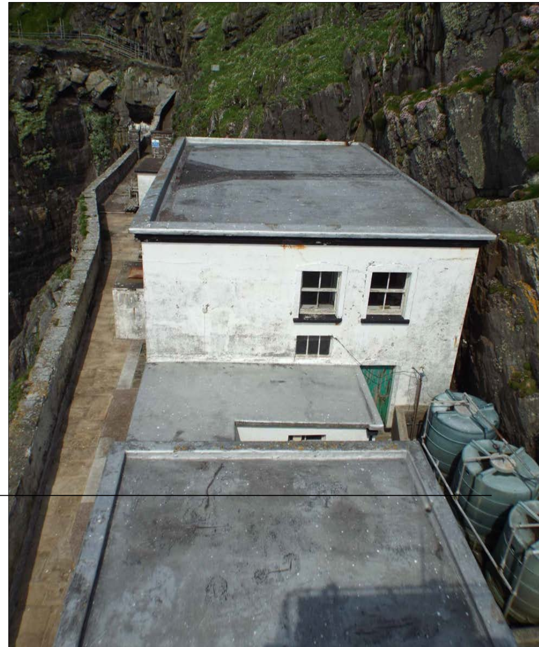
03 Image showing the flat rooftop of the current lower lighthouse
