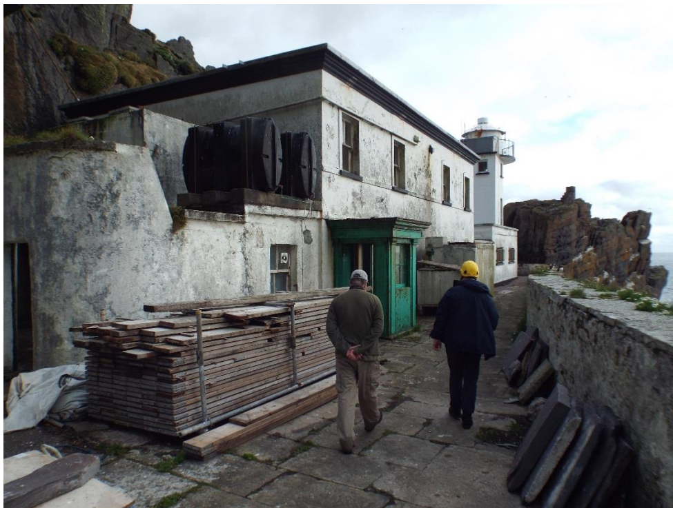
Figure 3: Image showing the entrance to the lower lighthouse building
