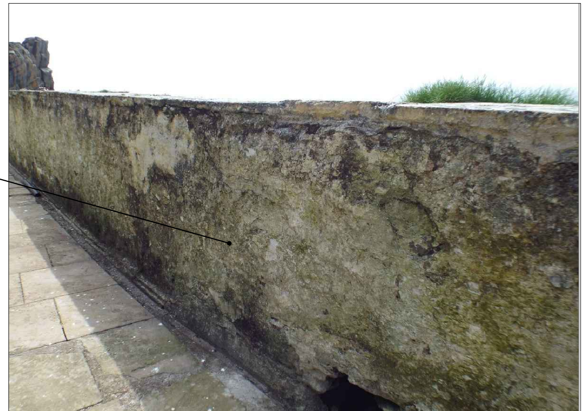
04 014 View of existing sea wall
