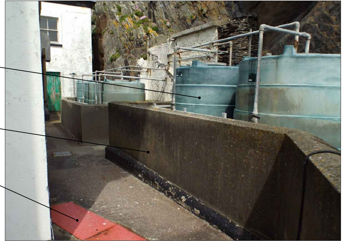
02 012 View of existing oil tanks & bund walls
