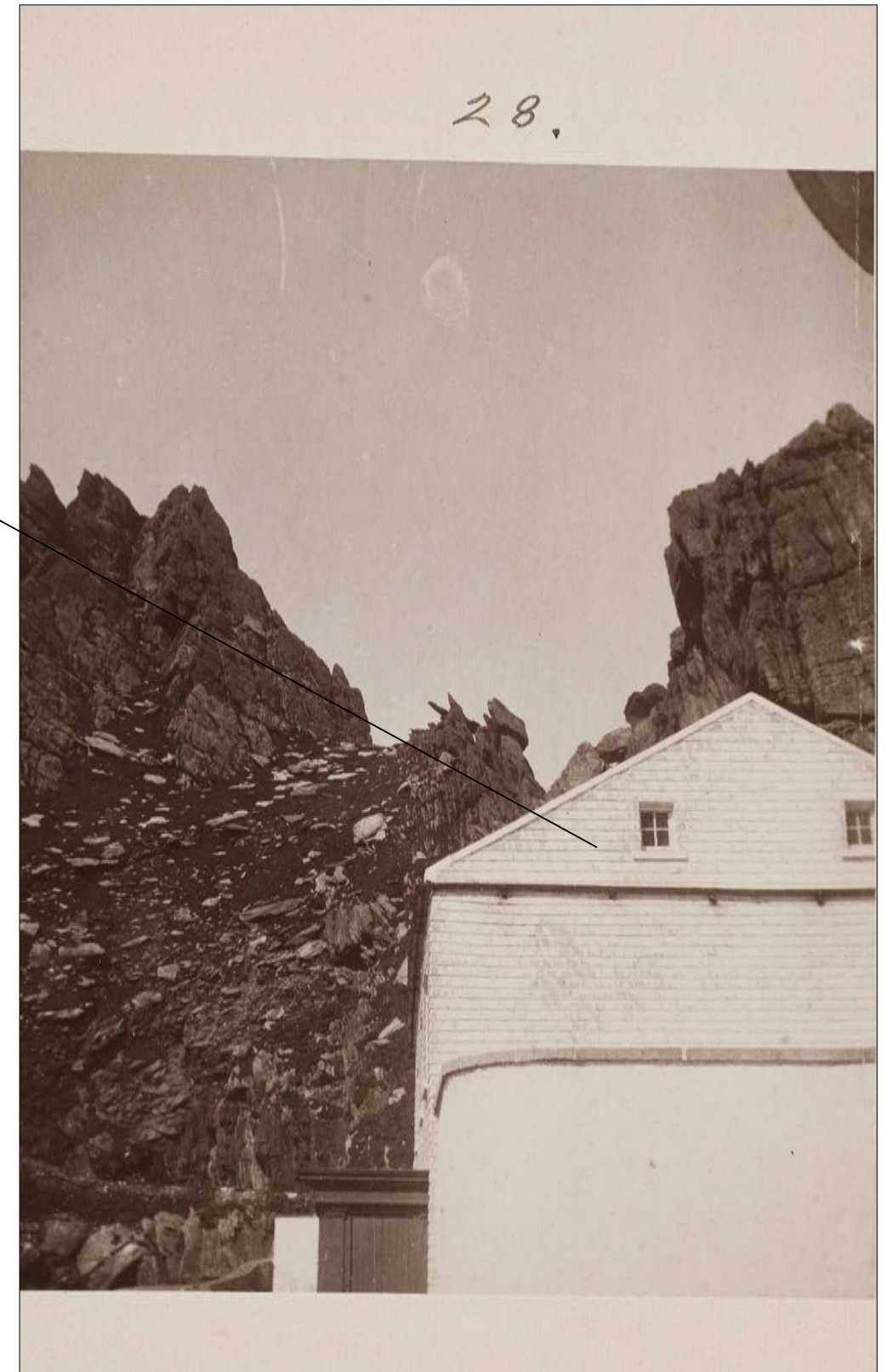
02 005 Archival image showing the original shape of the pitched roof before it was removed and replaced by a new concrete flat roof in 1910 (1905)
