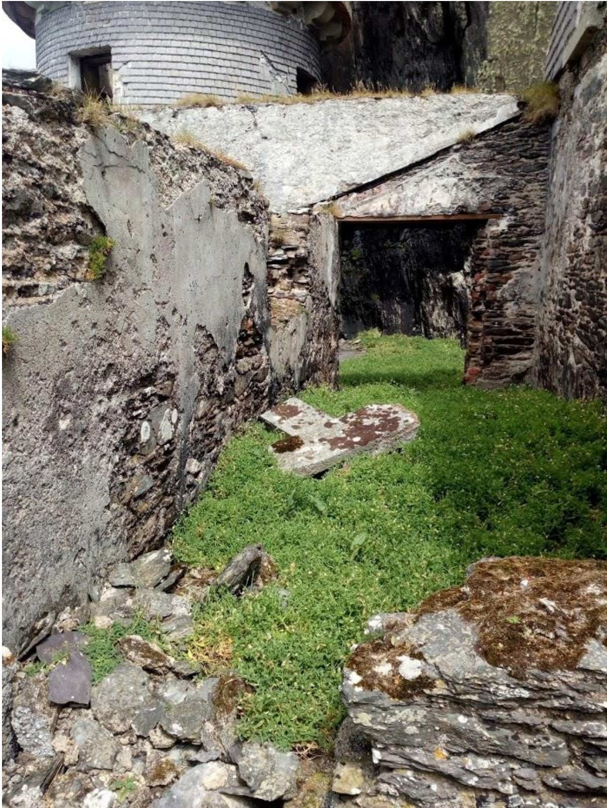
Fig. 6 – View of Interior of ancillary building.
