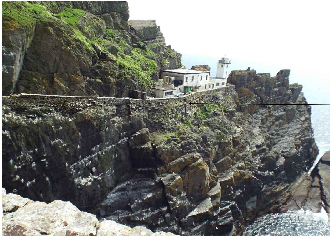
01 013 View of lower lighthouse & existing sea wall
