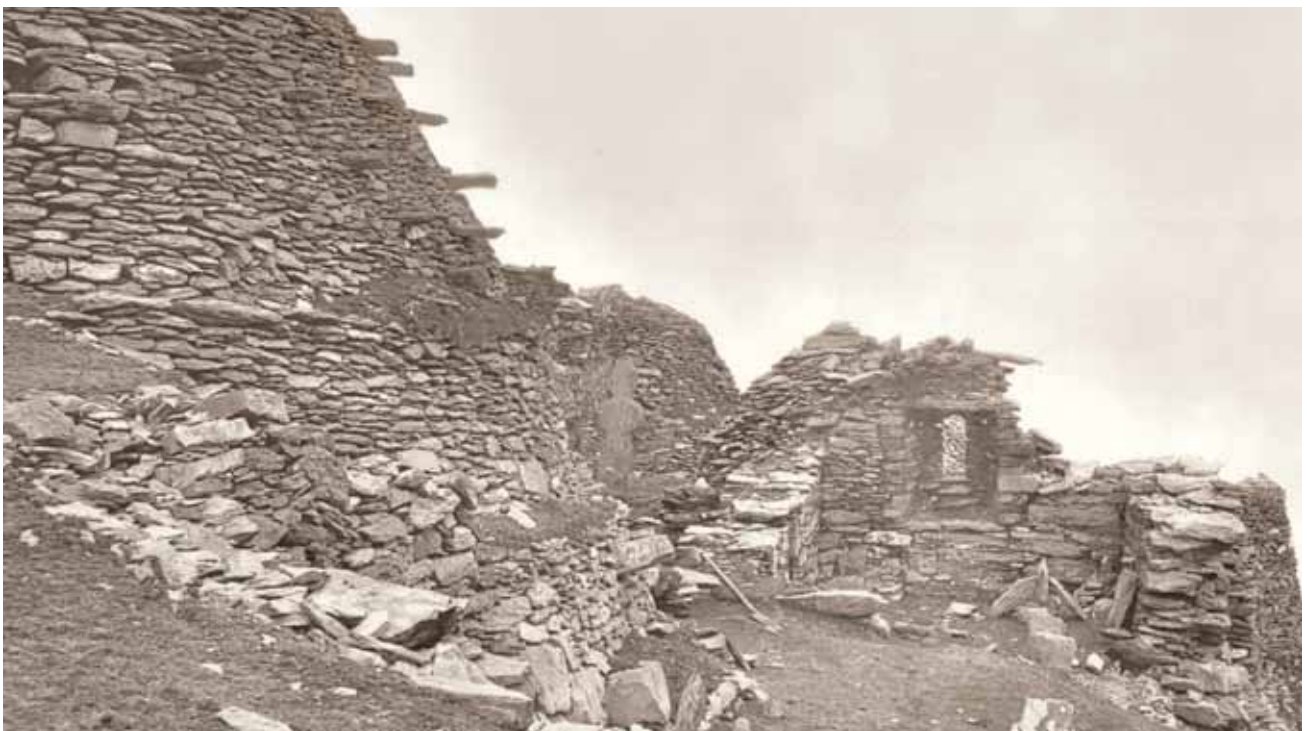
Pl. 7 - View of St Michael's Church, showing collapsed retaining wall on the south side, published in 'Notes on Irish Architecture'.
