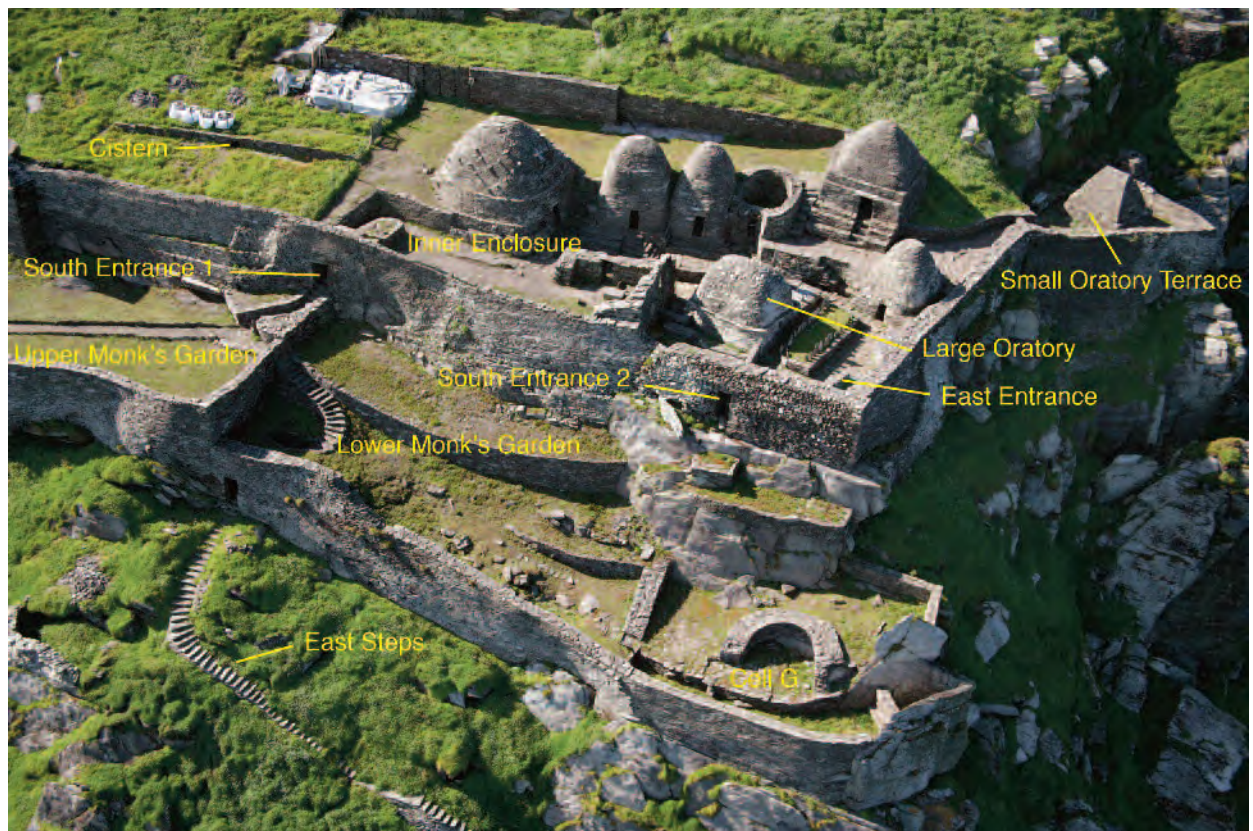
Pl. 4 Aerial view of the monastery, showing the Inner Enclosure (illustrating the location of cells, oratories, church and leachtanna in the Lower Outer Enclosure). This view also shows the top of the East Steps and the original entrance to the monastery.
