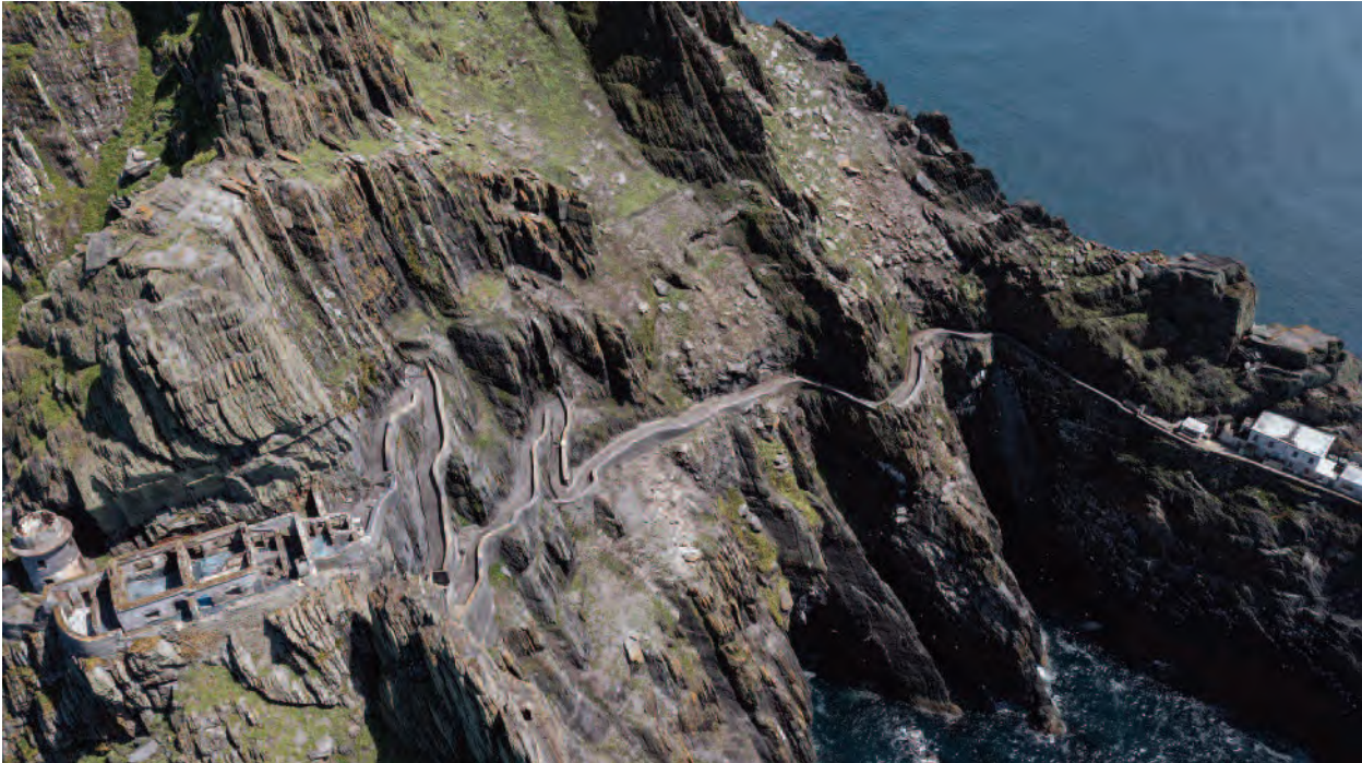
Pl. 66 The Upper and Lower Lighthouses and and Upper Lighthouse Road.
