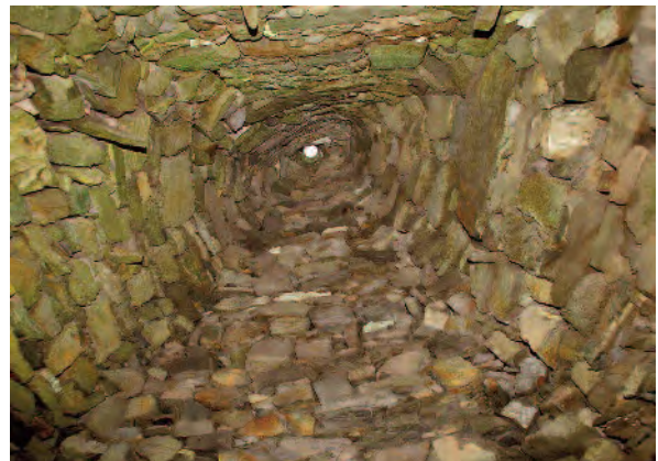
Pl. 45 The inner dome of Cell F, showing corbelling and projecting stones.
