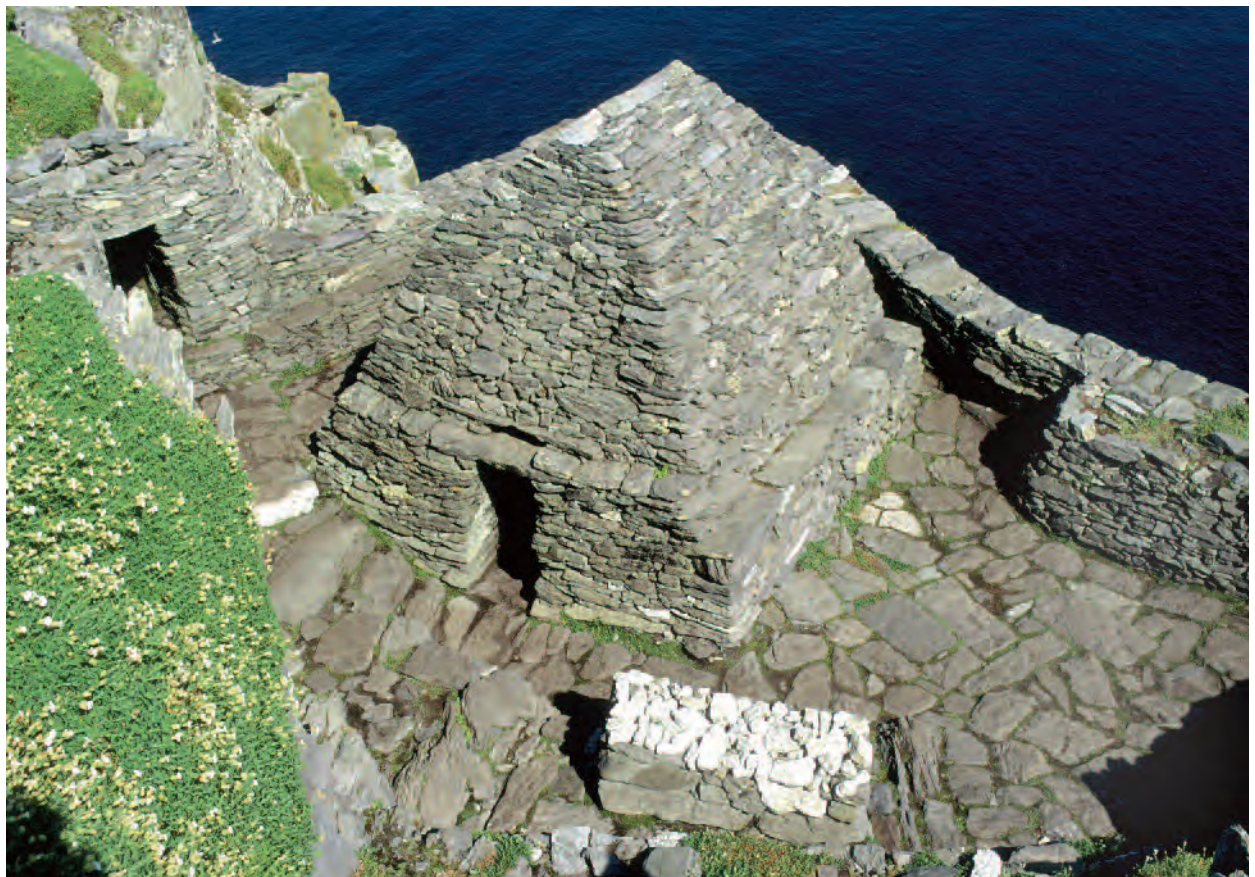
Pl. 59 The Small Oratory Terrace after excavation, consolidation and conservation works.
