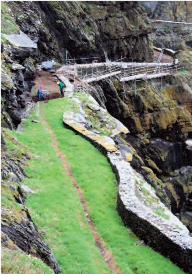
Pl. 30 The Upper Lighthouse Road covered with material deposited from above (excavations ongoing in background).
