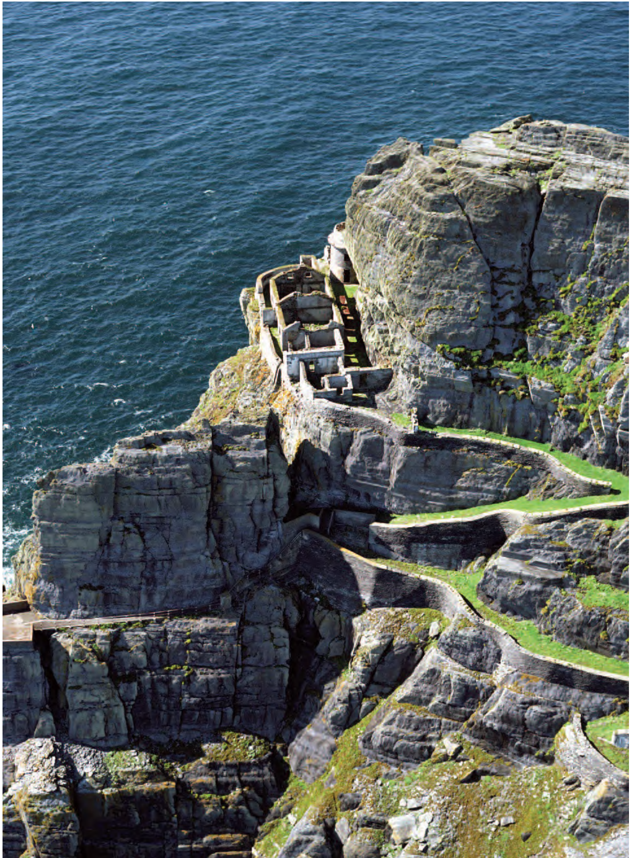
Pl. 29 A view of the Upper Lighthouse and the Upper Lighthouse Road before archaeological excavation and conservation works to the road.
