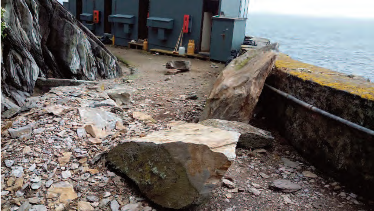
Pl. 26 Rockfall close to staff accommodation.
