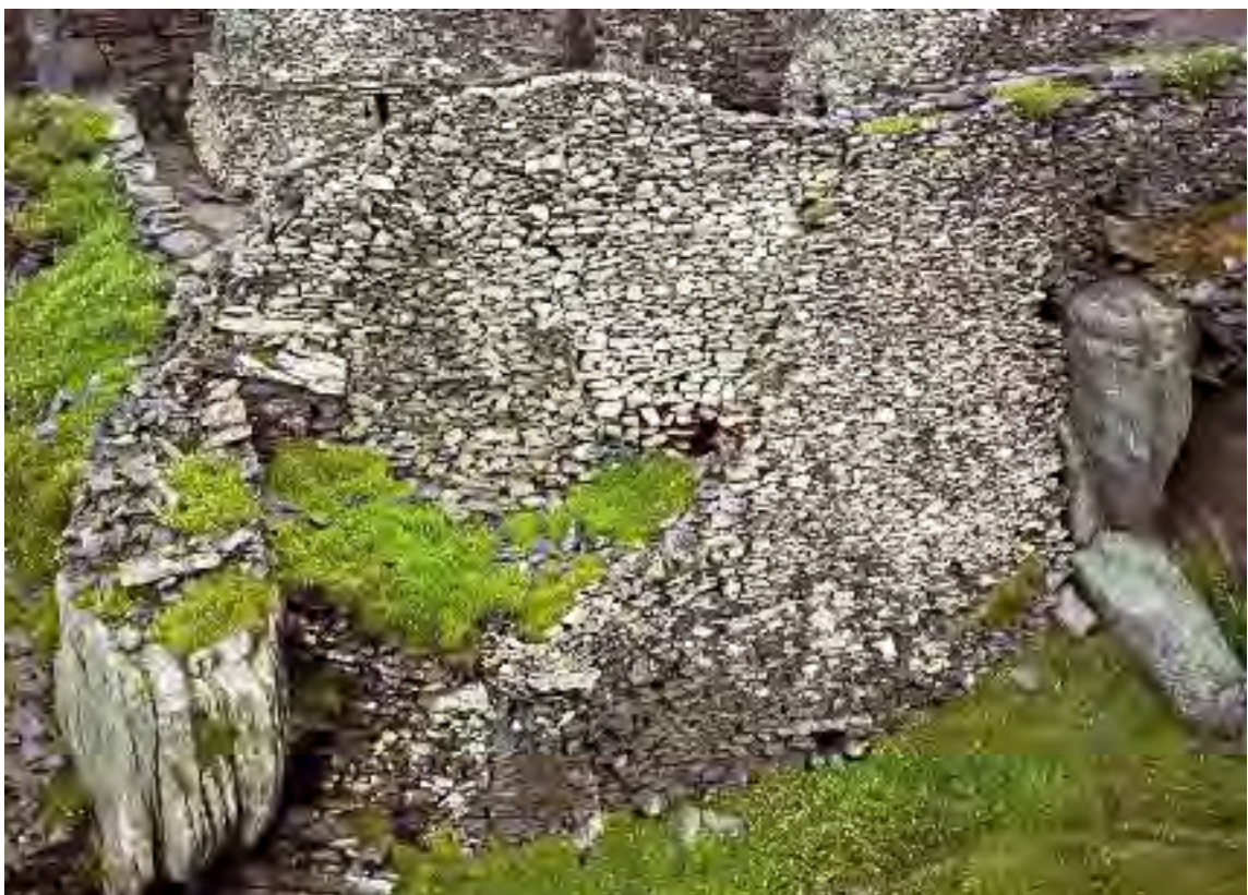
Ill. 2.73—Entrance area from east, showing wall collapse (Con Brogan, DAHG).
