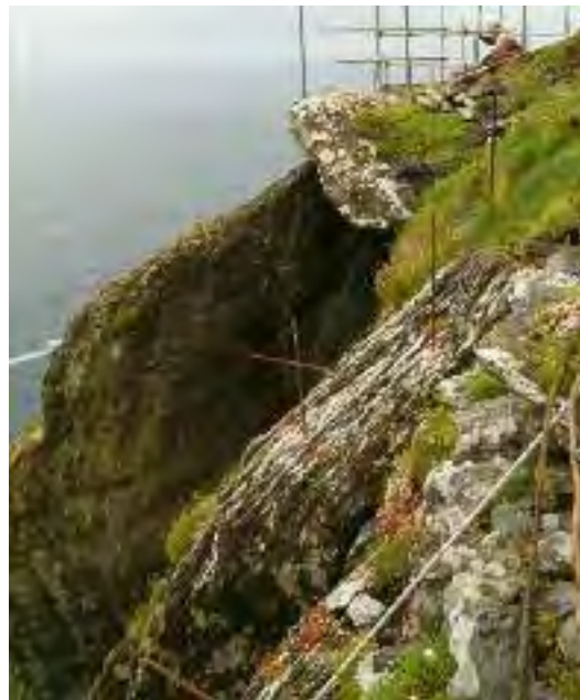
[Right] Ill. 2.401—The collapsed upper bridging stone over the gully viewed from the north-east before excavation (A.R. Hayden).
