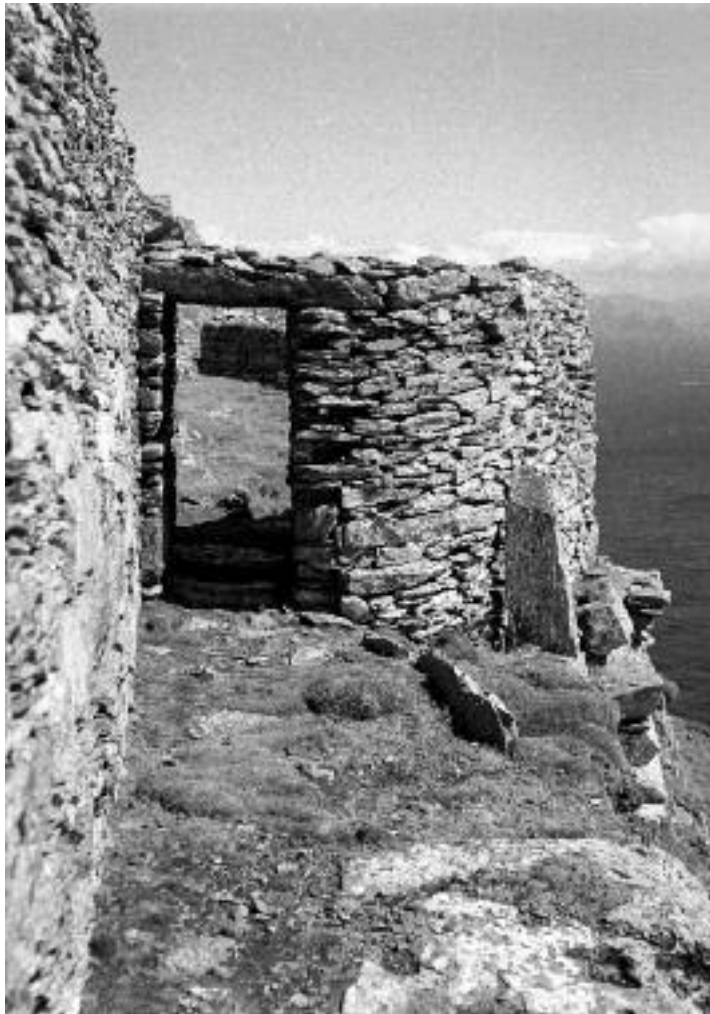
Ill. 2.134—The nineteenth-century entrance in the 1950s (DAHG Archive).
