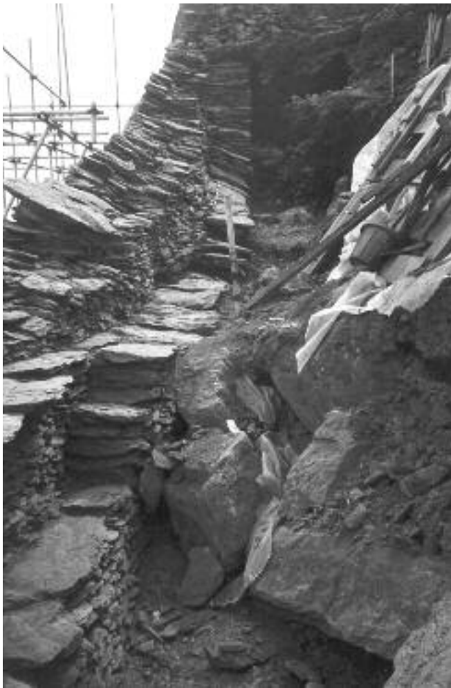
Ill. 2.107— Boulders and F640 from east, showing the boulders collapsed against the interior of F640 and the resulting distortion of the wall (E. Bourke).
