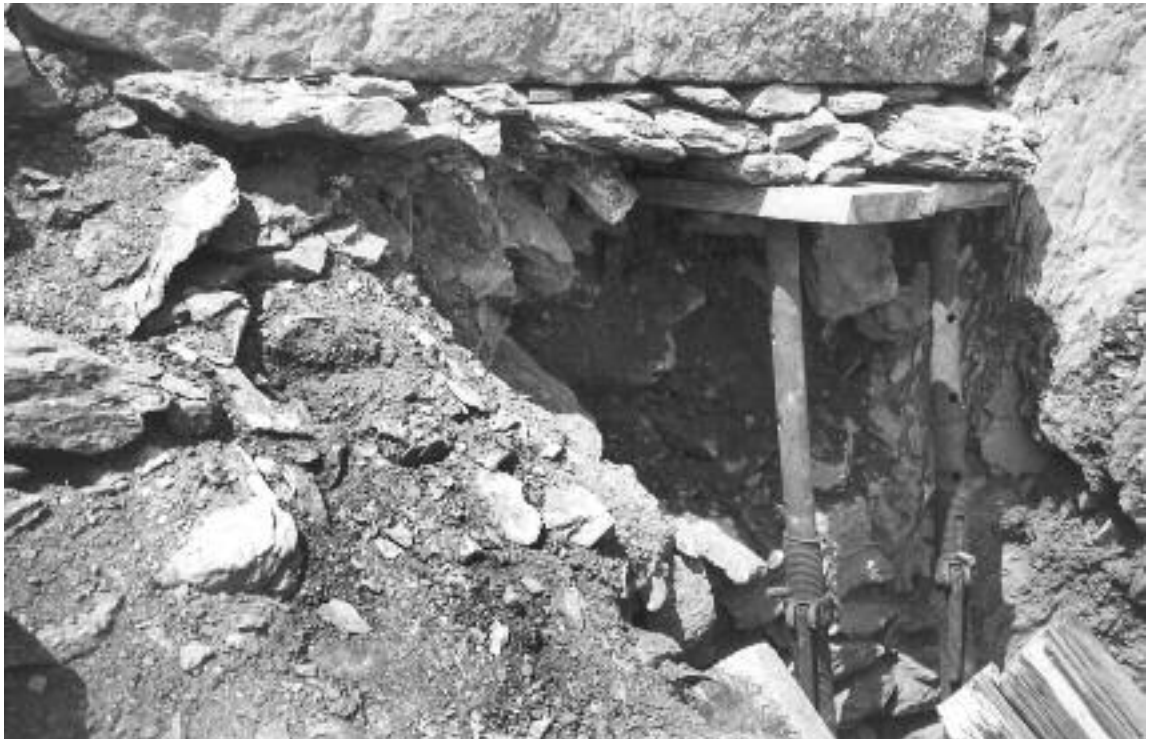
III. 2.104—Base of wall of inner enclosure, directly below St Michael's Church, showing 1890s rebuild directly onto unsorted rubble (E. Bourke).
