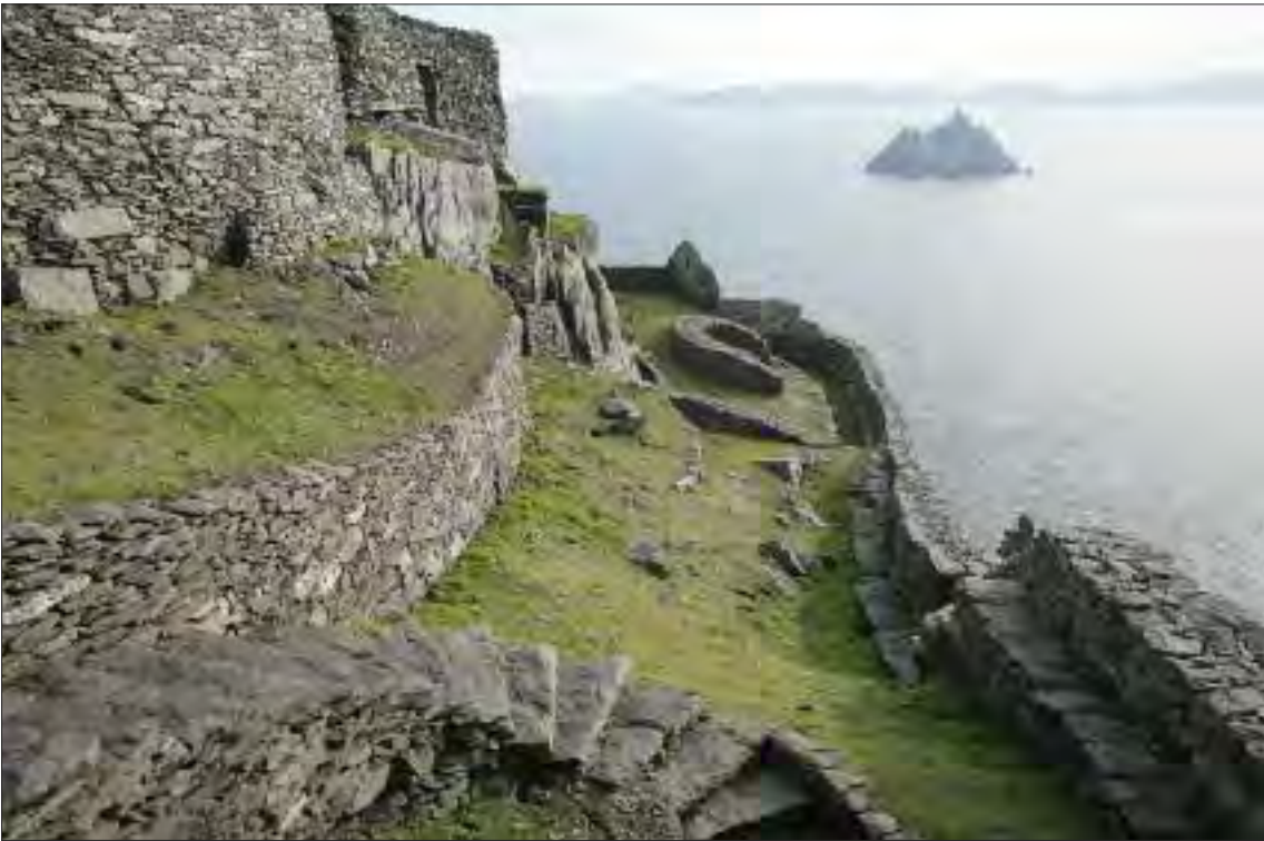
Ill. 2.116— Lower monks' garden after conservation, showing stones of boulder layer left in situ (Con Brogan, DAHG).
