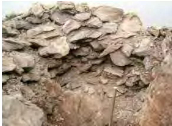
[Left] Ill. 2.370—The inward slumping of the wall at the northern end of the terrace, with the reinforcing wall at its base (A.R. Hayden).
