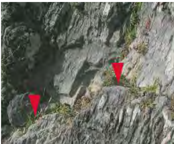
Ill. 2.298—The left-hand side of the ledge crossing the gully, with a possible step (5) in the deep notch on the left and another (6) on the flat-topped rock spine at the centre (photo: A.R. Hayden).
