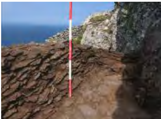
[Right] Ill. 2.460—The top of the masonry steps at the northern end of the upper traverse leading to the climb to the top of the Peak (A.R. Hayden).
