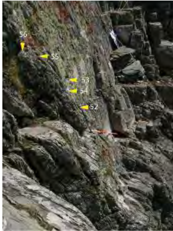
Ill. 2.316—The rock-cut handholds where the route turns back into the gully (A.R. Hayden).
