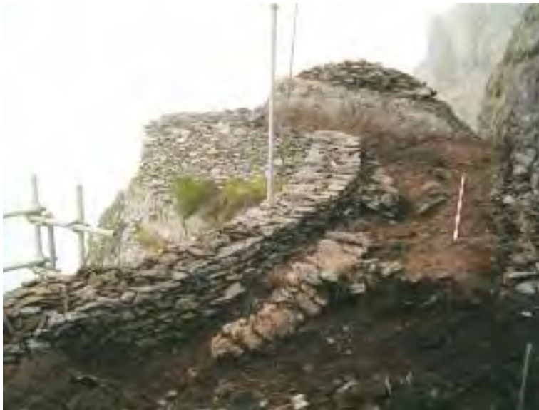
Ill. 2.373—The reinforcing wall viewed from the south-east (A.R. Hayden).
