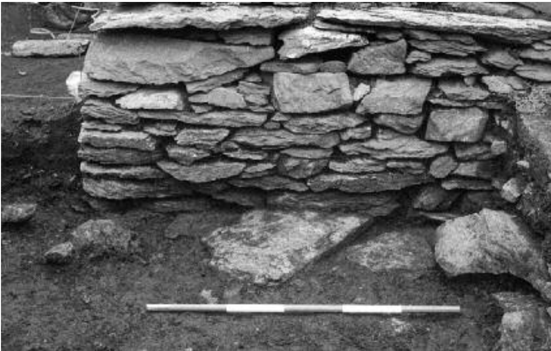
Ill. 2.24—Paving stones (F220) on south side of the small oratory (A. Lynch).
