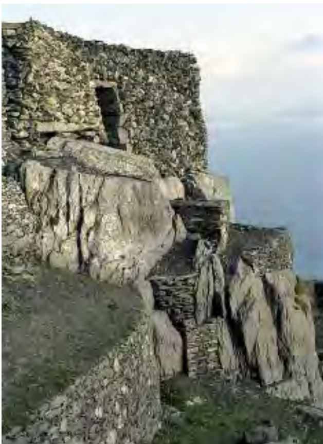
Ill. 2.54—South entrance I after conservation (Con Brogan, DAHG).
