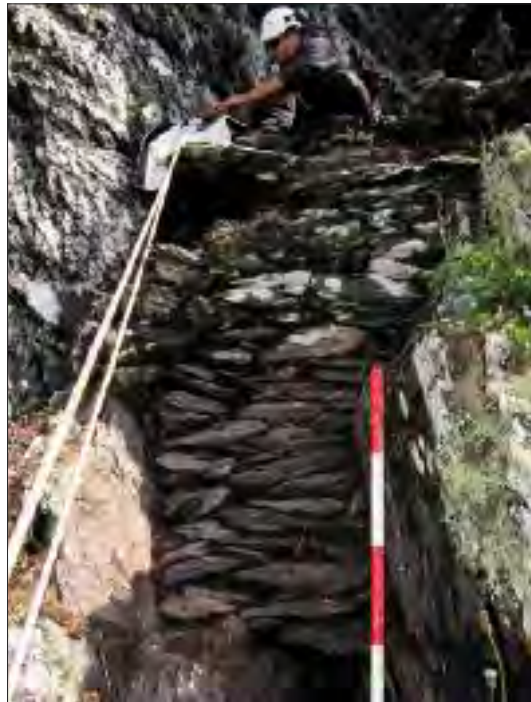
Ill. 2.451—The base of the external face of the terrace wall rose and fell considerably, as it was erected crossing deep fissures, which gave the wall a secure foundation. The ranging rod lies in the same position as that in the preceding photograph (A.R. Hayden).
