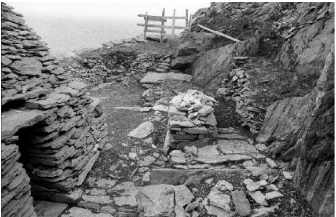
III. 2.16—The small oratory terrace, viewed from north, during excavation (A. Lynch).
