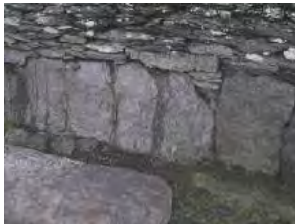
[Below] Ill. 2.413—Base of the north wall of the oratory. The upright rock on the left is bedrock; two upright stones support the wall on the right. Note the grooves in the top of the bedrock, which channel water down to the drain (A.R. Hayden).
