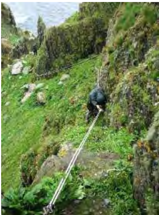
[Left] Ill. 2.576—Looking down along the rock-cut steps and masonry (8) to terrace (7) and gully (6) (A.R. Hayden).
