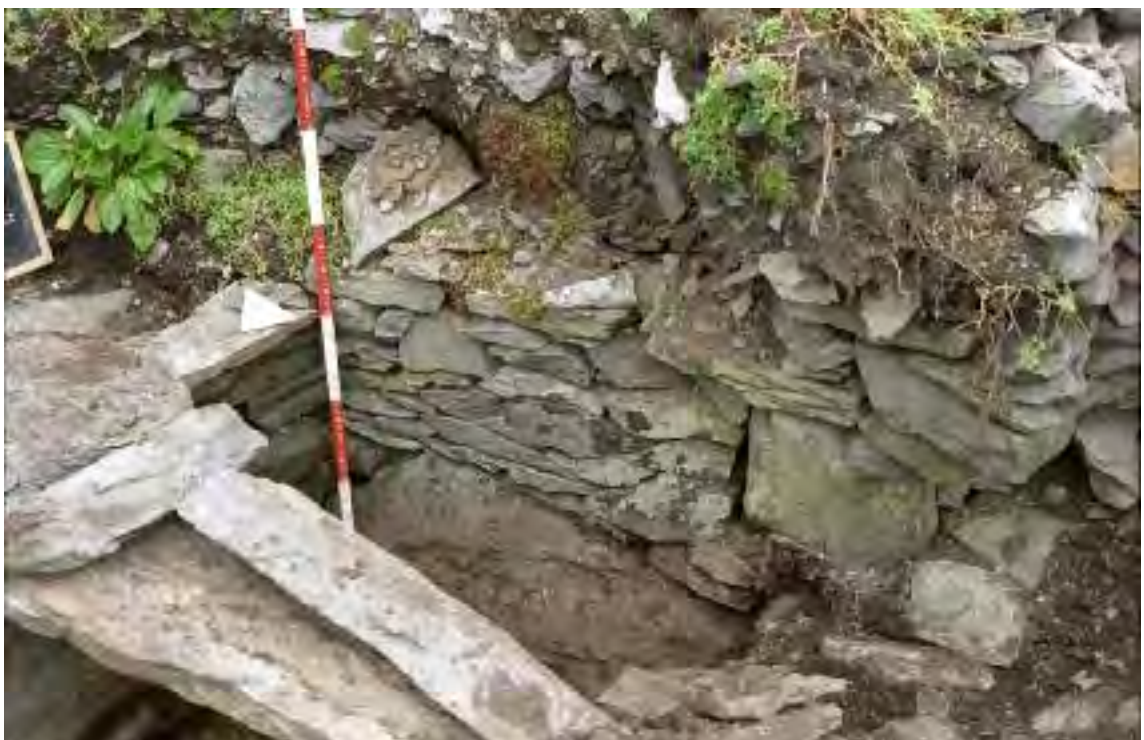
Ill. 2.82—East end of cistern with most of the lintels removed (A. Halm Schlag).
