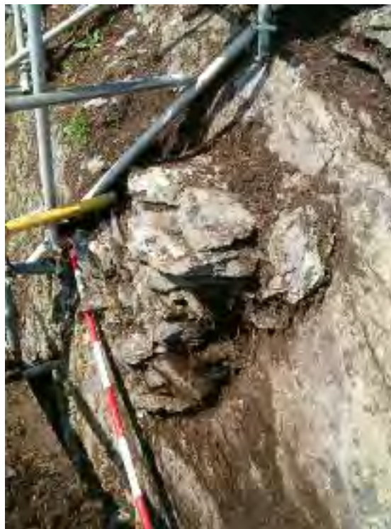
III. 2.397—The hauling platform. Note hollow cut in rock ledge to secure its base (A.R. Hayden).
