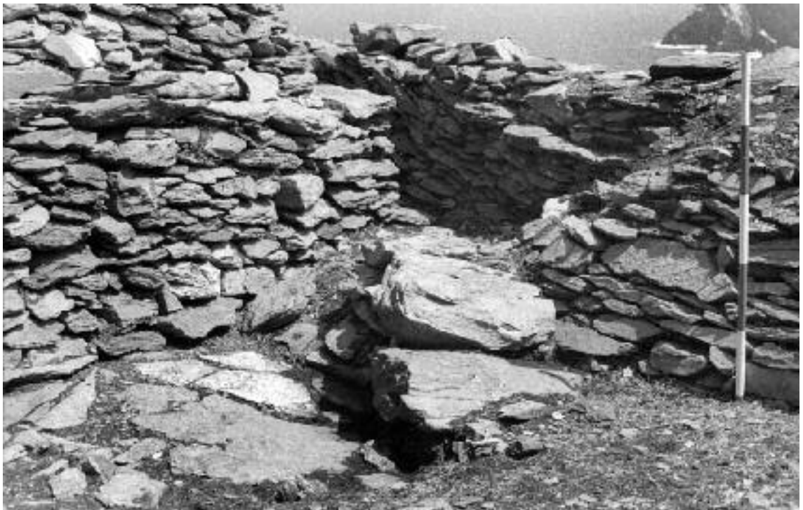
III. 2.28—Rudimentary steps and revetment to retaining wall visible on right (A. Lynch).
