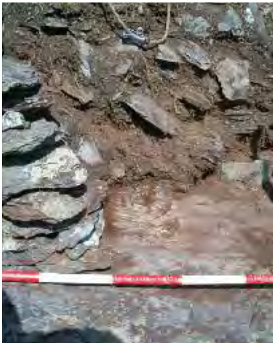
III. 2.396—Hollow cut on rock ledge to secure foundations at east end of eastern section of outer walling (A.R. Hayden).
