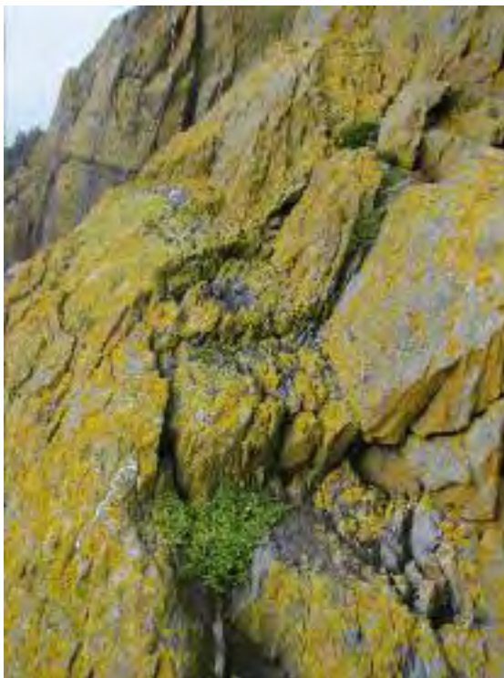
[Right] III. 2.551—The finely carved lower end of the earlier lighthouse steps. These steps retain tooling identical to that on the later lighthouse steps (photo: A.R. Hayden).
