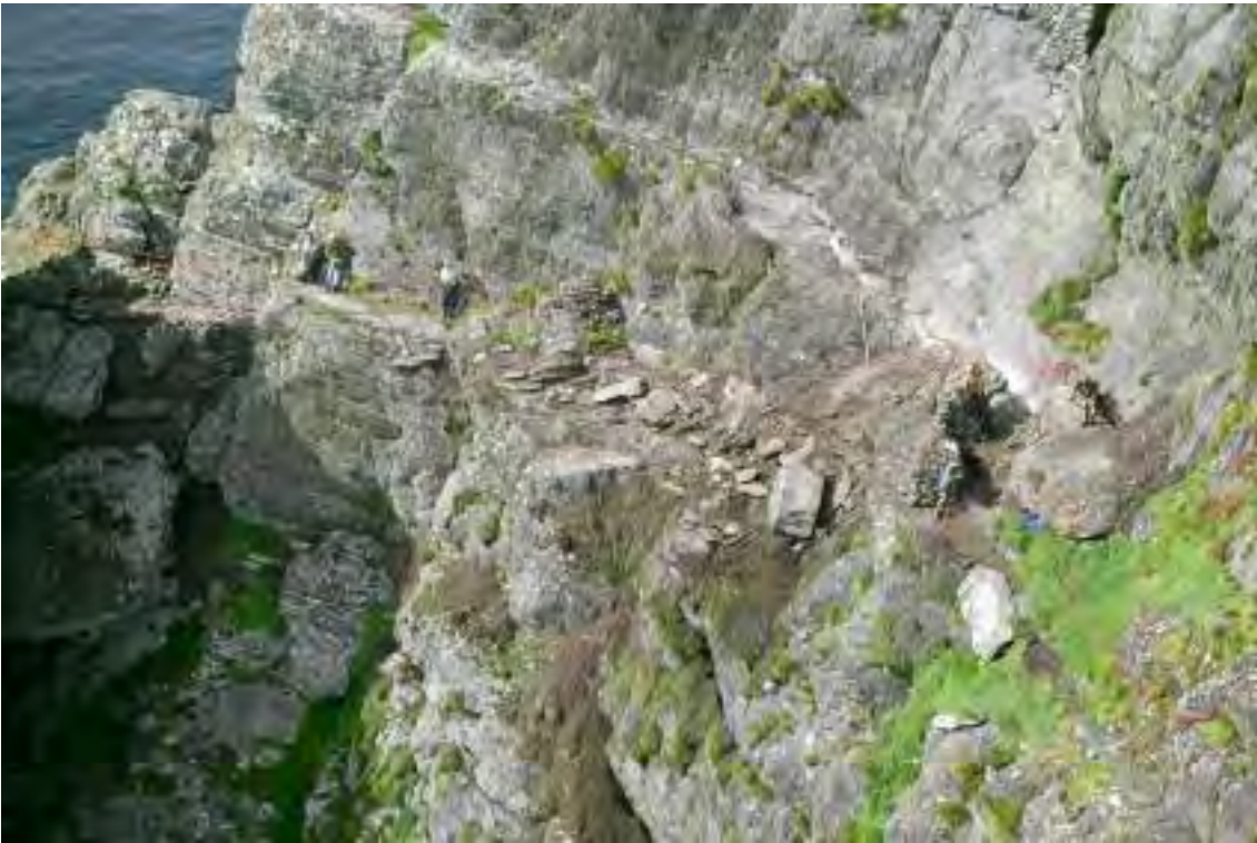
Ill. 2.245— Aerial view of the southern traverse of the north-west passage during excavation (Con Brogan, DAHG).
