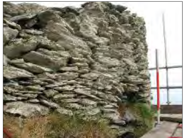
Ill. 2.502—Large hole in the base of the wall at the south-western corner of the terrace (A.R. Hayden).
