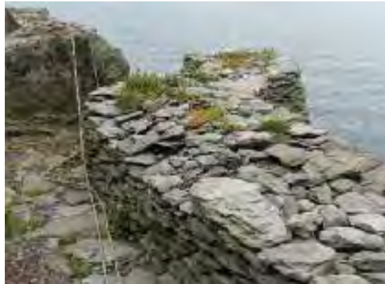
[Left] Ill. 2.461—The external face of the wall at the southern end of the upper traverse after excavation (A.R. Hayden).
