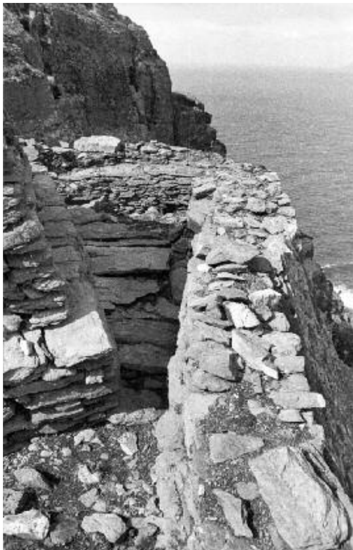
Ill. 2.22—The flagstones projecting from beneath the east wall of the small oratory (A. Lynch).
