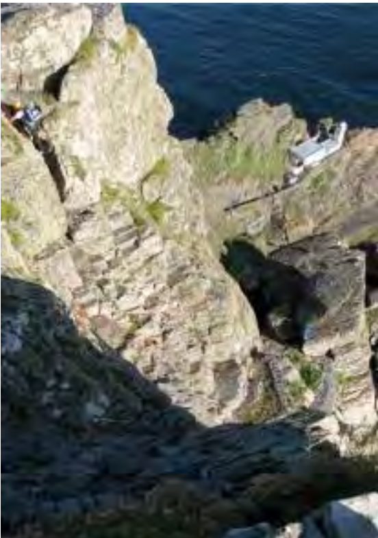
III. 2.356—Looking down from the outer terrace on the climb from the upper platform (bottom right) to the 'garden' terrace (upper left). The heavily quarried surface of the slope behind is clearly visible (A.R. Hayden).
