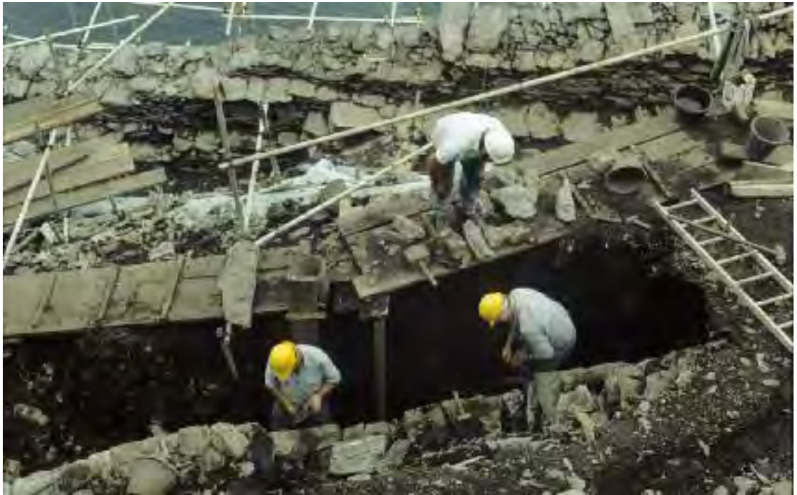
Ill. 2.124— Constructing the revetment wall in Cutting 4 (E. Bourke).
