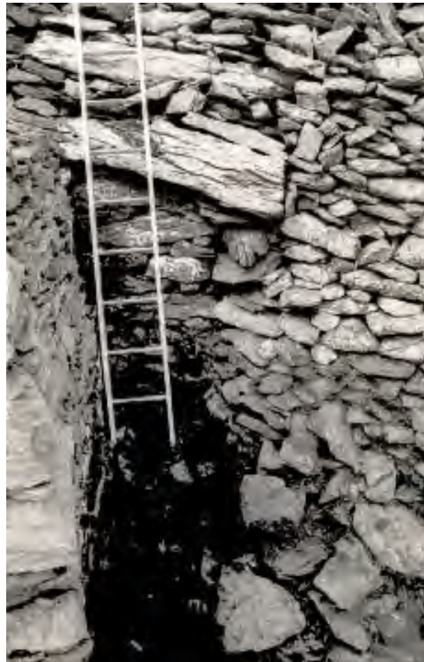
Ill. 2.63—Exterior of lintel, showing wall pushing outwards (E. Bourke).
