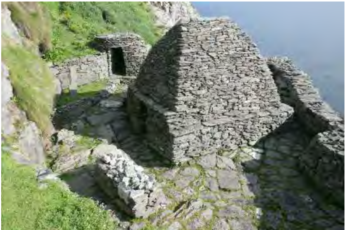
Ill. 1.6—The small oratory terrace viewed from south (Con Brogan, DAHG).
