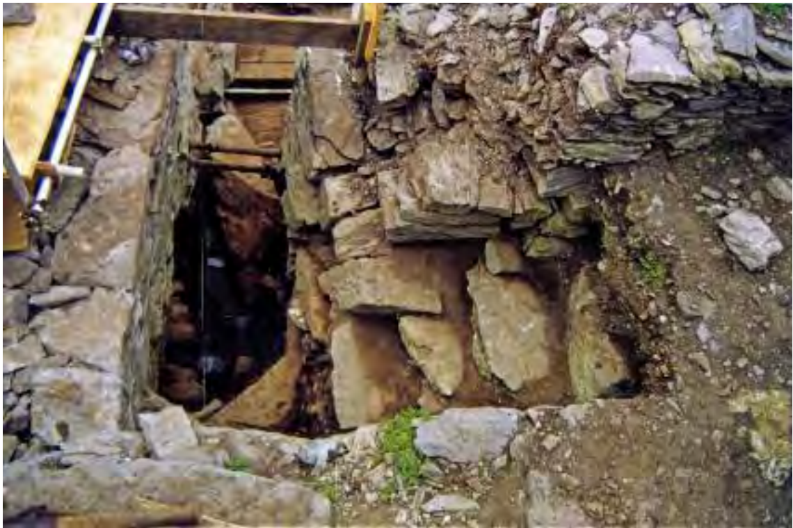
III. 2.42—Upper level of steps, south entrance I, from north (E. Bourke).
