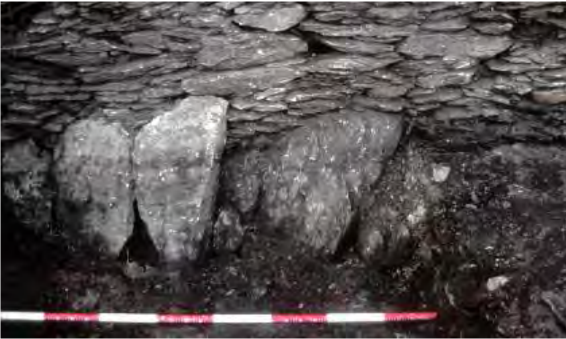
Ill. 2.144—Wall showing orthostatic base (E. Bourke).
