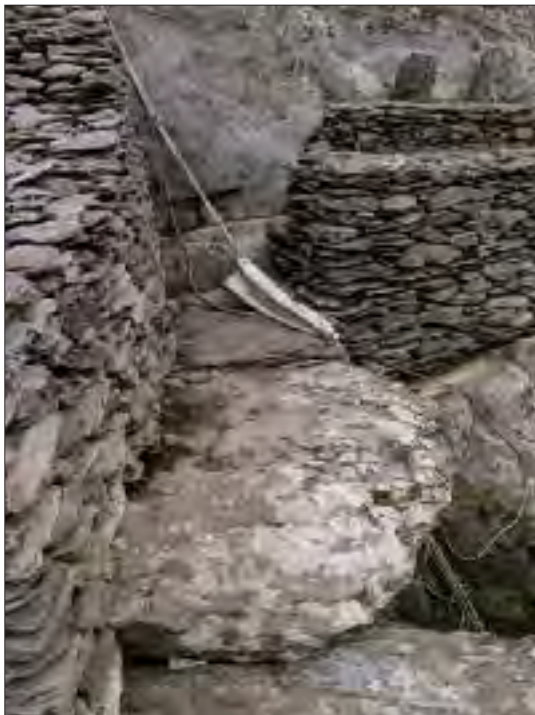
Ills 2.404 and 2.405—The upper bridging stone replaced, showing that there was ample room for access around the east end of the oratory, even though the stone was replaced further to the west than its original position (A.R. Hayden).
