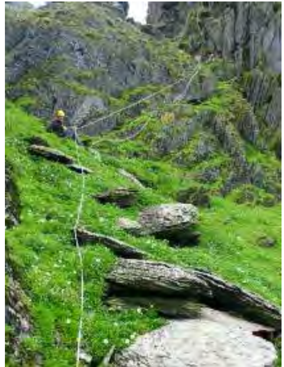
[Right] Ill. 2.567—Slipped stair treads in gully (6), with terrace (7) above (A.R. Hayden).
