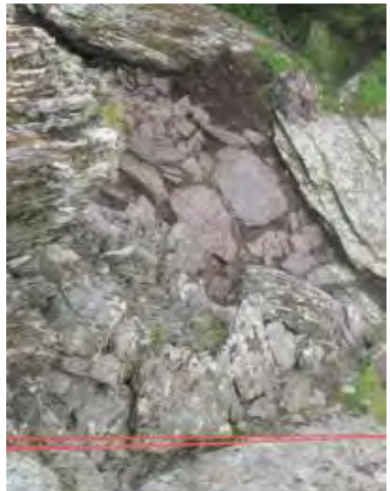
[Right] Ill. 2.262—The gaps in the base of the wall were built up with stone to support the wall as the excavations progressed (A.R. Hayden).
