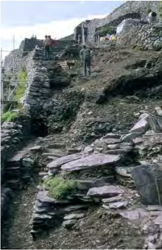
Ill. 2.89— Collapse over Cell G (E. Bourke).
