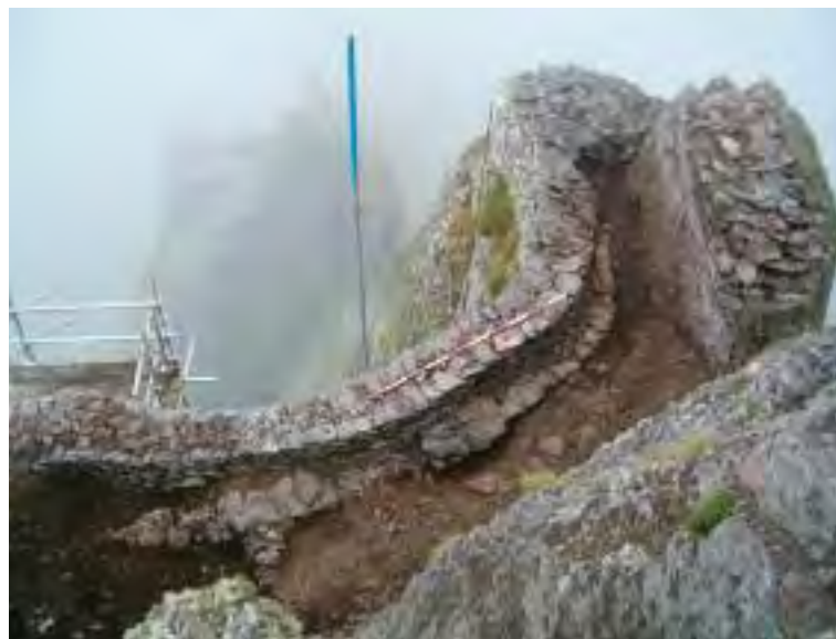
Ill. 2.374—The reinforcing wall viewed from above (A.R. Hayden).
