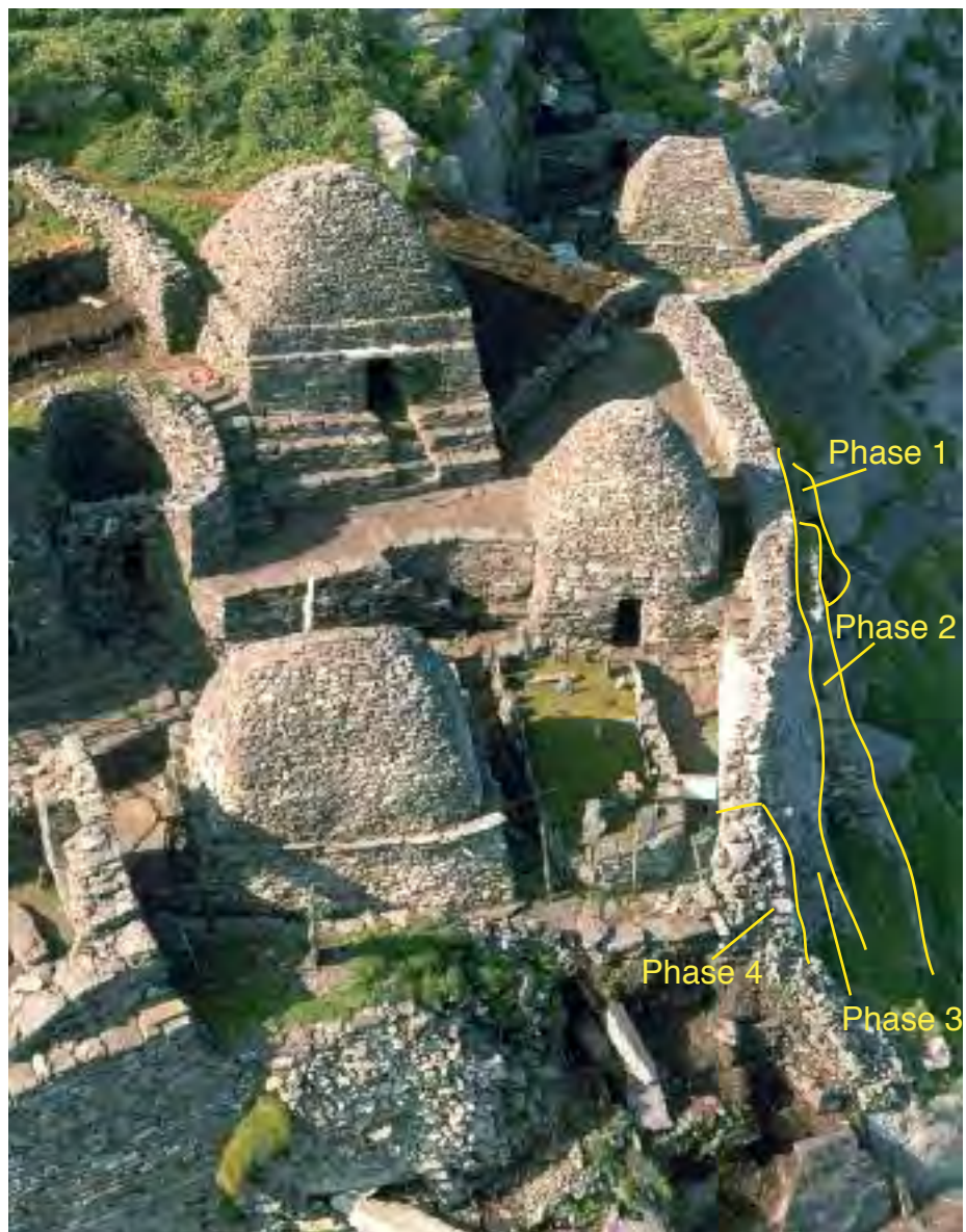
Ill. 2.61—Phases of development in east wall, inner enclosure, from south (Con Brogan, DAHG).
