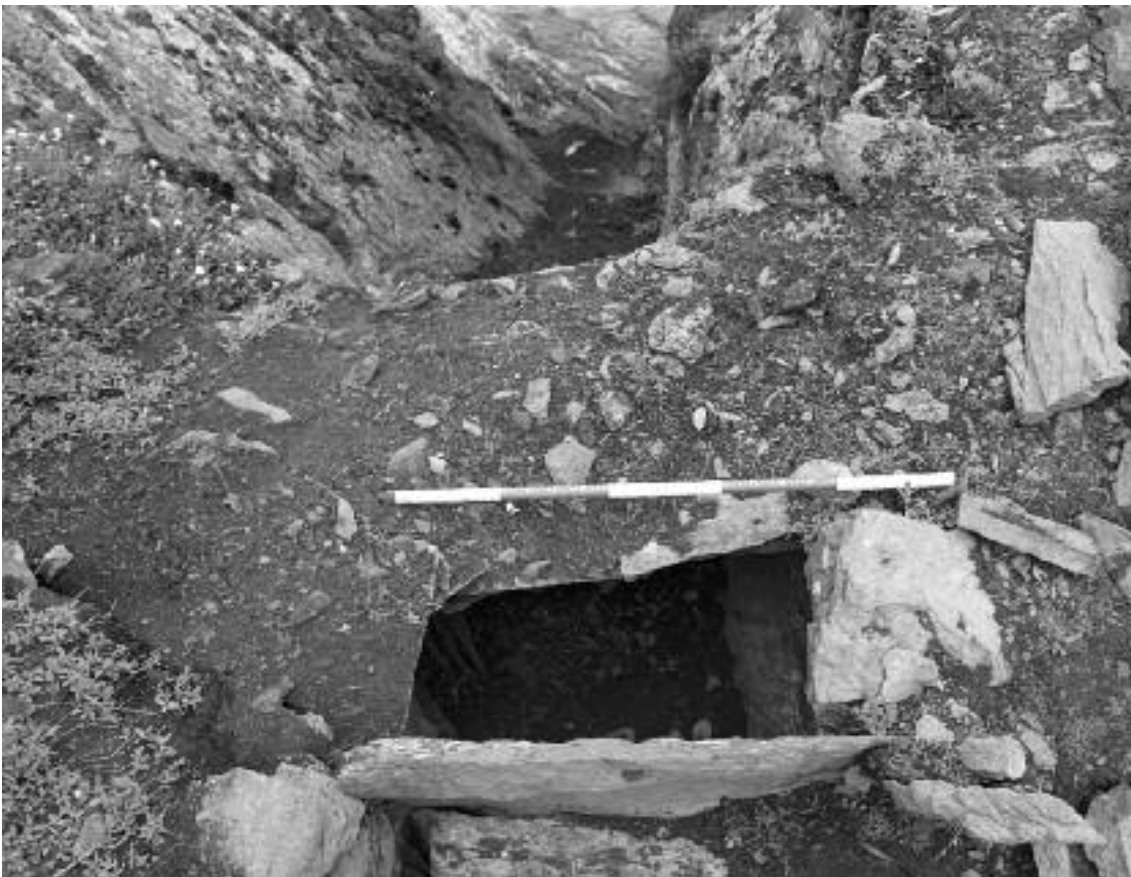
Ill. 2.20—The east wall of the 'latrine' and opening to gully below, after removal of campion growth (A. Lynch).
