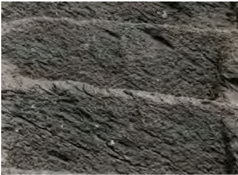
III. 2.549— Detail of tooling on latest lighthouse steps (A.R. Hayden).
