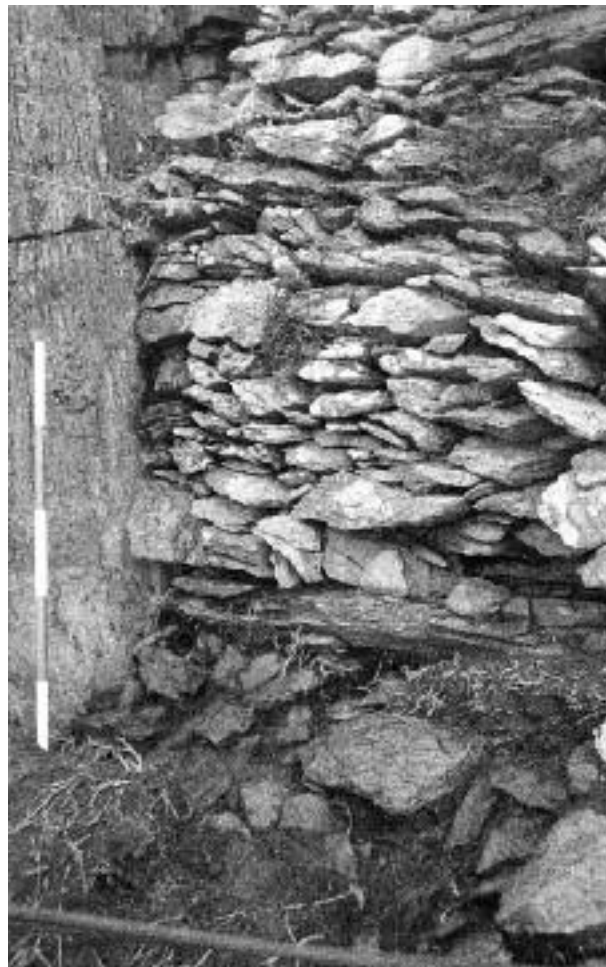
III. 2.8—Rubble foundations of the small oratory terrace retaining wall (A. Lynch).
