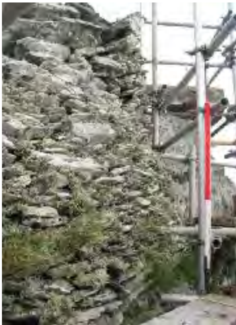
Ill. 2.502—Large hole in the base of the wall at the south-western corner of the terrace (A.R. Hayden).
