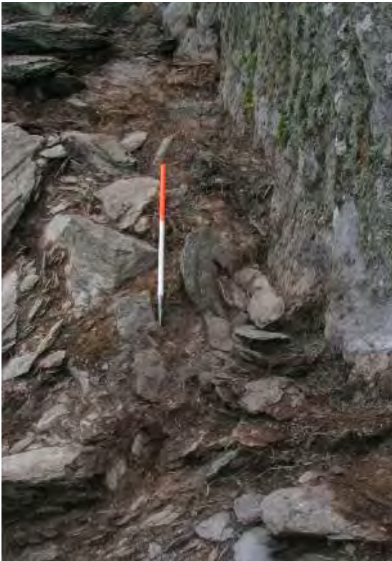
III. 2.224—The drip gully on the inner side of the stairway (A.R. Hayden).
