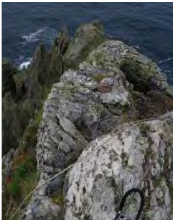
[Left] Ill. 2.470—The final part of the climb down originally lay partly on the wall top, which no longer survives (A.R. Hayden).
