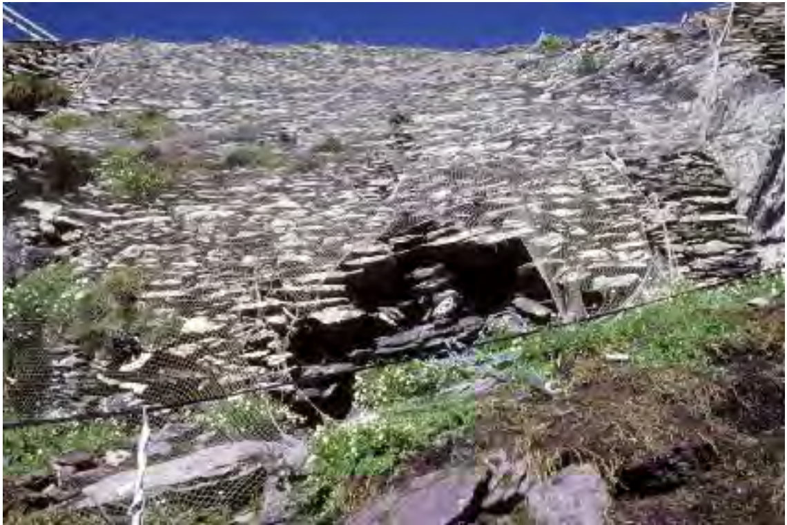
Ill. 2.3— Unravelling at base of small oratory terrace retaining wall, before works (A. Lynch).
