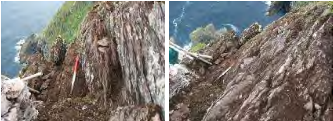
Ills 2.489 and 2.490—Looking down on the north-eastern corner of the terrace during excavation. The few surviving stones of the northern wall lie on the right (southern) side of the bedrock rib at the cliff edge. No trace of an eastern wall survived. The conserved lower end of the western wall is visible at the left (A.R. Hayden).
