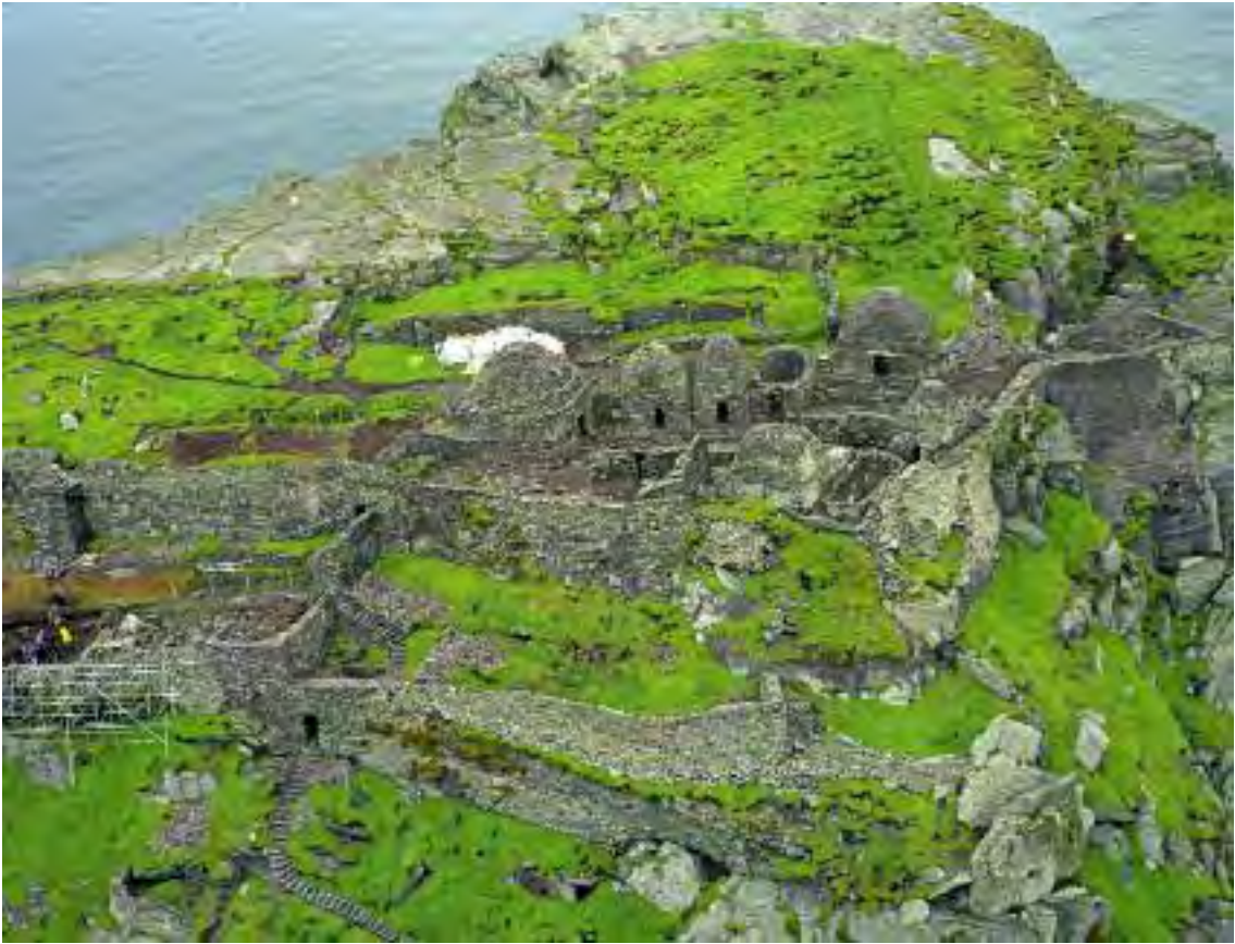
III. 2.121— Nineteenth- century wall F630 and its position relative to the early medieval wall F640 (Con Brogan, DAHG).
