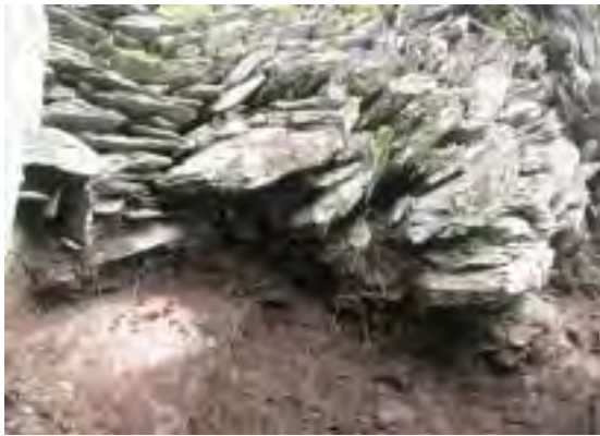
[Left] Ill. 2.261—The gaps at the base of the wall of the fourth section (A.R. Hayden).
