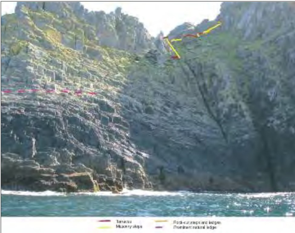
III. 2.556— Photograph taken from sea level to the east, showing the features of the lowest explored part of the new route to the monastery (A.R. Hayden).
