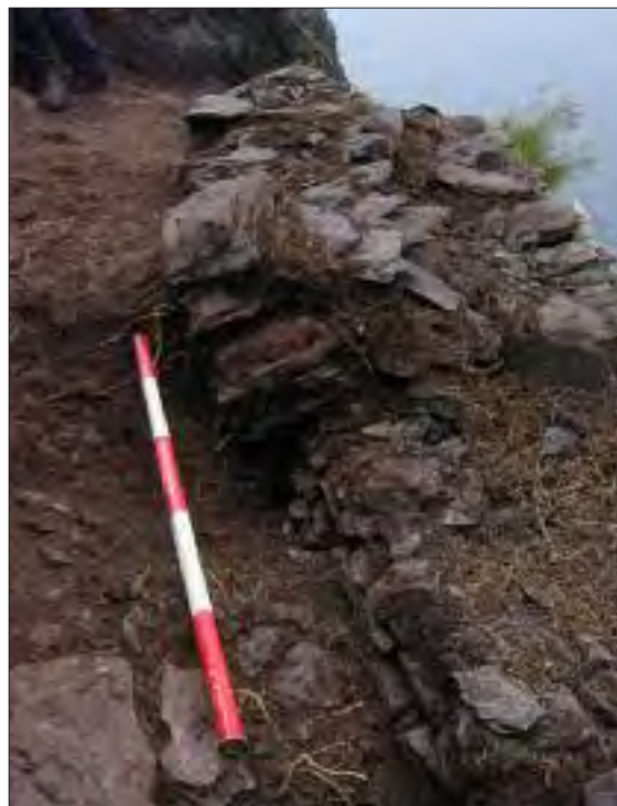
Ills 2.452 and 2.453—The collapsed secondary facing of the inner face of the wall of the upper traverse (A.R. Hayden).
