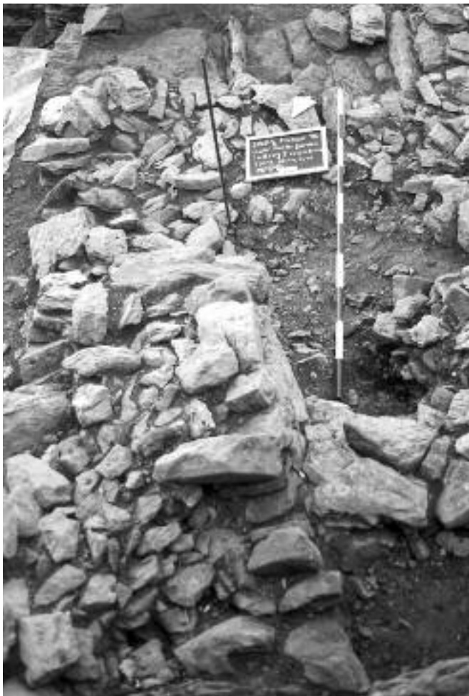
Ill. 2.125— North-south wall (F637) west of Cell G during excavation (A. Halmschlag).
