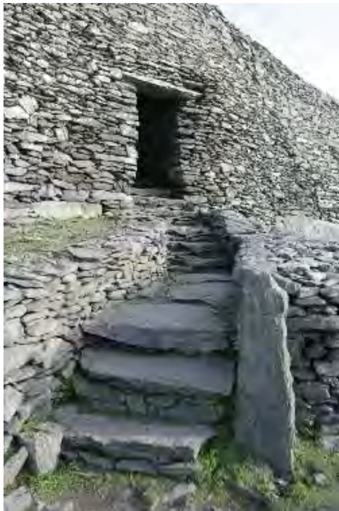
Ill. 2.57—South entrance 2 (inner enclosure), steps leading from outer enclosure (Con Brogan, DAHG).
