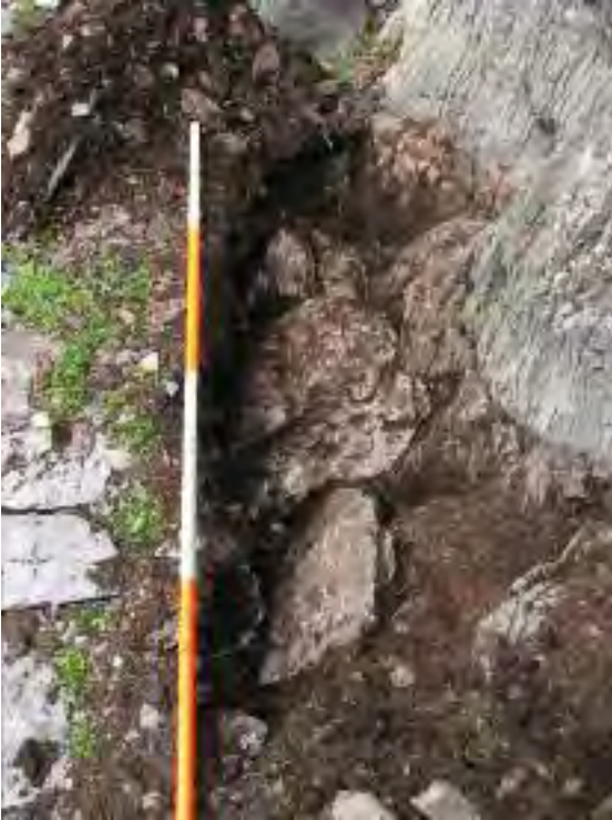
III. 2.354—Distorted paving at the back of the upper platform (A.R. Hayden).
