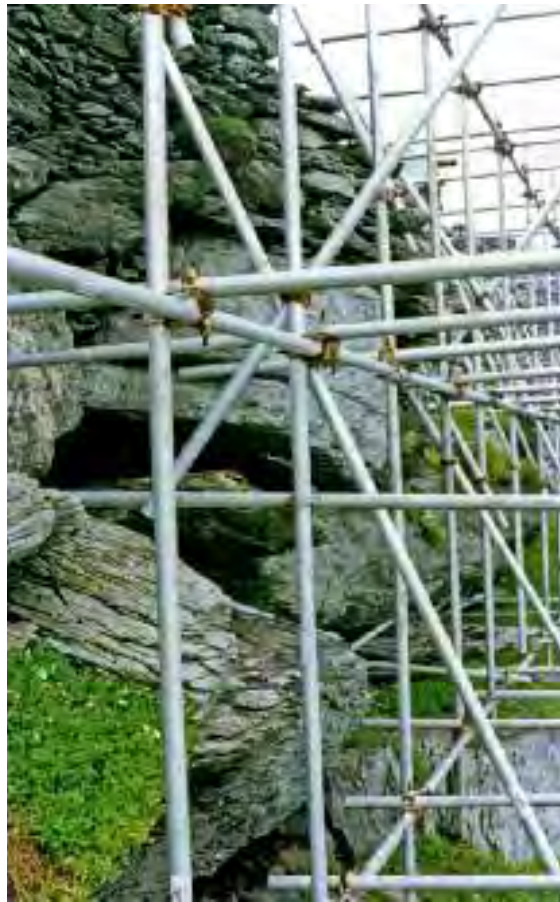
Ill. 2.138—Boulder layer at exterior face of wall (C. Cotter).
