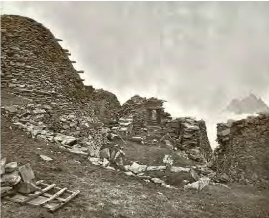
Ill. 2.126— Photograph from Dunraven 1875–7, showing collapse of wall of inner enclosure.
