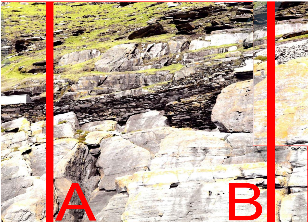
Retaining wall A-B. This section was completed in 2014.
