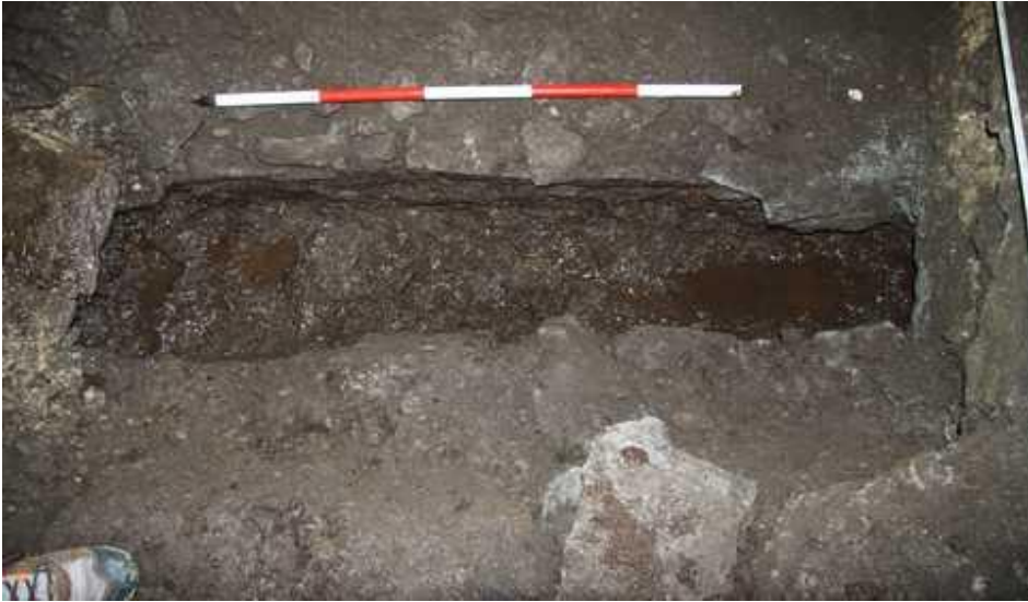
Drain after opening up.
