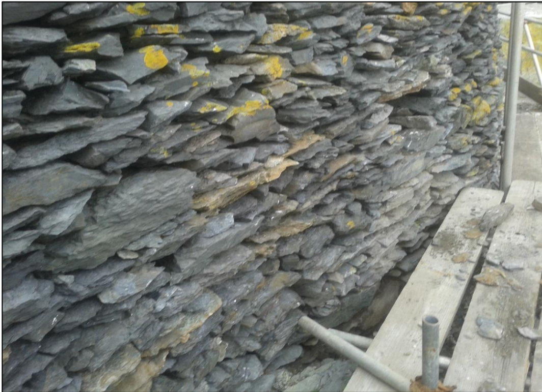
Figure 3. Typical section of masonry seawall undergoing wall tightening works
