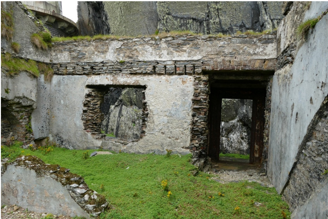
Figure 4 – Existing debris in Upper Lighthouse
