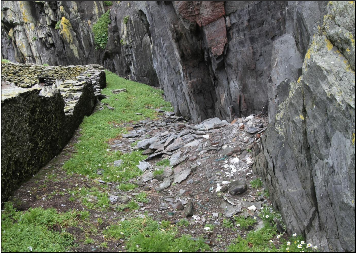
Figure 4. Typical road surface along Upper Lighthouse Road prior to removal of surface vegetation
