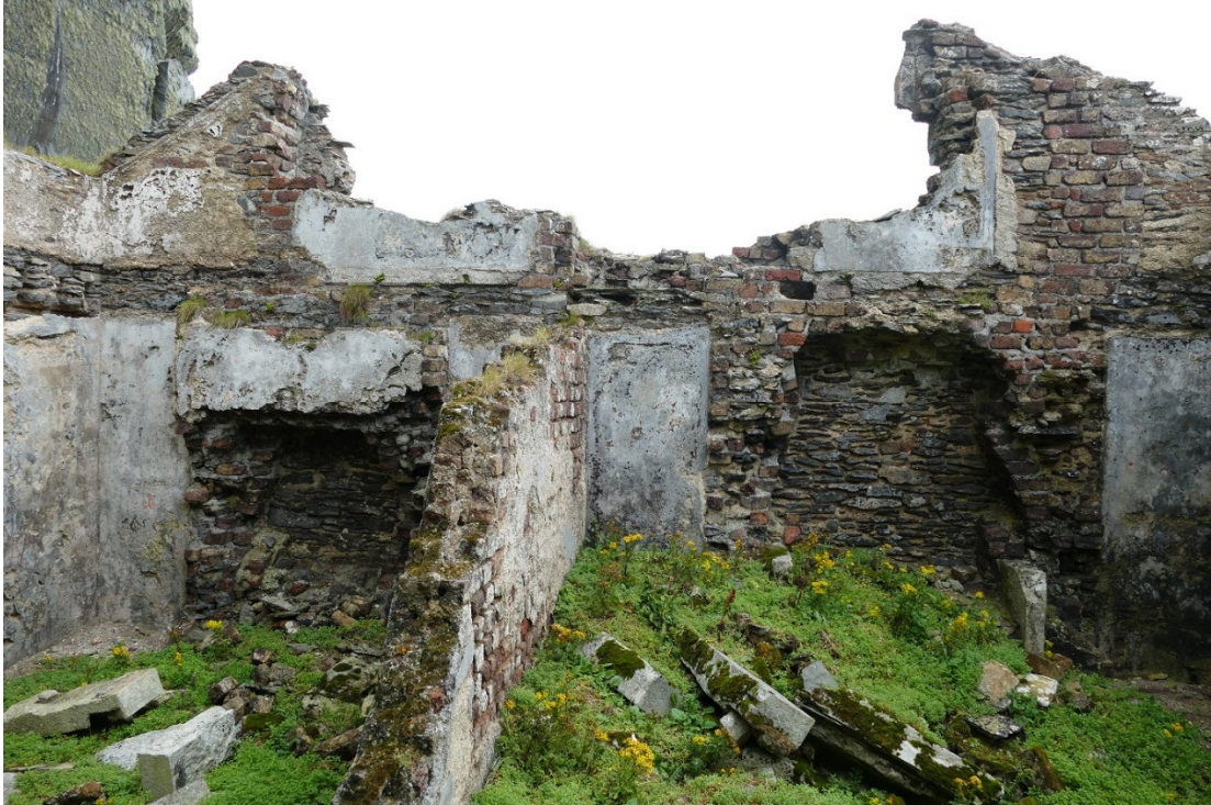
Figure 7 - Existing debris in Upper Lighthouse
