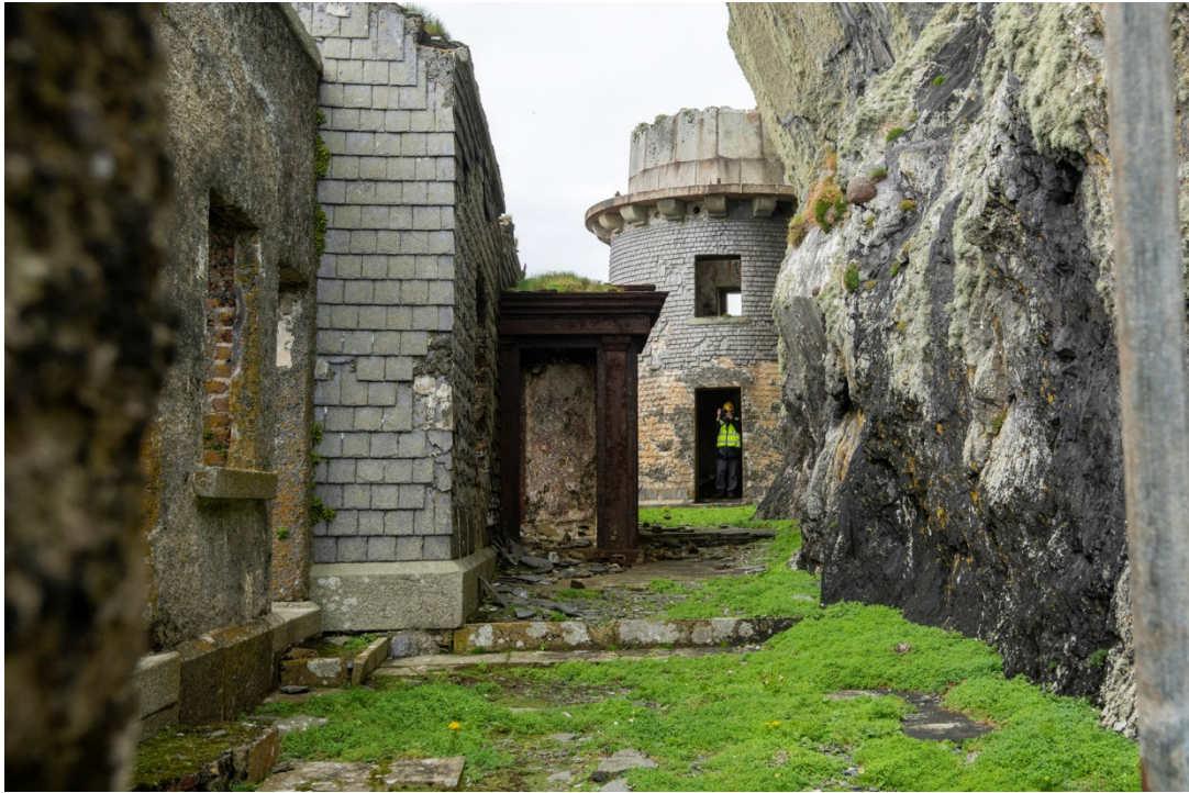
Figure 3 - General view of the Upper Lighthouse building and tower
