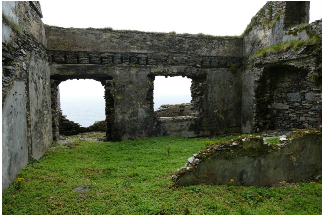
Figure 6 - Existing debris in Upper Lighthouse
