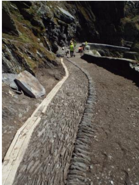
Pl. 26B Upper Lighthouse road, post excavation, showing original road surface, drains and an electrical conduit inserted in the early 20 th century
