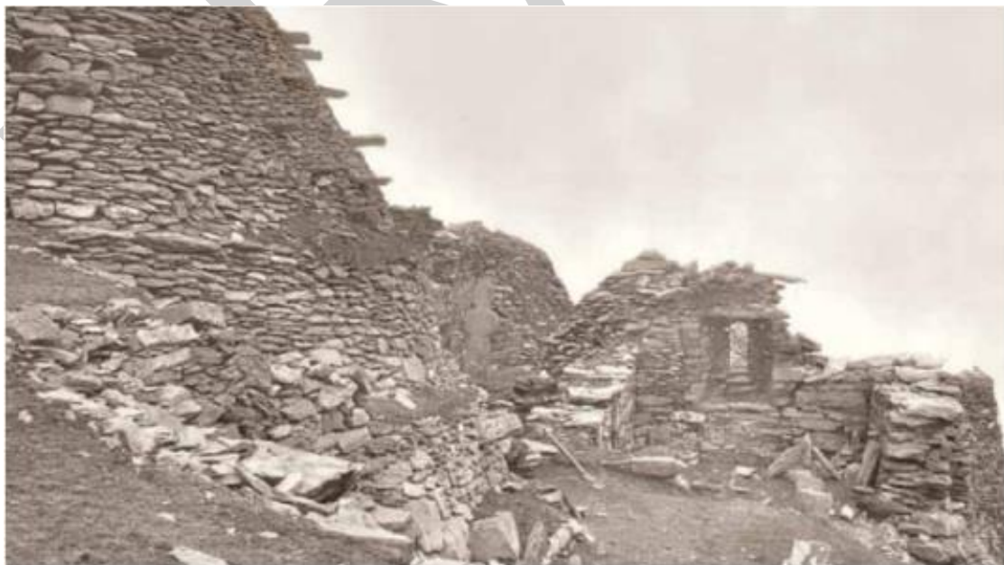
Pl. 6 View of St Michael's Church, showing the collapsed retaining wall on the south side.
