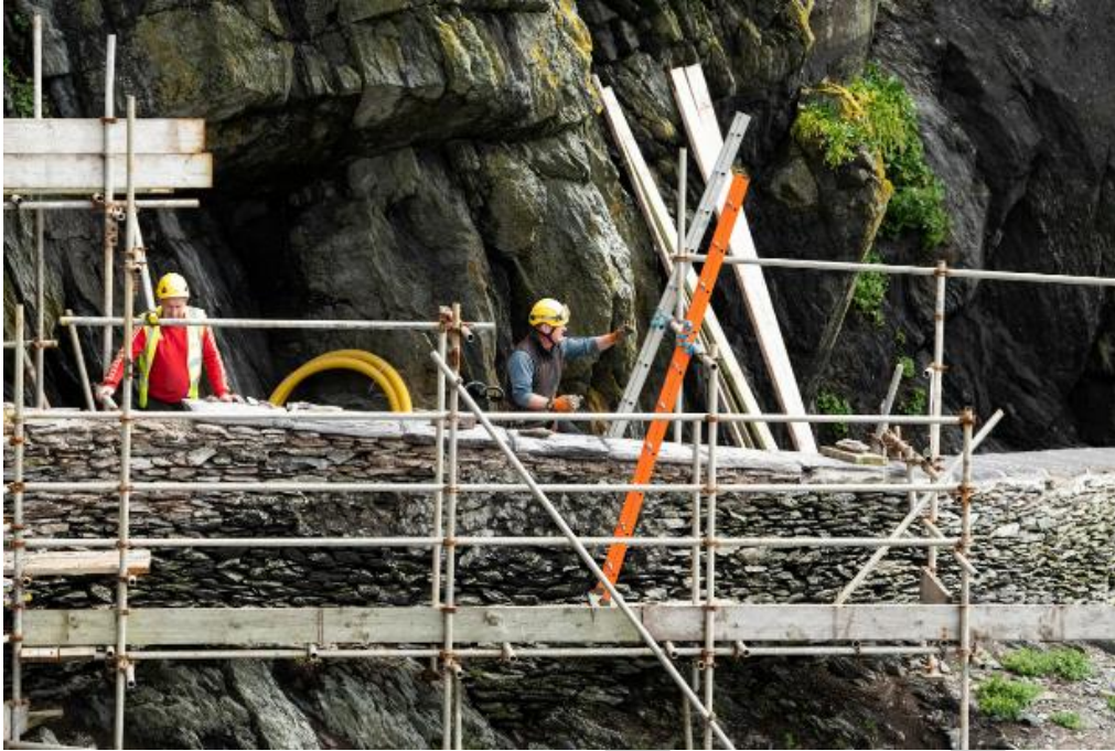
Pl. 17 Re-laying Valentia Slate capstones on the sea wall north east of the Lower Lighthouse Compound
