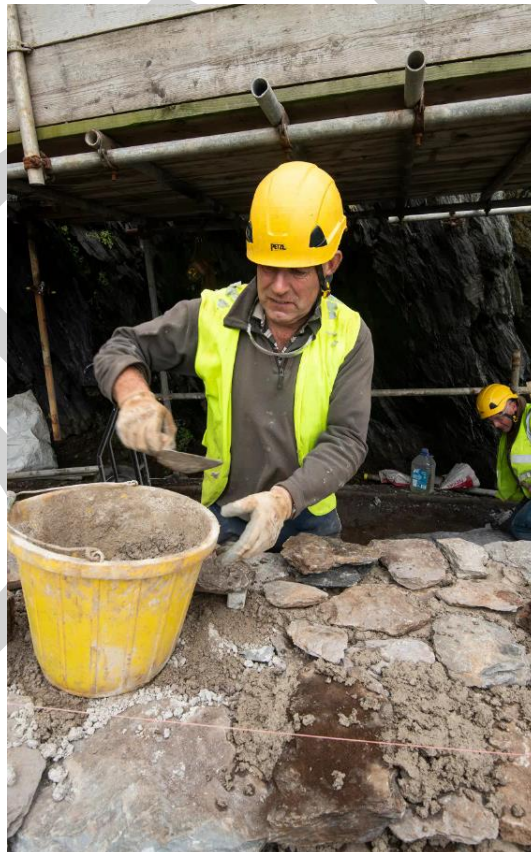
Pl. 18 OPW mason laying base for new capstones on the sea wall, Upper Lighthouse road.
