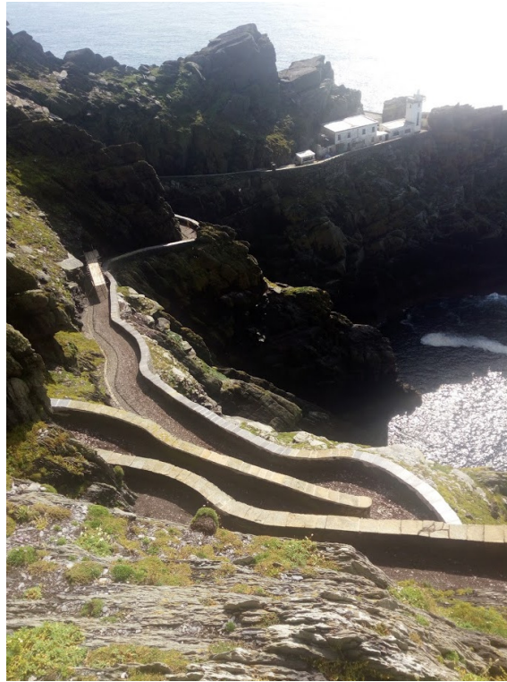
Fig. 6. – View of Upper Lighthouse Road from Upper Lighthouse Gate. Debris removed, wall tops repaired.
