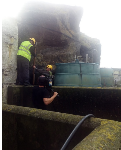
Fig. 15.- Dismantling of fuel storage tanks at Lower Lighthouse, September 2020.
