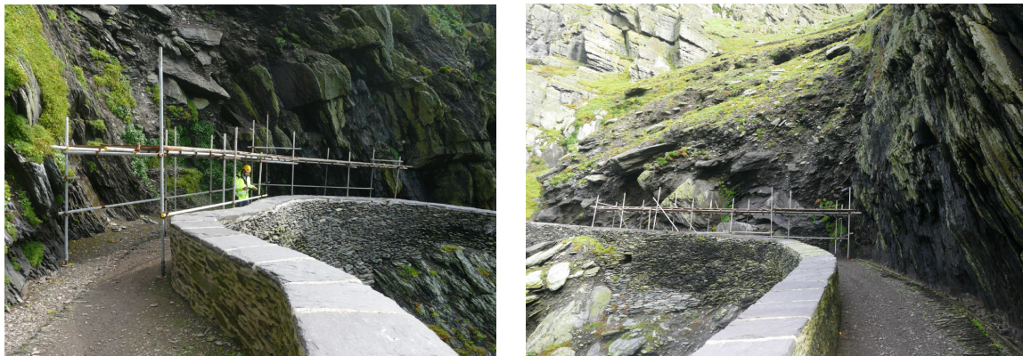
Fig.29. – Temporary crash deck location B & C on the Upper Lighthouse Road.
