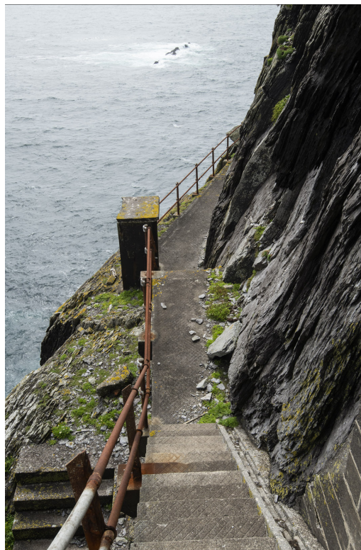
Fig. 10. – Existing fog signalling station walkway.
