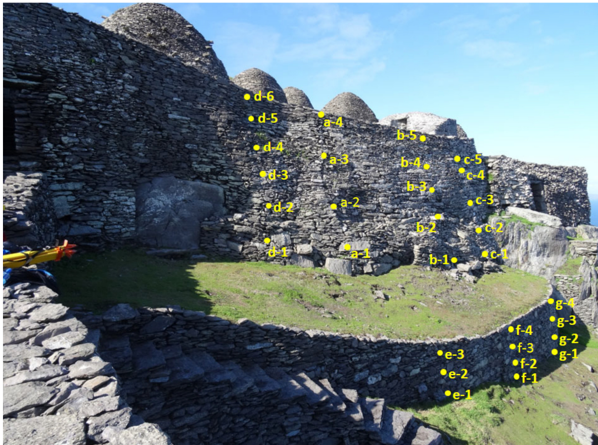
Fig. 13. - Discovery Programmed marker point locations at monastery retaining wall.
