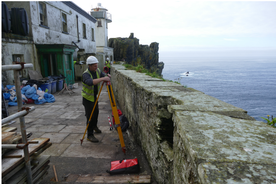
Fig. 12. – Survey works being conducted by PCA on Skellig Michael
