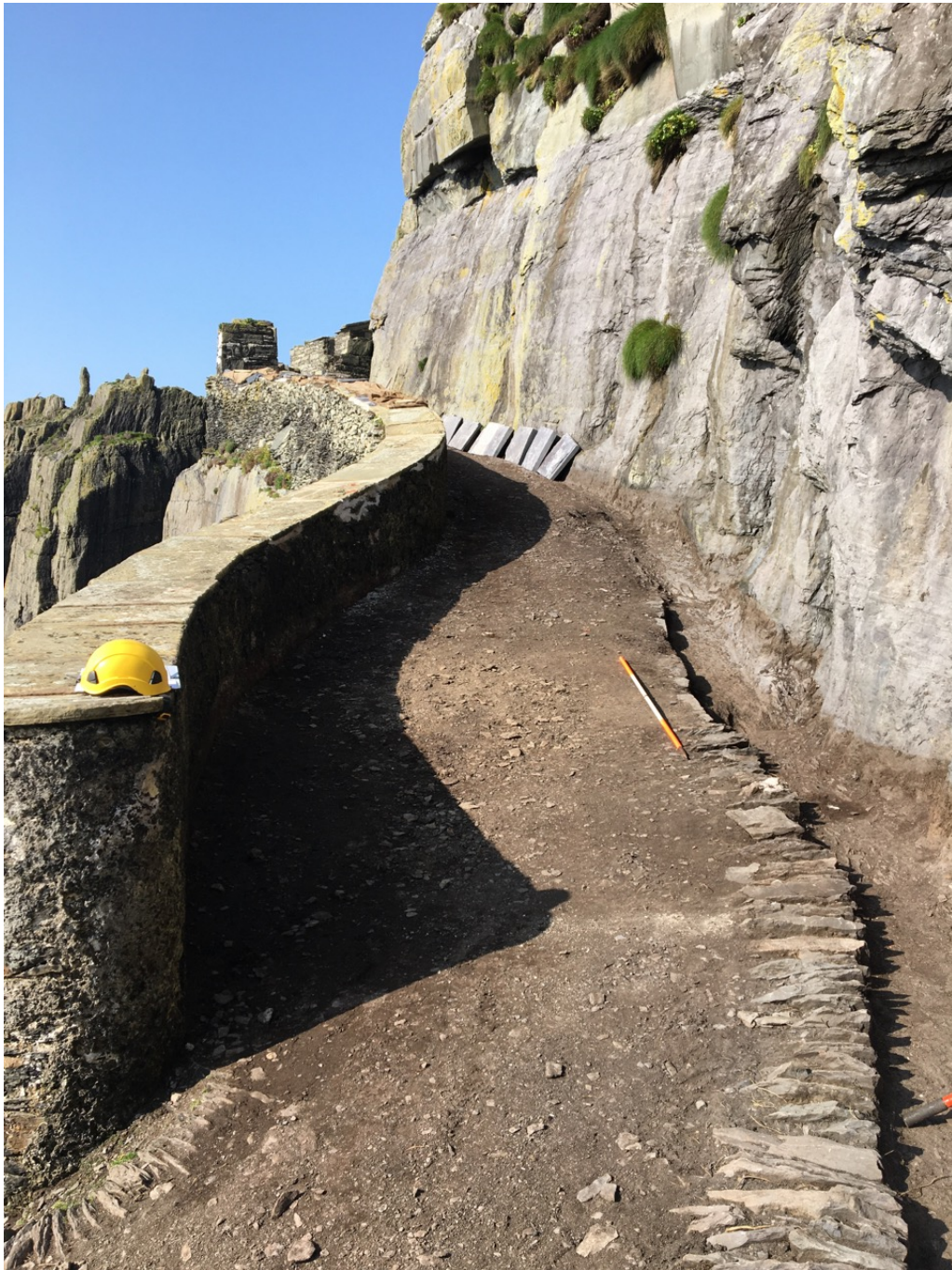
Photograph 22, section E4 looking west. Intact road edging and lateral drain, with disturbed shore / drain open by ranging rod (see photograph 23).
