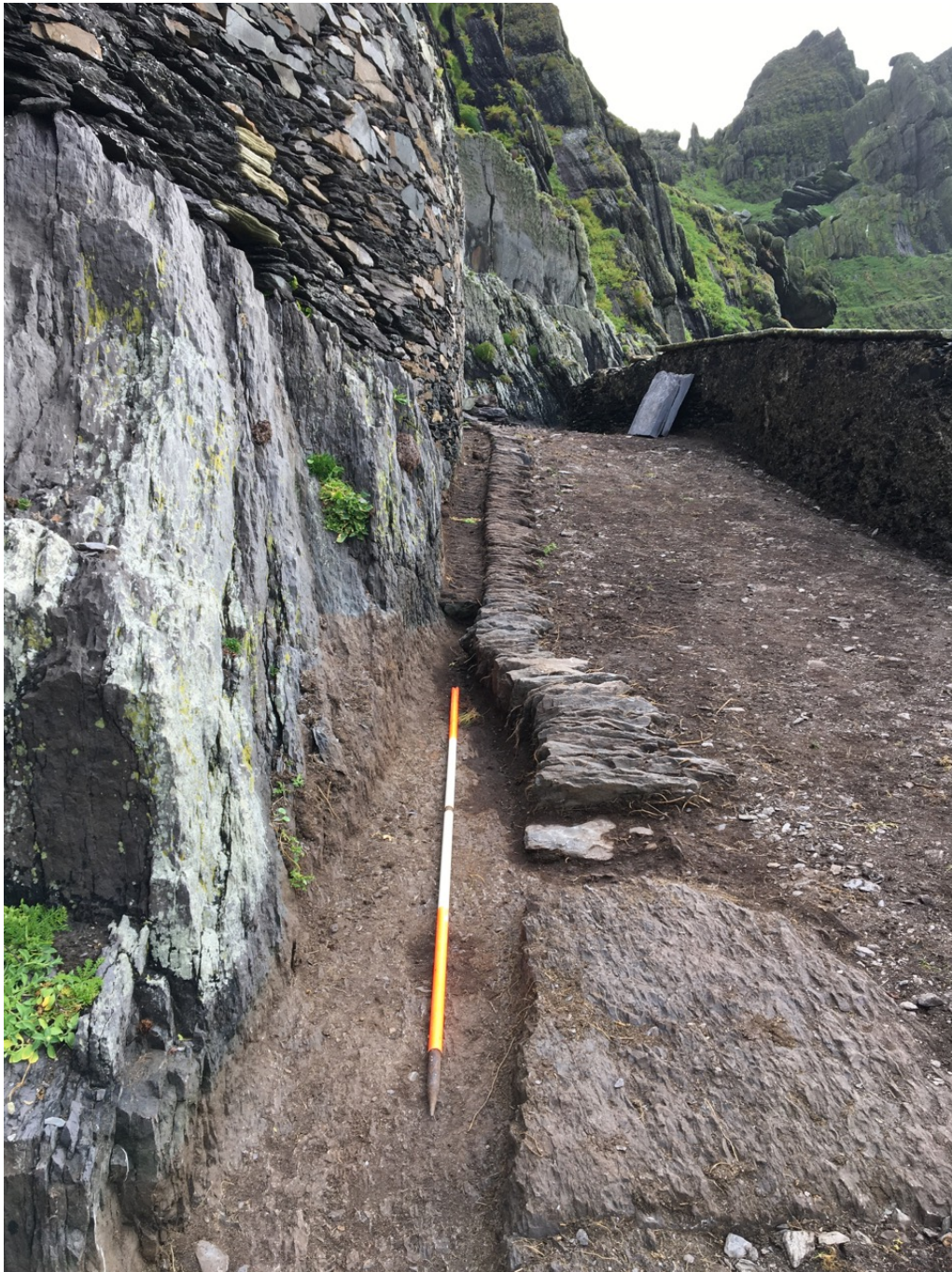
Photograph 20, section E3 looking east. Rock cut lateral drain in foreground, original road edging and intact set stone base of lateral drain behind.
