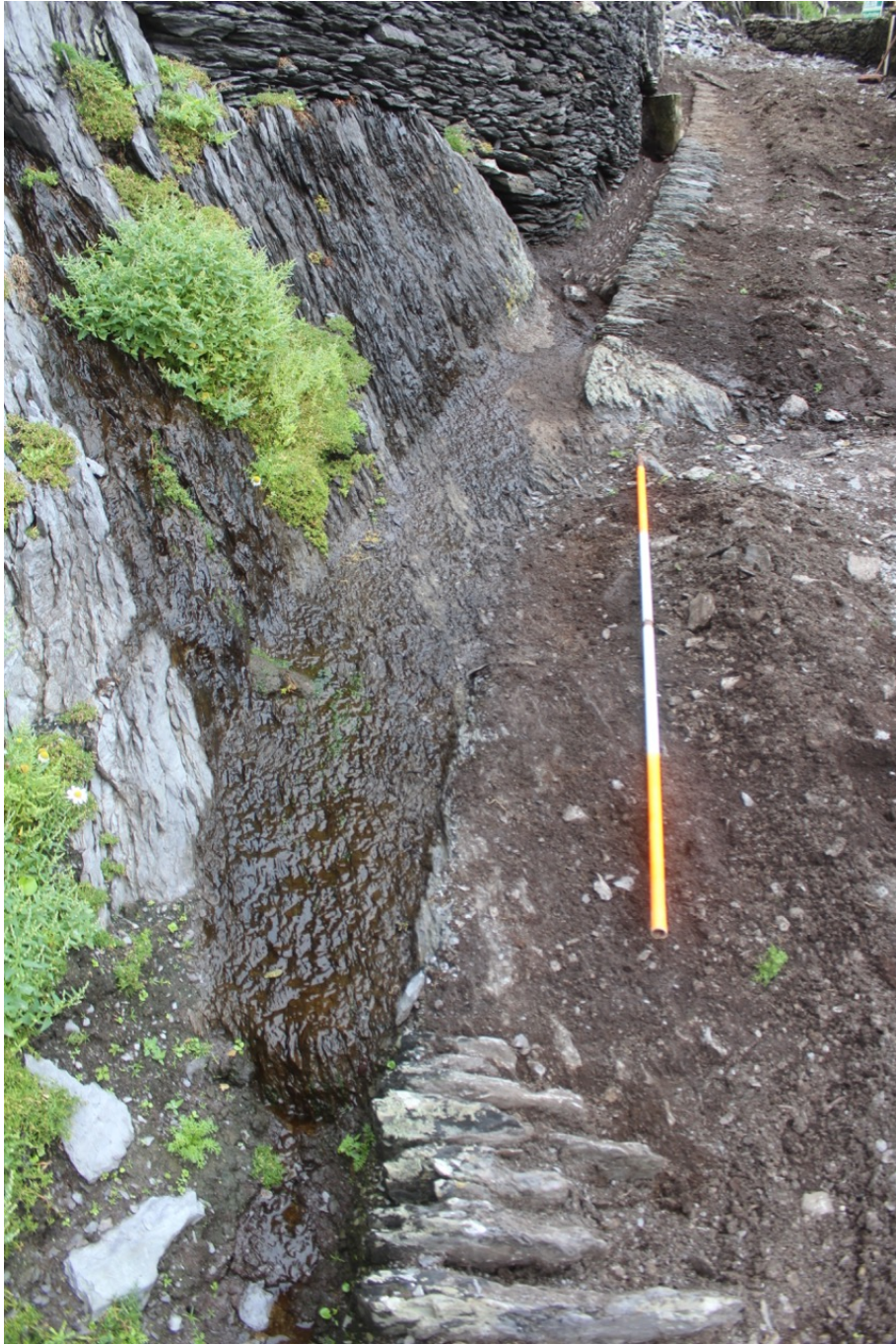
Photograph 2. Section E1 looking east. Rock cut lateral drain, with replaced road edging beyond ranging rod.
