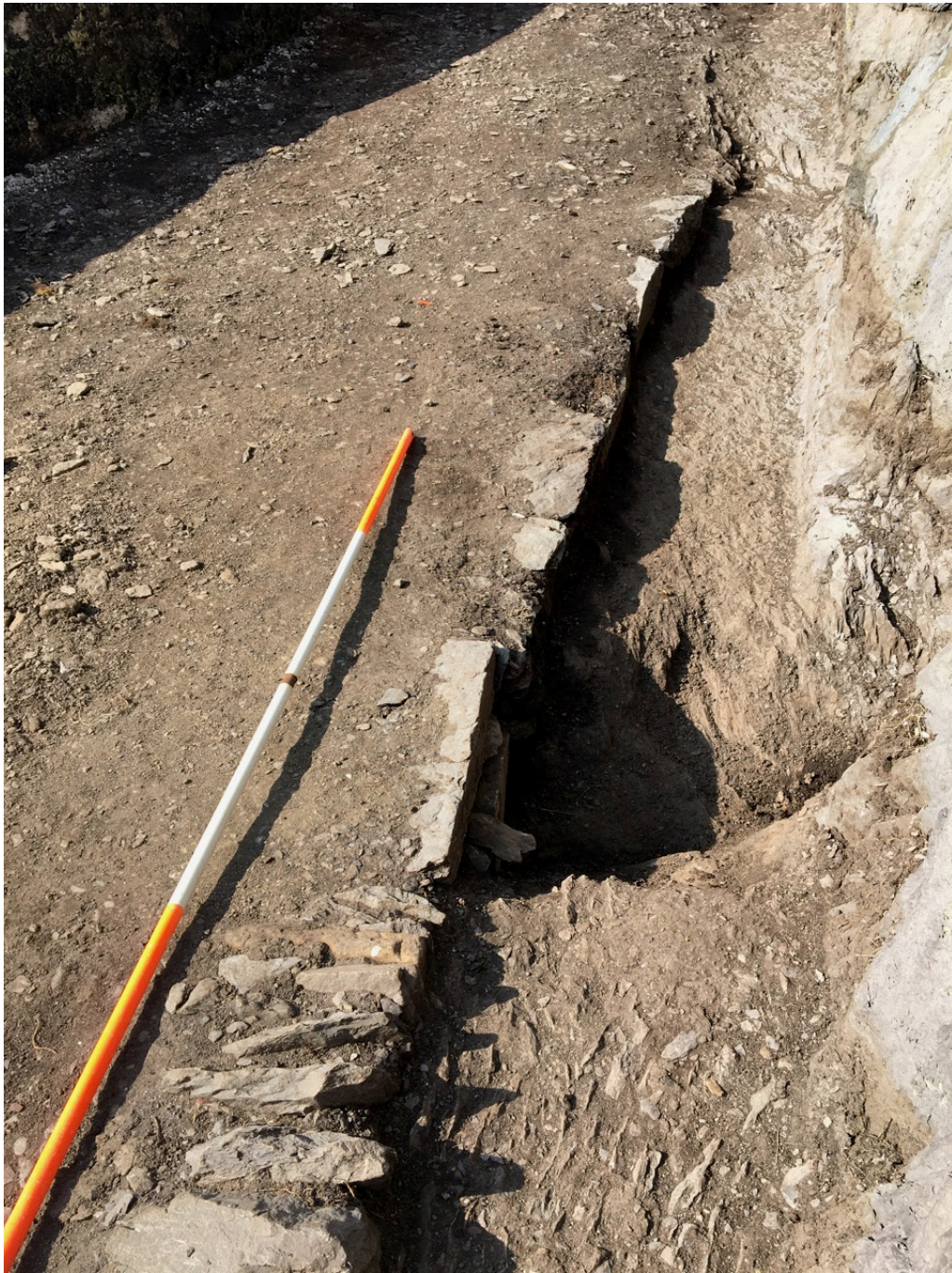
Photograph 23, section E4 looking west. Subsurface drain opening, possibly originally holding stone shore and intact set stone base of lateral drain, rock cut base in background. Note possibly rebuilt road edging.
