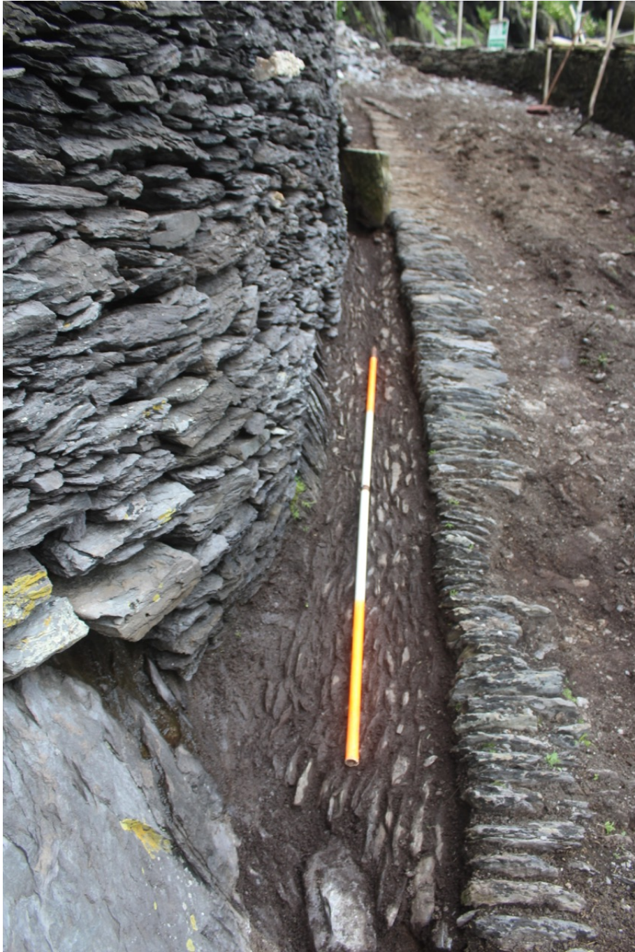
Photograph 3, section E1 looking east. Replaced road edging and intact lateral drain base. Surviving road surface below original level.
