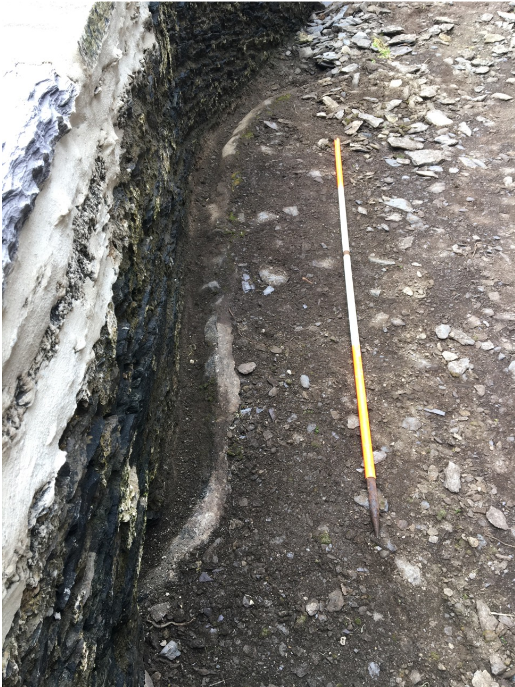
Photograph 13, section E2 looking west. Surface drain inside parapet wall.
