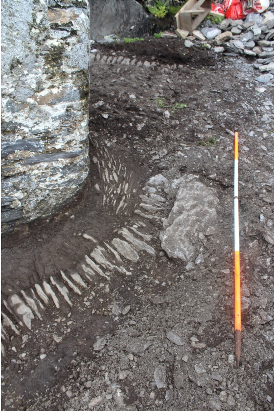
Photograph 6, section E1 looking north. End of parapet wall with lateral drain curving around it. Note change in alignment of stones in lateral drain.
