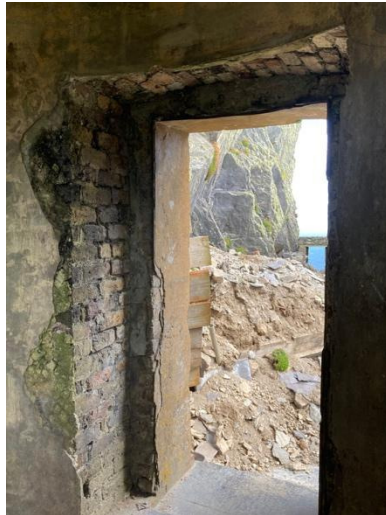
Fig.89. Interior of lighthouse doorway.
