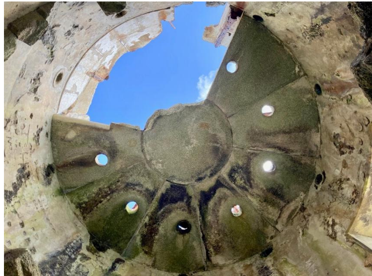
Fig.98. Second floor from below.
