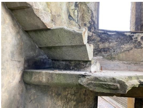
Fig.92. Detail of ope in first floor & stairs up to second floor.
