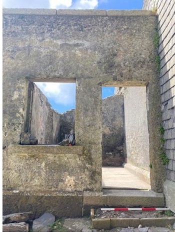
Fig.76. Outhouse (4) front wall.
