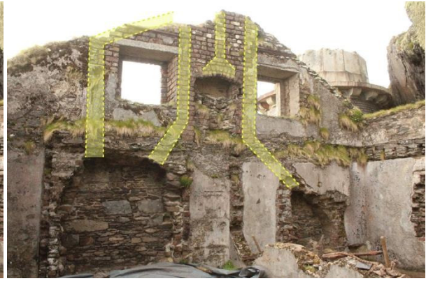
Fig.43. House (1), interior west gable, with lines of flues from fireplaces shown.
