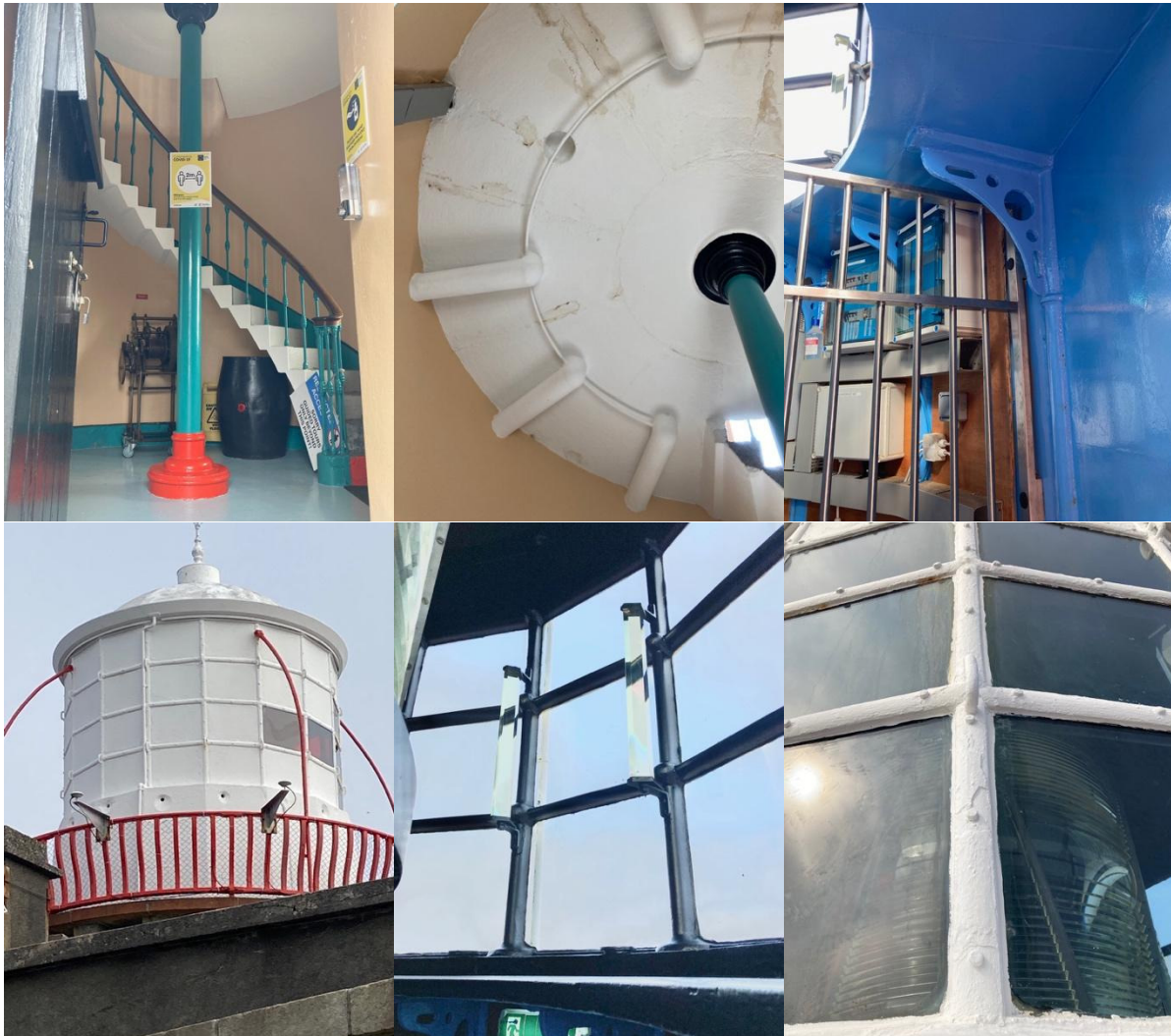
Fig.175. Details of the stairs, underside of the top floor & the lantern of the Valentia Island lighthouse. Virtually identical to the lighthouses on Skellig, apart from the (possibly later) central column supporting the floors. Other details of the station, such as the use of the same yellow sandstone paving and granite wall caps closely parallel those of the Skellig stations.
