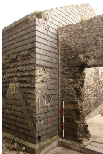
Fig.13. House (1), NW corner.
