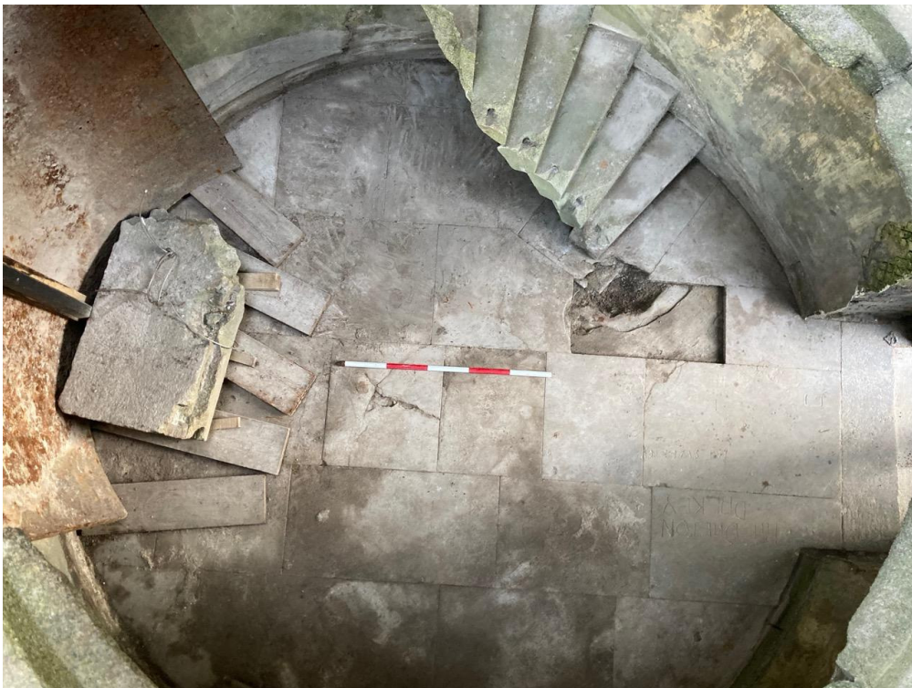
Fig.91. Ground floor of lighthouse after excavation. Back of lantern and fragment of mantlet wall stored at left.
