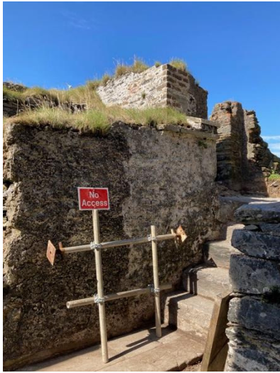
Fig.115. Brick masonry added to Coal Shed, part of Toilet (17).
