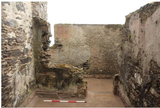
Fig.69. Rear wall & doorway of Outhouse (3).
