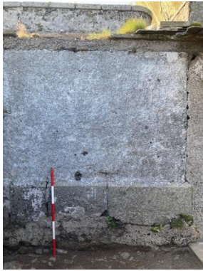
Fig.123. Plinth at base of east wall of Shed (21).
