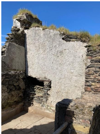
Fig.111. North wall of Teacher's House (16).
