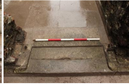
Fig.68. Outhouse(3), cill of front door.
