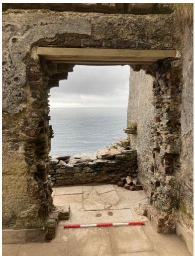
Fig.24. house (2), back door.
