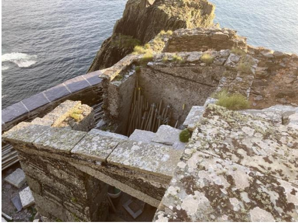
Fig. 138. Shed (25,) roof level, with shed (26) behind.
