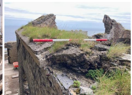
Fig.48. House (2), granite cornice on front wall.
