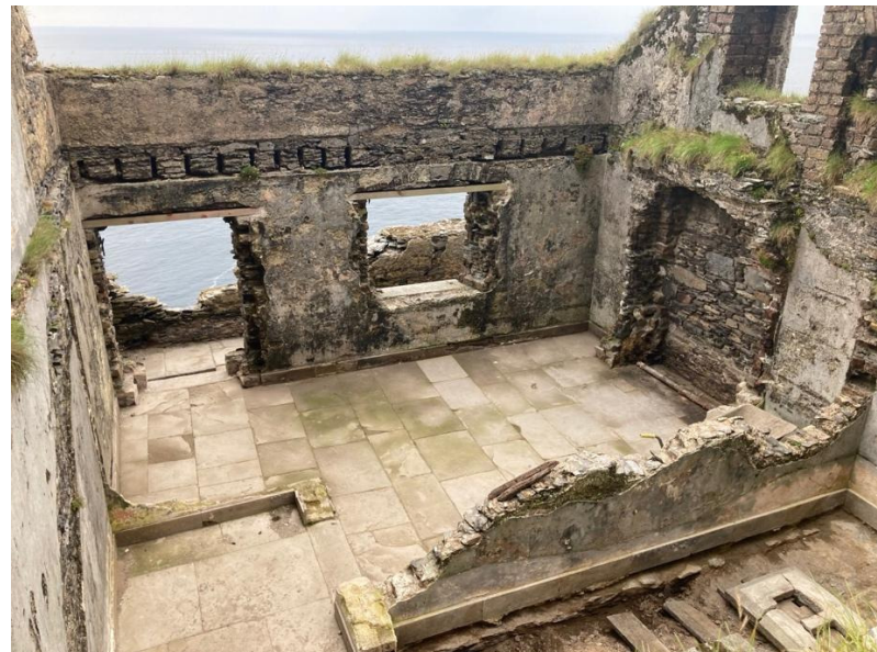
Fig.38. House (1), back kitchen.
