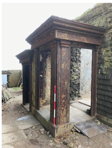
Fig.16. Porches, House (1) at front.
