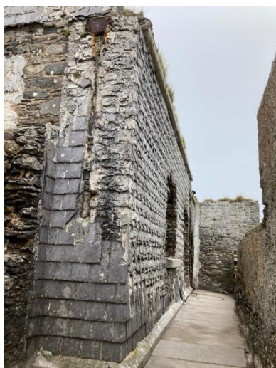
Fig.14. House (1), SW corner.
