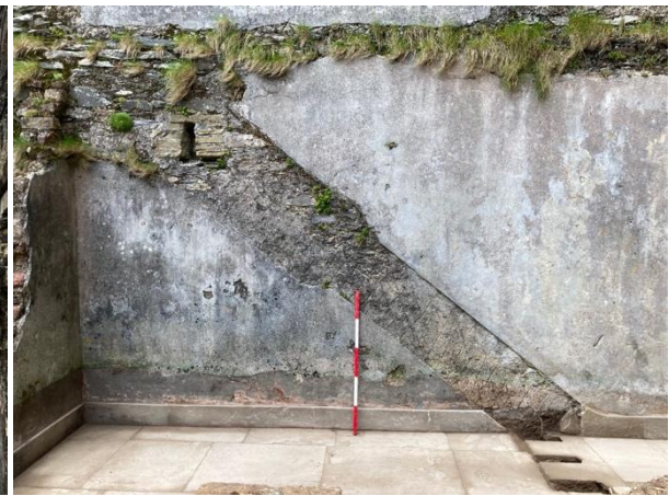
Fig.31. House (2), ghost of stairs on west gable.
