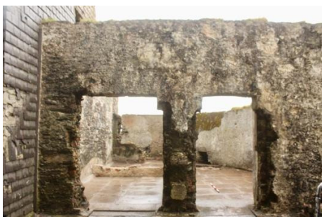
Fig.54. House (1), front wall of yard (10) & outhouse (3), outhouse doorway on left.
