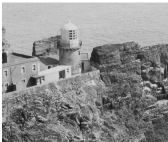
Fig. 168. The Lower Station before the 1960s after the original roof of the houses was removed & the corridor was added to the tower.
