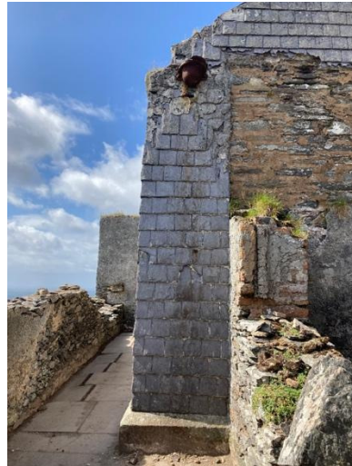
Fig.50. House (2), SE corner, hopper & downpipe.
