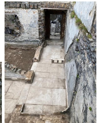
Fig.26. House (1), hall from south.
