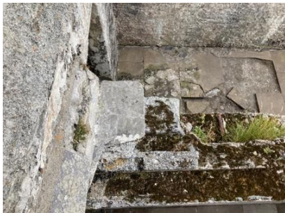
Fig.81. Outhouse (4) detail of roof.
