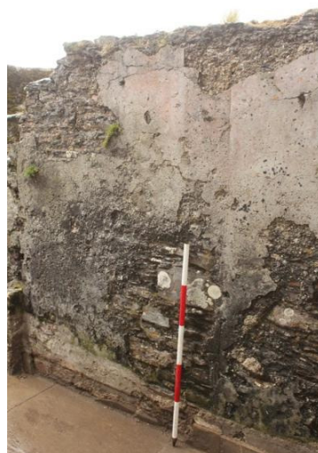
Fig.73. Outhouse (3), scar of original internal wall on west side wall.
