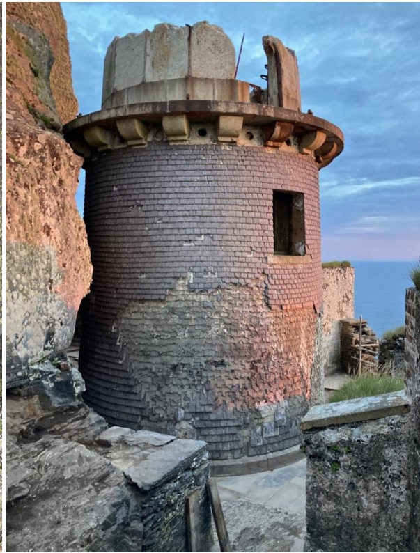
Fig. 87. The lighthouse from the north.
