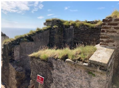
Fig.105. Roof level of Coal Shed.
