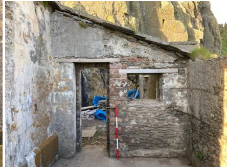
Fig.120. Inner face of front wall of Shed (21).
