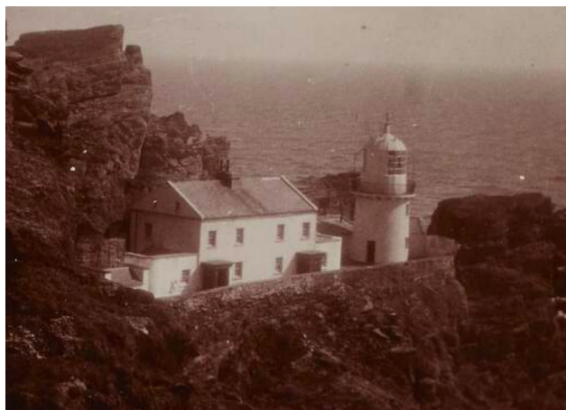
Fig. 167. The Lower Station in 1906.
