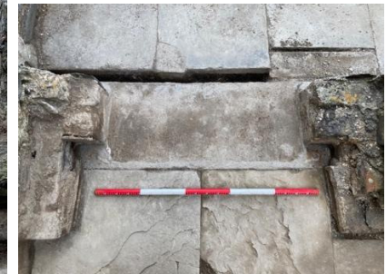
Fig.23. House (1) back door
