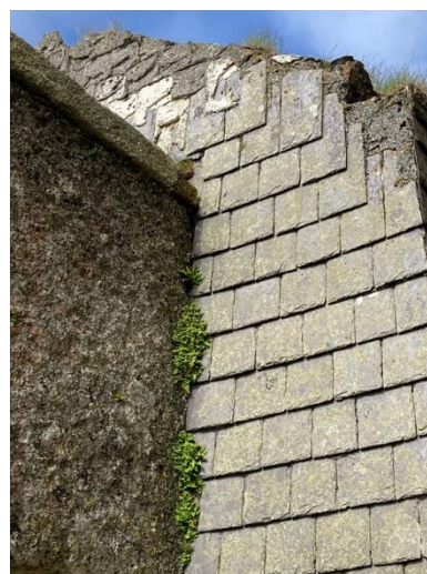
Fig.15. House (2), NE corner.
