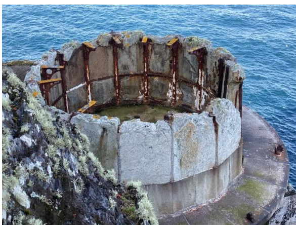
Fig.99. Second floor, balcony and mantlet from the north.
