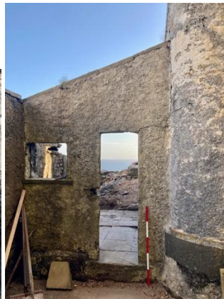
Fig.119. Front wall of Shed (21).
