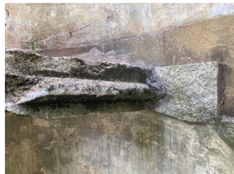
Fig.93. Detail of tongue of first floor granite slabs.
