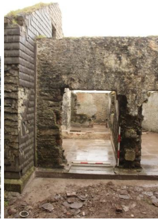
Fig.67. Front doorway of outhouse (3).
