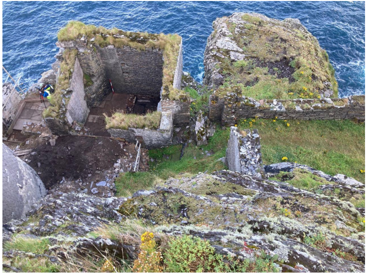
Fig.102. The Coal Shed (13) with the later Teacher's House (16) on the left.
