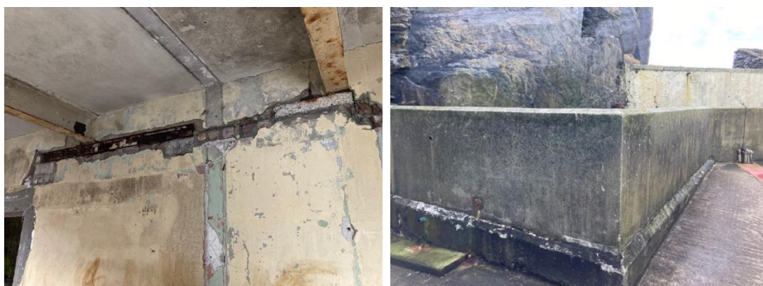
Fig. 172. (l.) Granite reused from the Upper Station, in this case a granite wall cap & (r.) The surviving chamfered plinth at the base of the demolished sheds in the Lower Station.
