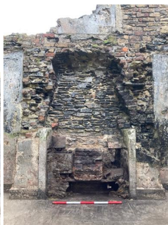
Fig.40. House (2), kitchen fireplace.
