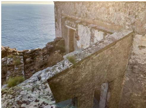
Fig.129. Roof of Sheds (21) and (23).
