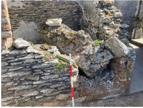
Fig.75. Outhouse (4), rear wall and room.
