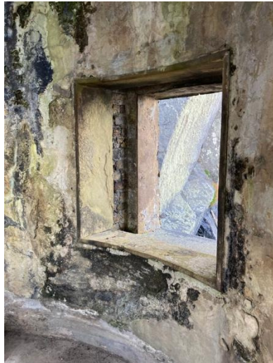
Fig. 95. First floor, SE window.
