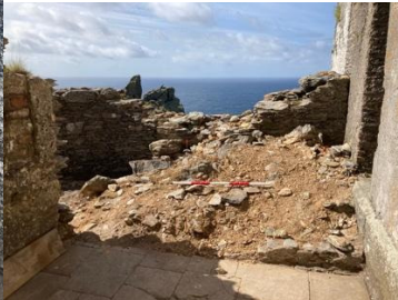
Fig. 127. The unexcavated end of Shed (23)
