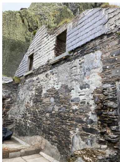
Fig.12. House (1), exterior west gable.
