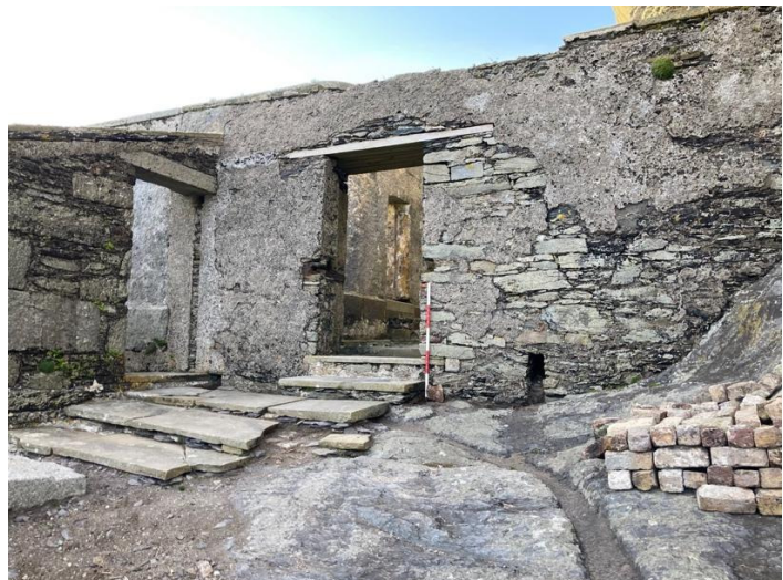
Fig.130. Phase 3 wall (22) with doorway, from the east.
