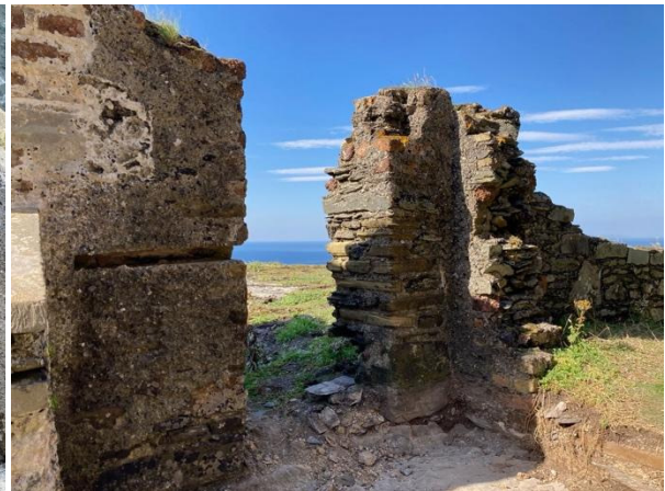
Fig. 114. Doorways to Toilet (17) (left) and (18) to North Terrace (right).
