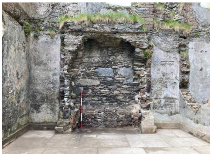
Fig.39. House (1), kitchen fireplace.
