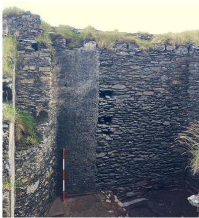
Fig.103. Coal Shed (13), west wall with later Chimney on left.
