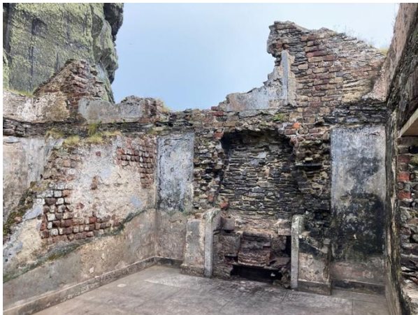
Fig.44. House (2), interior of east gable.
