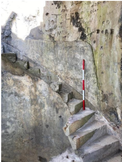
Fig.97. Stairs up to second floor.
