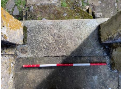
Fig.57. House (2), cill of doorway to yard (9).
