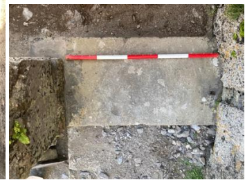
Fig.135. Shed (25), cill of doorway.
