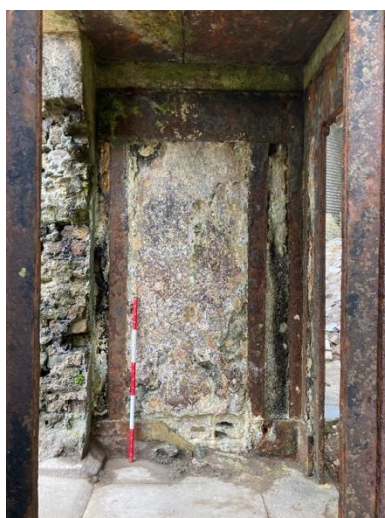
Fig.17. House (2), Interior of porch.
