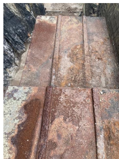
Fig.18. Roofs of porches, House (1) at bottom.
