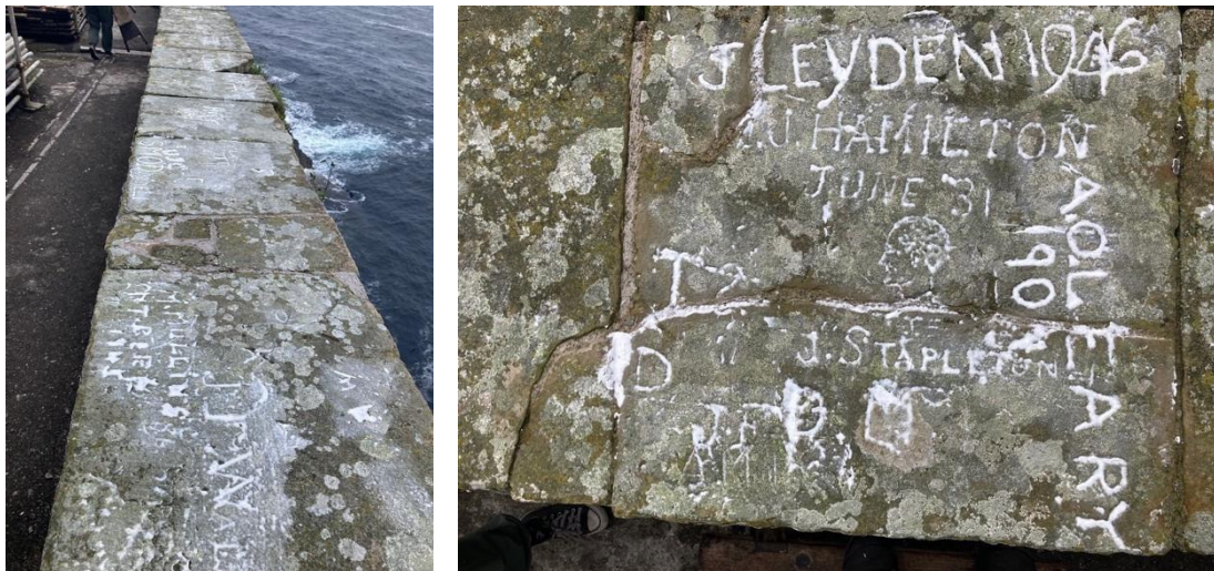
Fig.166. Some of the names carved into the top of the parapet wall beside the Lower Station filled with shaving foam to aid their recording.
