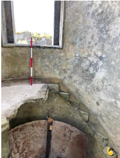
Fig.94. Top of stairs to first floor.
