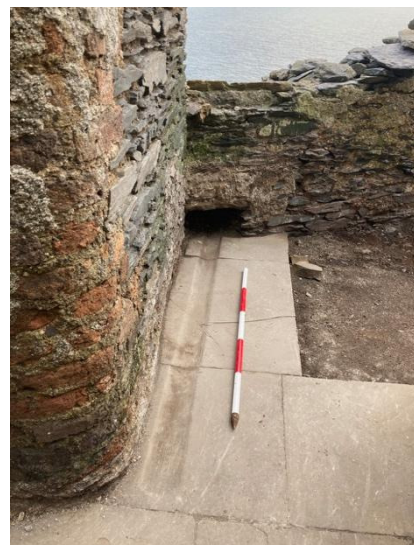
Fig.64. Drain at SE corner of yard (9).
