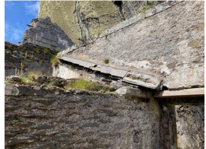
Fig.80. Outhouse (4) detail of roof.
