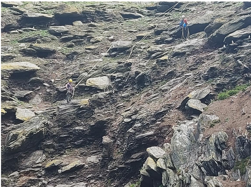
Image 7 Two sweepers at area 2 north of lower lighthouse
