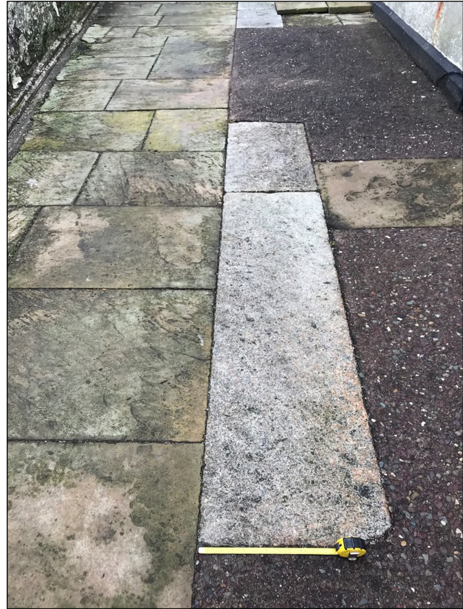
Photograph 4: Lower Lighthouse View to Northeast. Detail of Relationship Between Yorkshire Flagstone (left) and Wicklow Granite Setts (right).
