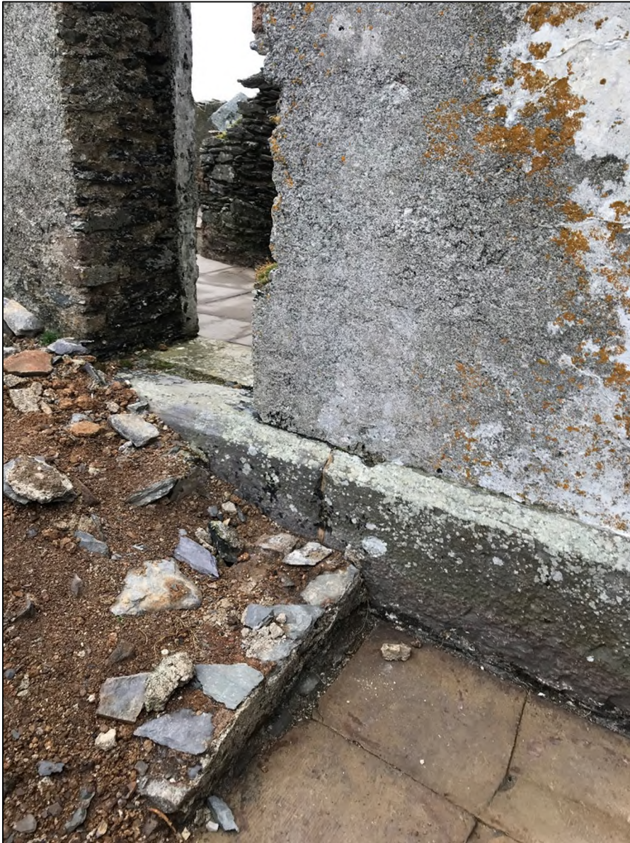
Photograph 27: Lighthouse Keepers' Cottages Base Plinth in Valentia Slate.
