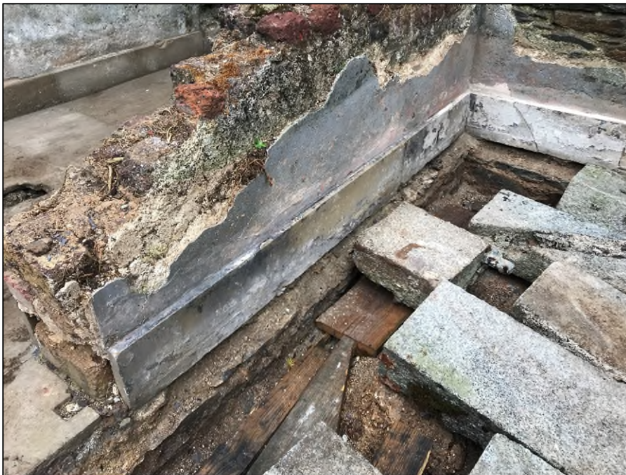
Photograph 21: Yorkshire Flagstone "Skirting Board" in Lighthouse Keepers' Cottages.
