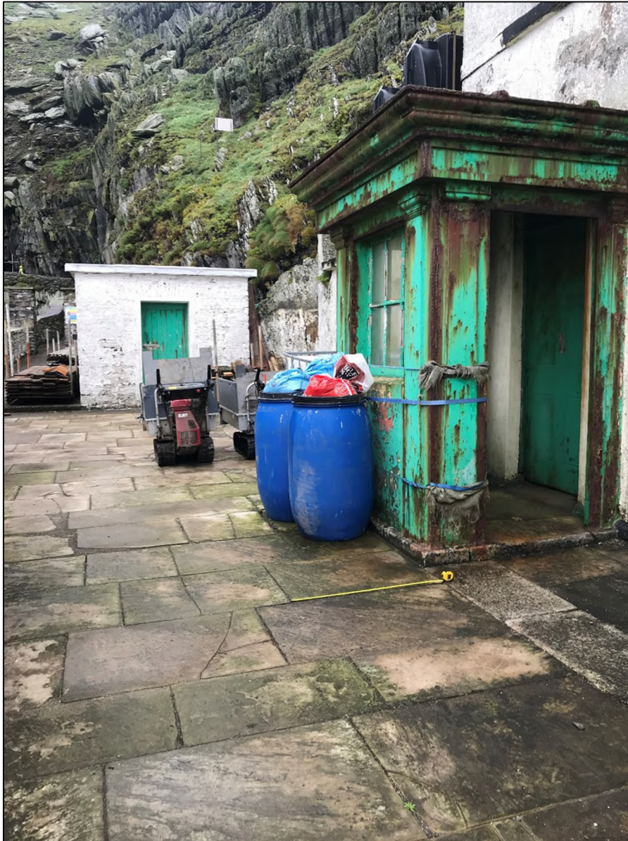
Photograph 1: Lower Lighthouse View to Northeast Showing Main Cast Iron Doorway. Note Yorkshire Flagstones (left) and Wicklow Granite Setts (right).
