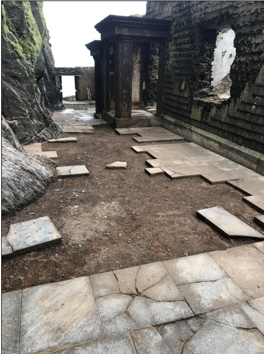
Photograph 17: Upper Lighthouse View to Southeast. Yorkshire Flagstone Setts in Front of Lighthouse Keepers' Cottages.
