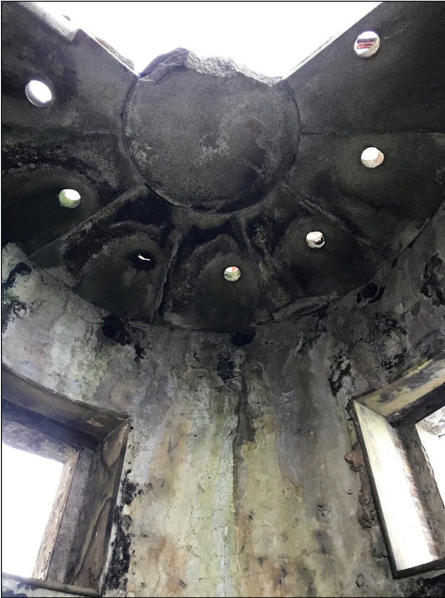
Photograph 31: Upper Lighthouse Wicklow Granite Corbel Plinth Roof with Yorkshire Flagstone Surrounds to Window Openings.
