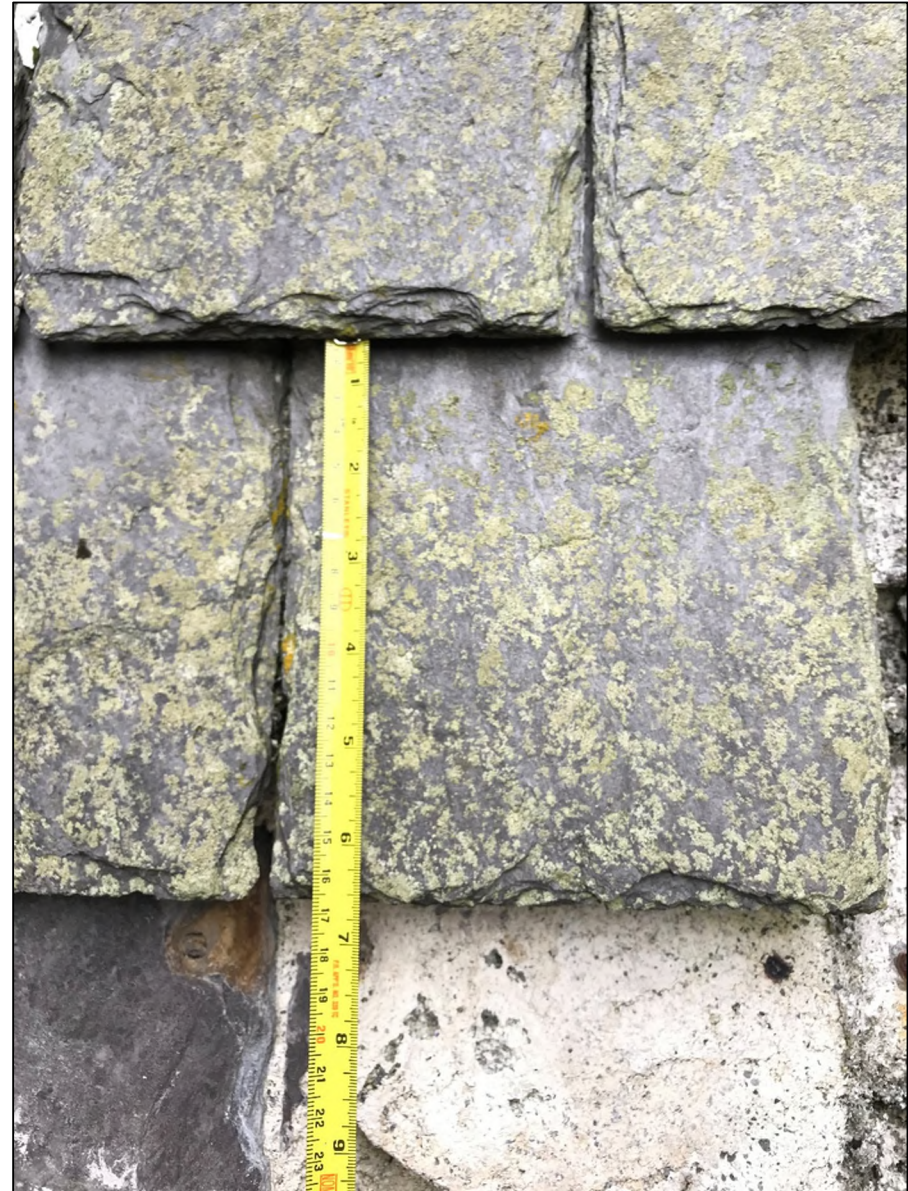
Photograph 26: Lighthouse Keepers' Cottages Cladded in Valentia Slate.
