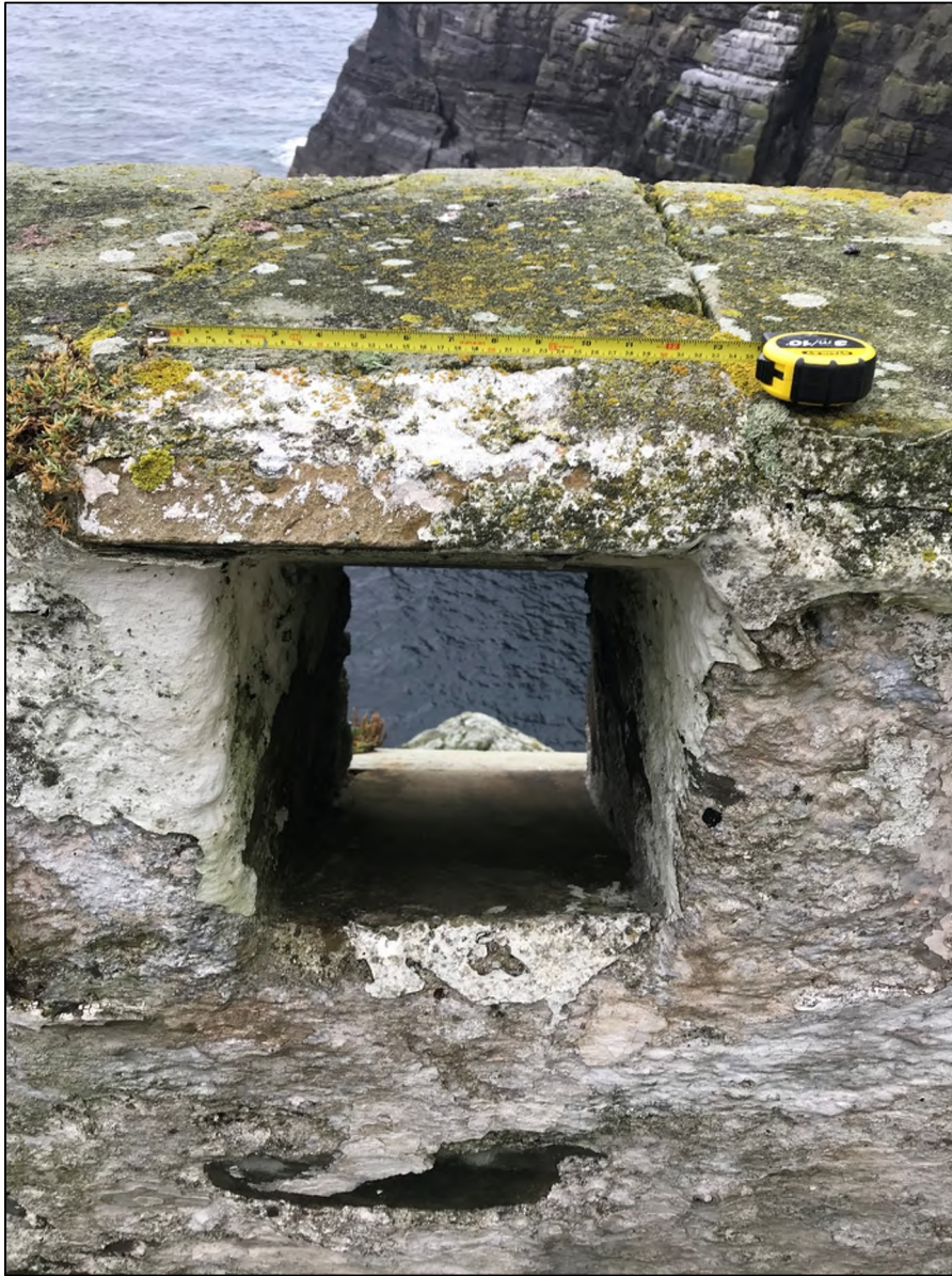
Photograph 7: Lower Lighthouse. Waste Chute to Seaward With Thick Yorkshire Flagstone Cap.
