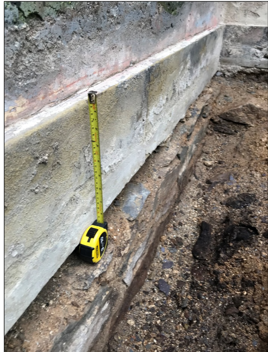
Photograph 22: Detail of Yorkshire Flagstone "Skirting Board" in Lighthouse Keepers' Cottages.
