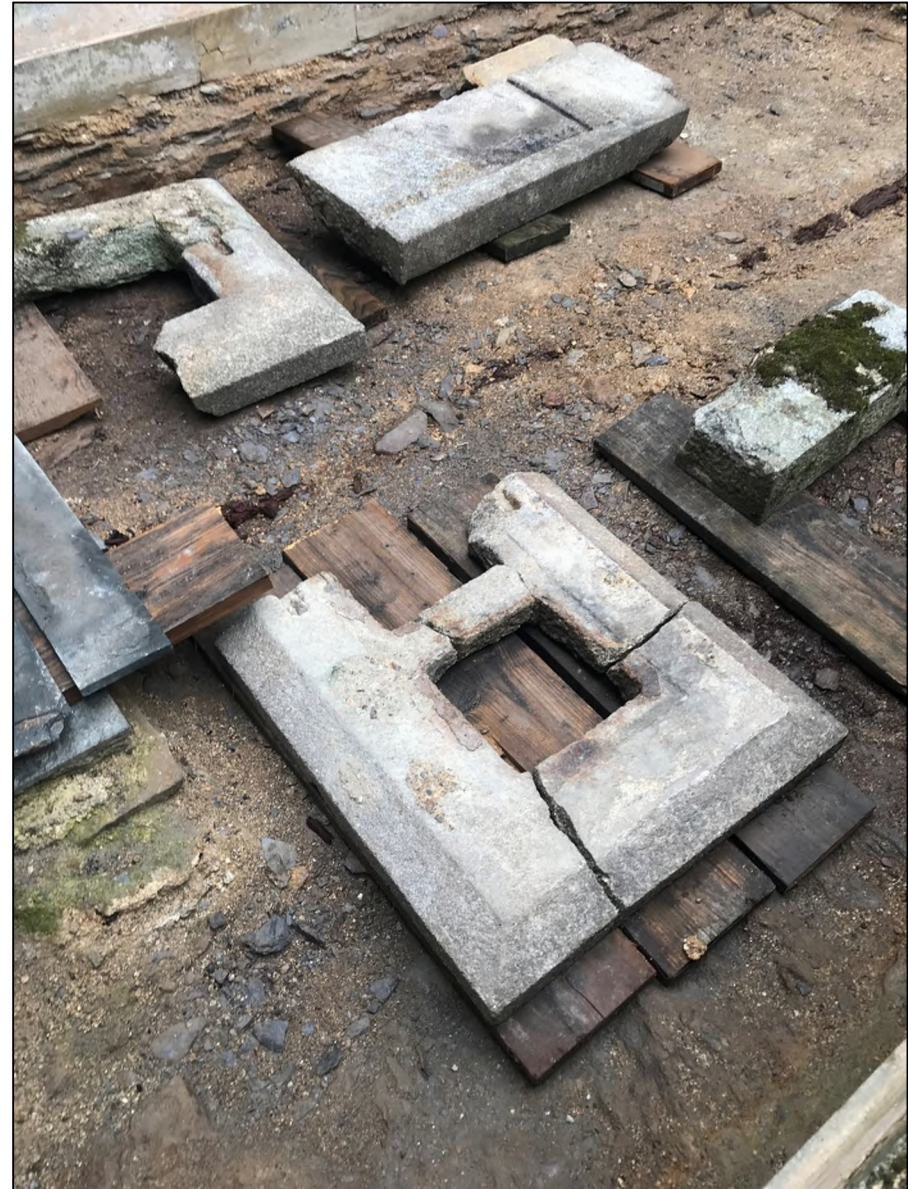
Photograph 24: Lighthouse Keepers' Cottages Chimney Basal Plinth in Wicklow Granite.
