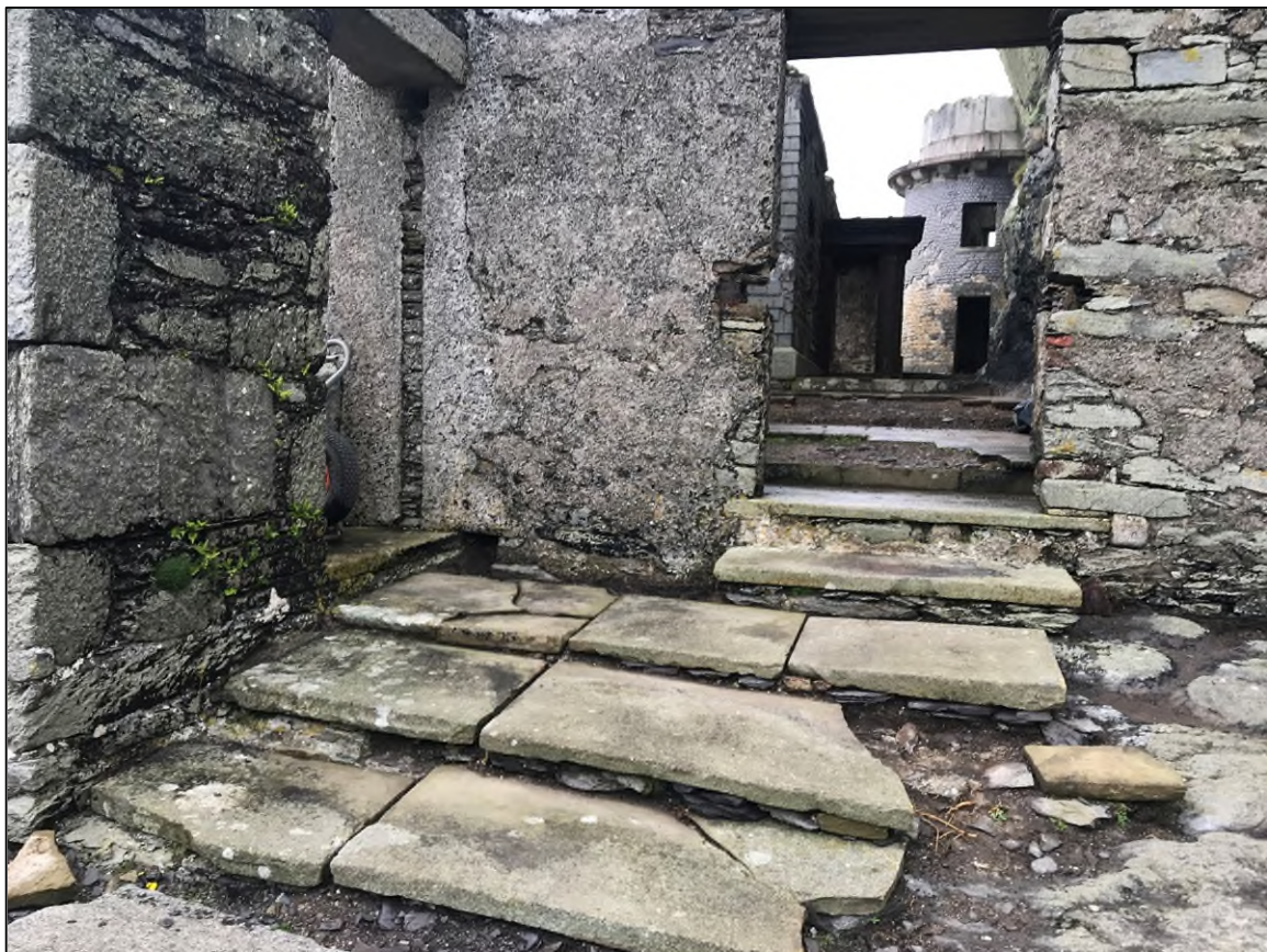
Photograph 16: Upper Lighthouse Entrance With Yorkshire Flagstone Steps.
