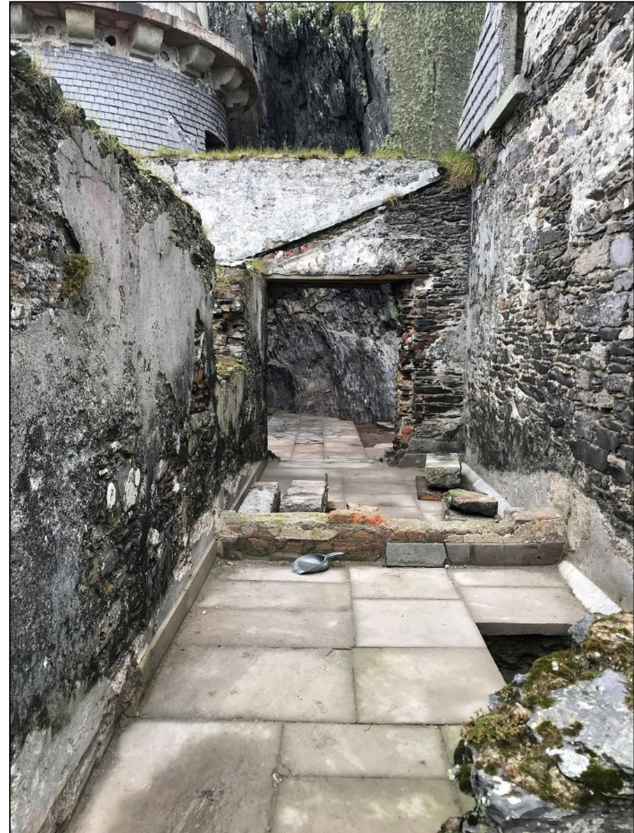
Photograph 18: Upper Lighthouse View to Northeast. Yorkshire Flagstone Setts in Extension to Lighthouse Keepers' Cottages.
