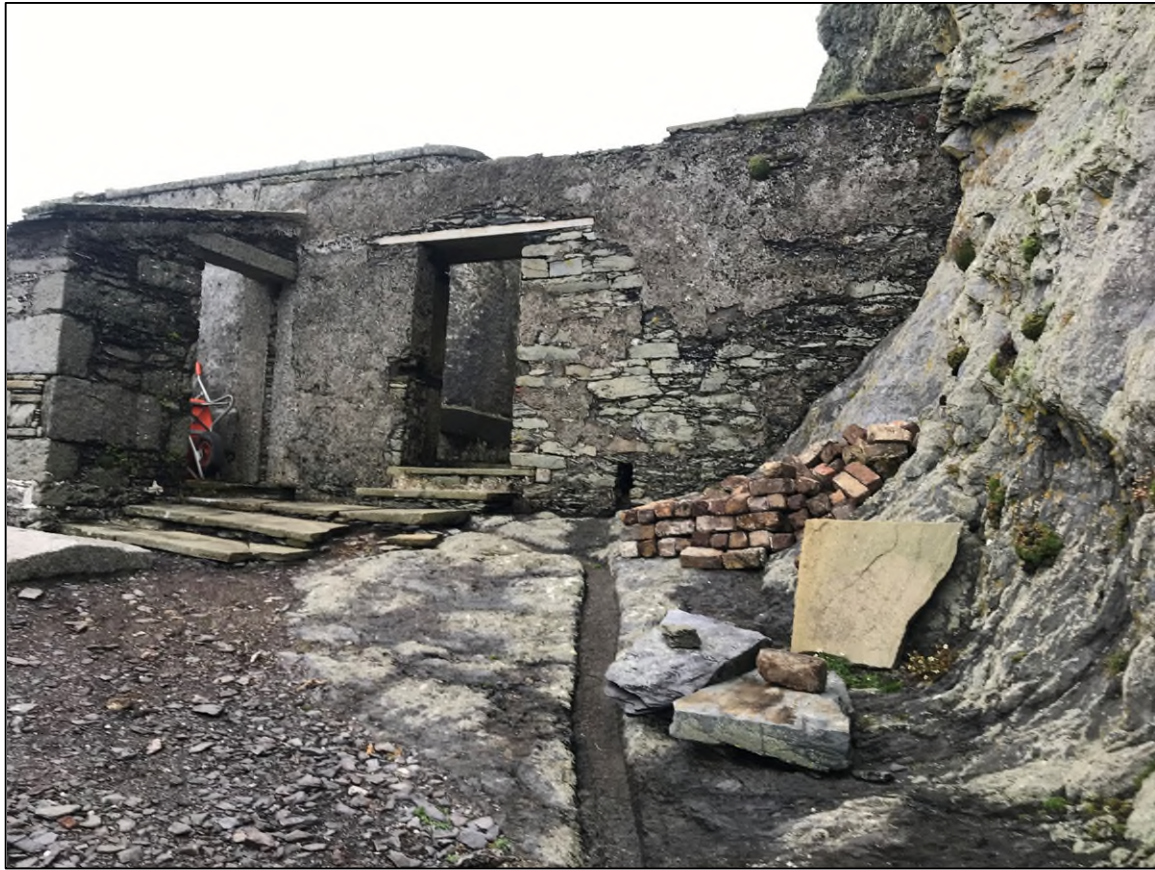
Photograph 15: Upper Lighthouse Entrance With Bedrock Surface Water Drainage Channel.
