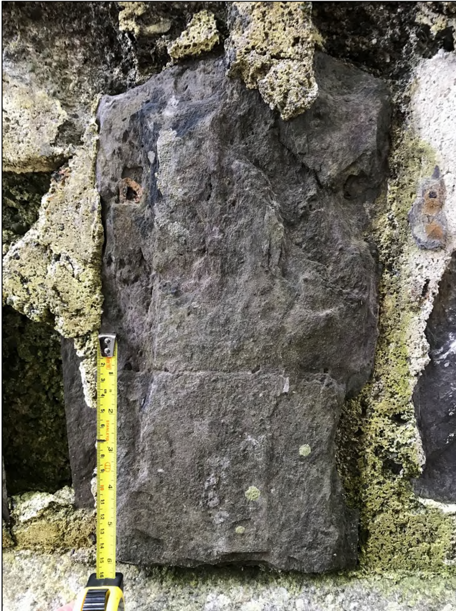
Photograph 25: Lighthouse Keepers' Cottages Cladded in Skellig (Silty) Sandstone.
