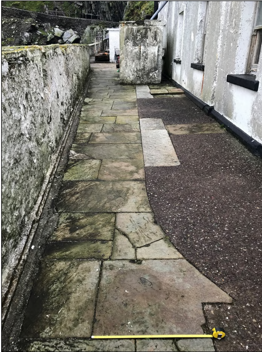
Photograph 3: Lower Lighthouse View to Northeast. Note Yorkshire Flagstones (left) and Wicklow Granite Setts (right).
