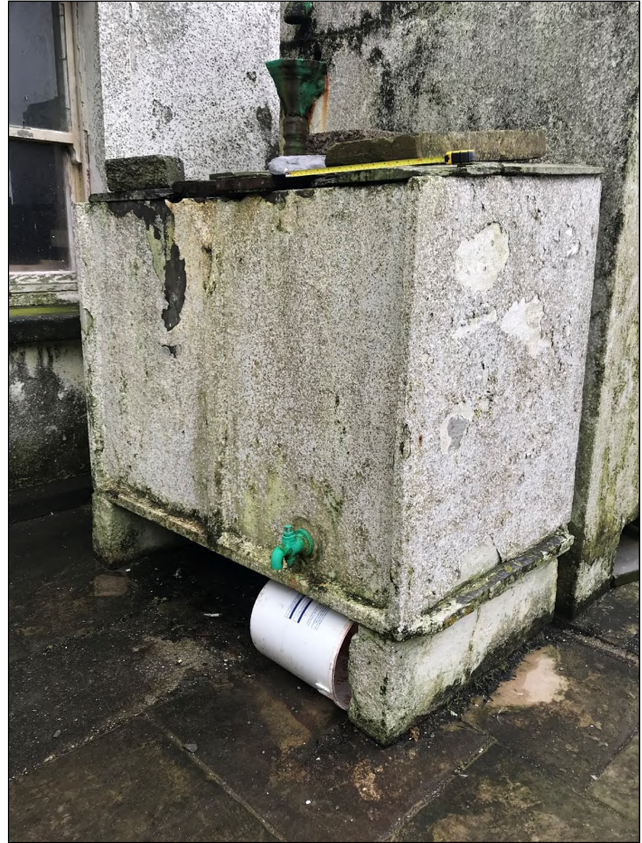
Photograph 6: Lower Lighthouse. Water Cistern Constructed From Valentia Slate.
