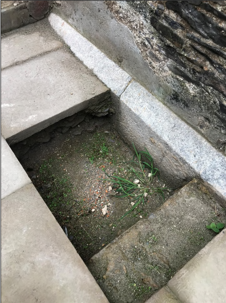
Photograph 19: Detail of Wicklow Granite Base Plinth to Lighthouse Keepers' Cottages.
