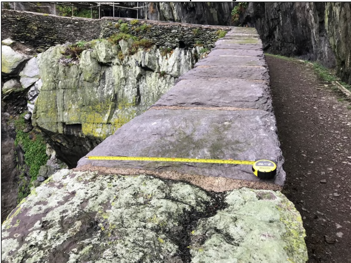
Photograph 10: Lighthouse Road Lower Section. "Old" Skellig Sandstone Cap in Foreground, "New" Valentia Slate Caps in Background.
