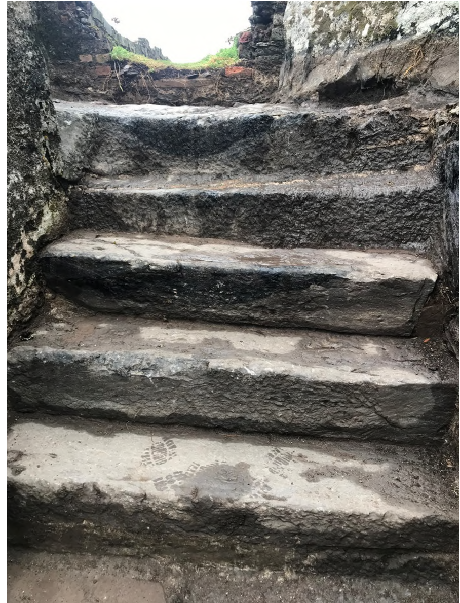
Photograph 28: Mix of Bedrock Cut Steps and Valentia Slate (?) Stone Steps to Northeast of Upper Lighthouse.
