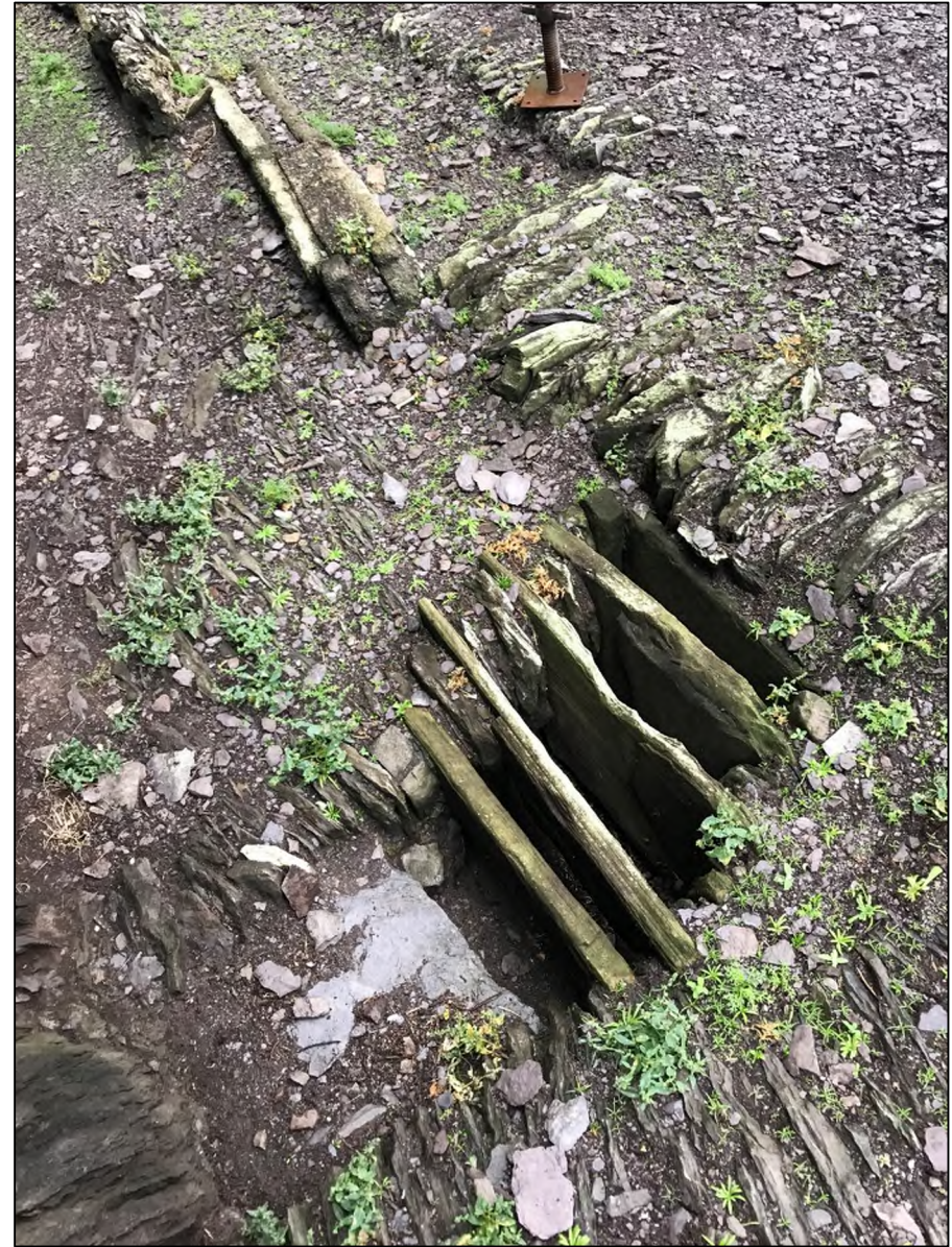
Photograph 8: Lower Lighthouse. Yorkshire Flagstone "Grill" at Surface Water Drainage Outlet.
