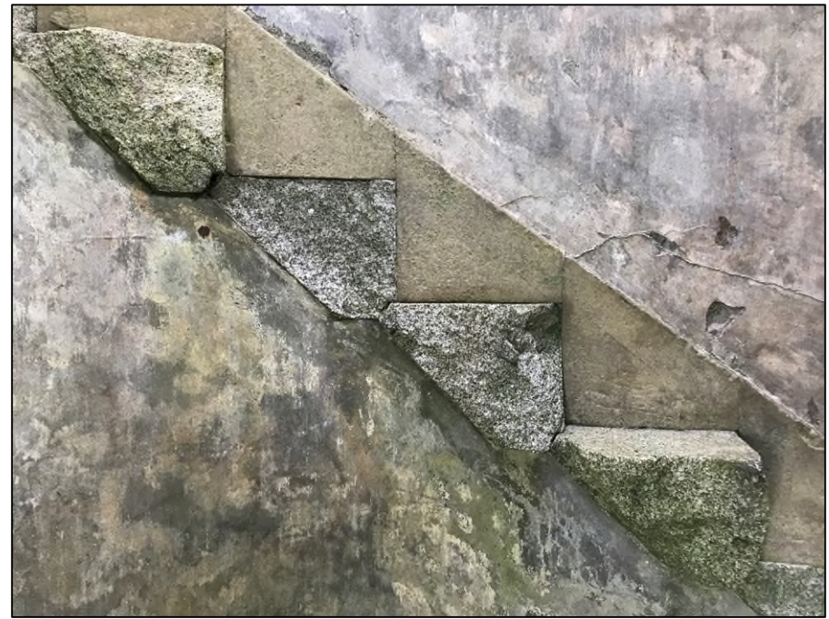
Photograph 32: Upper Lighthouse Wicklow Granite Cantilevered Steps.
