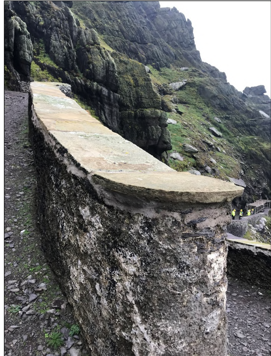
Photograph 12: Lighthouse Road Upper Section Dog-leg. Yorkshire Flagstone Caps on Skellig Sandstone Rubble Wall.
