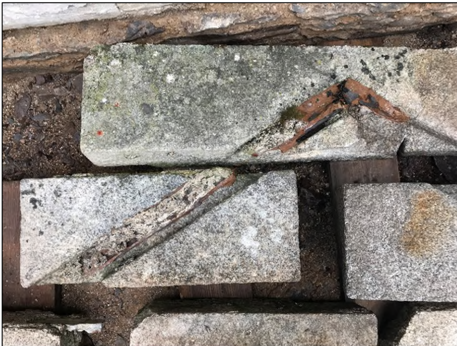
Photograph 23: Lighthouse Keepers' Cottages Roof Barge in Wicklow Granite Showing Outline of Roof Apex.
