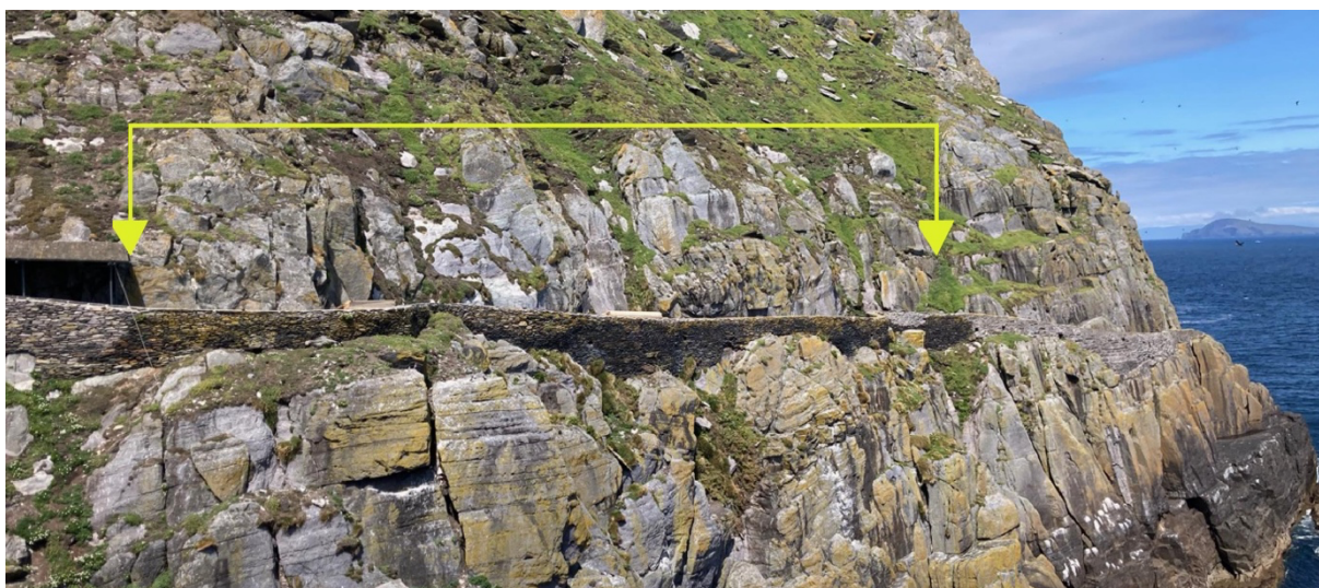
Fig. 2. The length of roadway to be canopied, viewed from the helipad.
