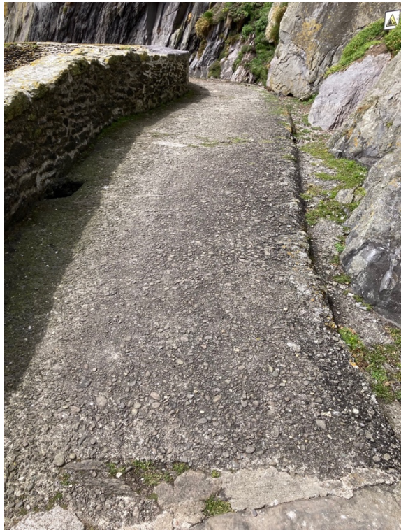
Photo 2. Concrete road surface and lateral drain
