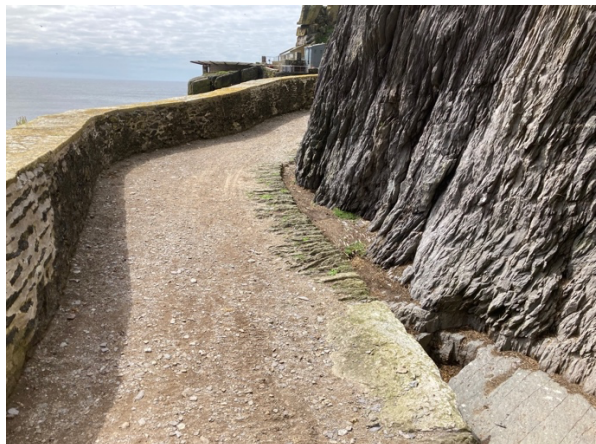
Photo 4. Rock cut drain and lateral drain base on right.
