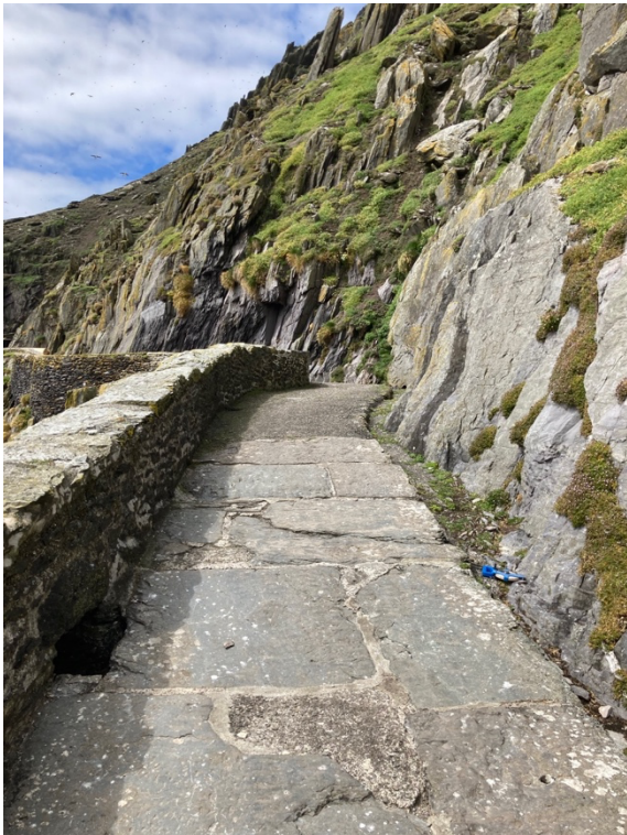
Photo 1. Stone paved road surface.
