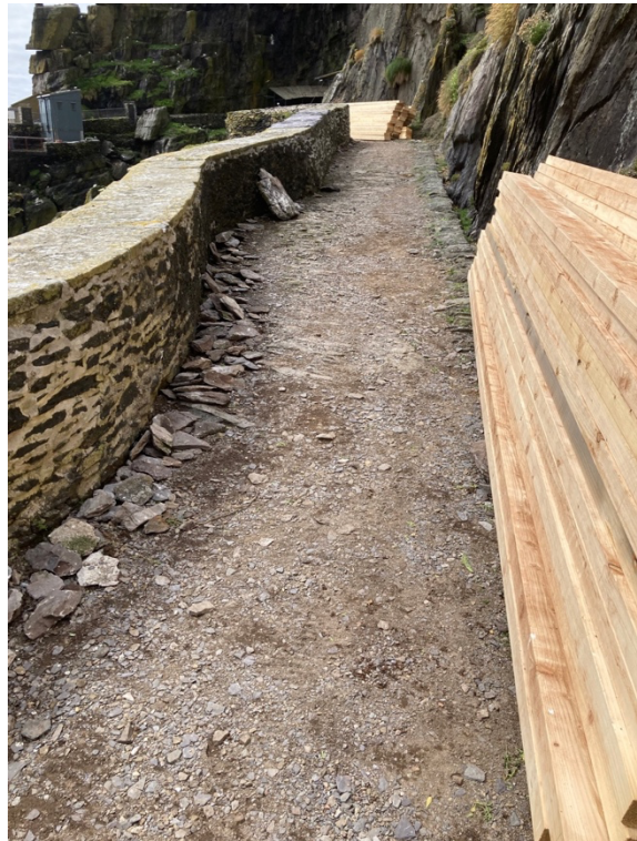
Photo 6. Vertically set stone surface on roadway
