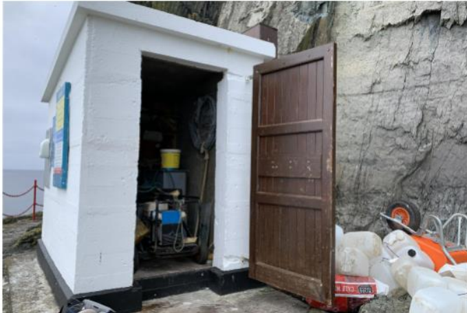
03 FRONT ELEVATION, SHED ENTRANCE 007
