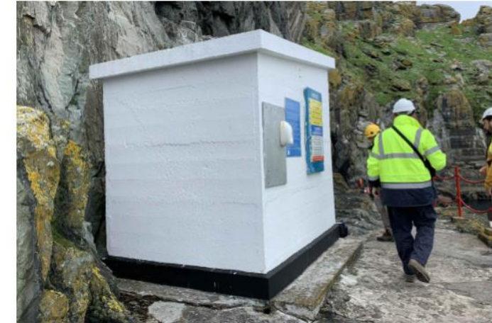
04 REAR VIEW OF SHED, PROPOSED LOCATION FOR CCTV CAMERA 007
