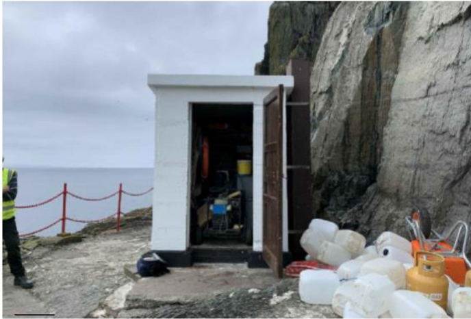
01 FRONT ELEVATION, SHED ENTRANCE 007
