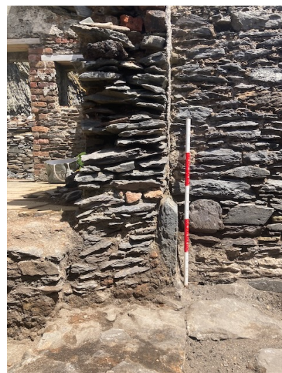
Fig. 13. Shed 21, east wall with fake plinth.
