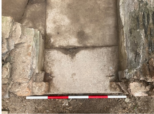
Fig. 3. Detail of doorway of shed 4a.
