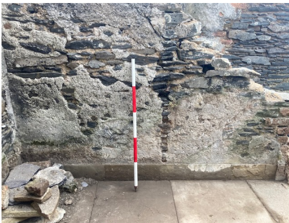
Fig. 6. East wall of shed 4a, scars of shelving.
