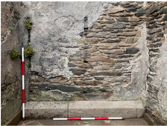
Fig. 4. West wall of shed 4a, scars of shelving.
