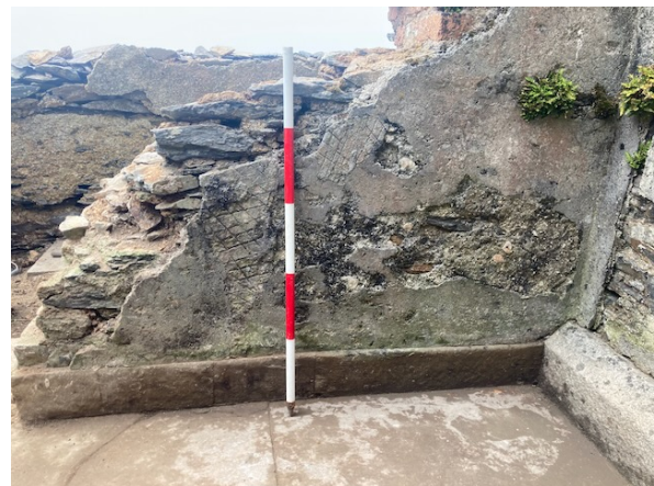
Fig. 7. South wall of shed 4a, scars of shelving.
