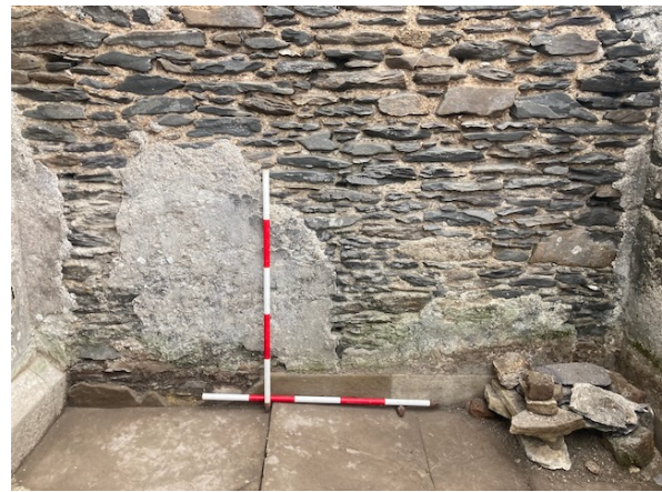
Fig. 5. North wall of shed 4a, scars of shelving.
