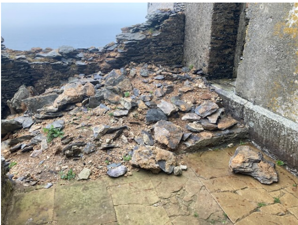
Fig. 10. Shed 21, south end before excavation.
