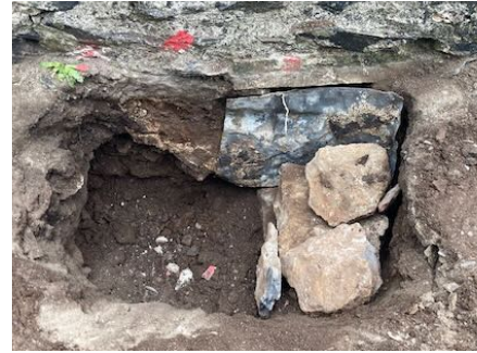
Fig 8. Drain ope sealed before backfilling.
