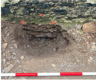
Fig. 6. Typical foundation for pole on outer side of canopy.
