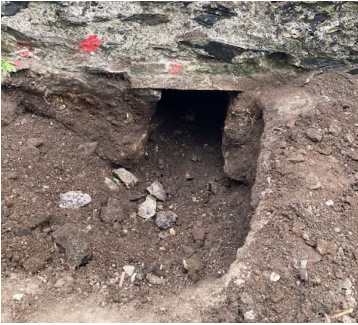
Fig. 7. Disused drain ope uncovered.
