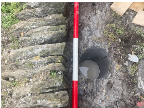
Fig. 4. Cored hole, inner side of roadway.
