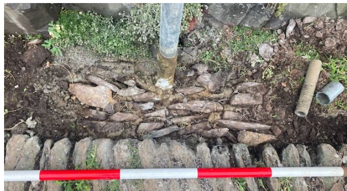
Fig. 5. Stones of lateral drain replaced after construction.
