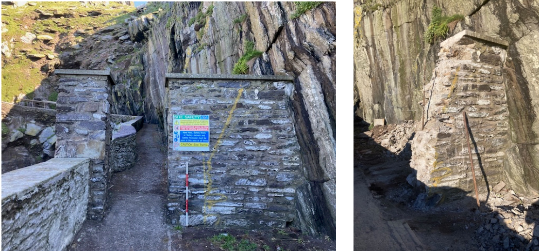
Fig. 3. The north gateway of the lighthouse before and after removal of part of its east side.
