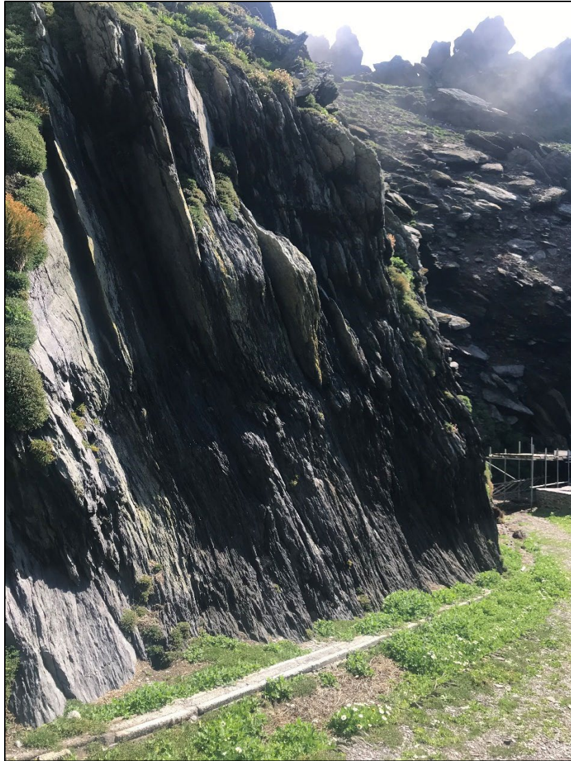
Photograph 03. Upper Lighthouse Road – Section 3.
