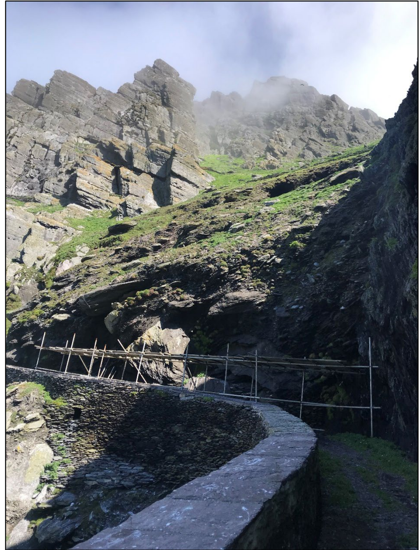
Photograph 04. Upper Lighthouse Road – Section 4.
