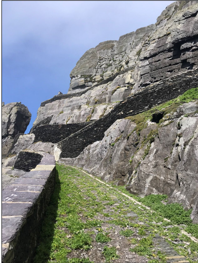
Photograph 04. Upper Lighthouse Road – Section 5.
