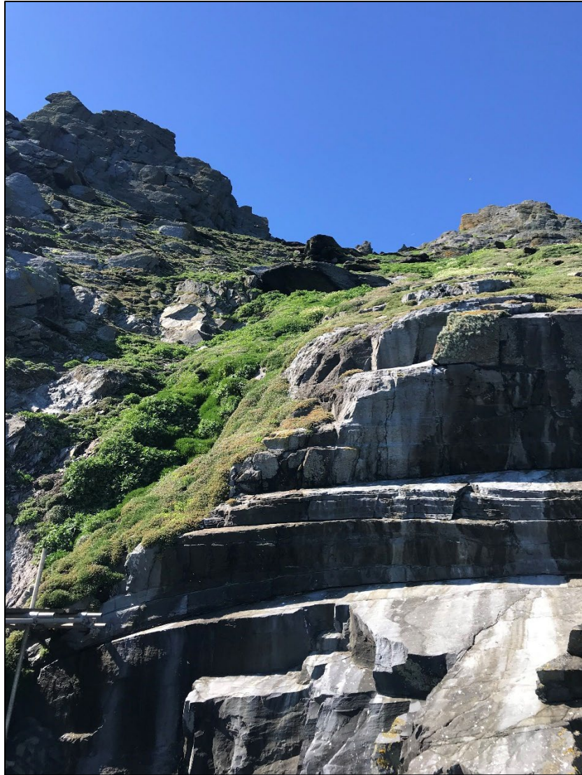
Photograph 08. Lower Lighthouse Road – Section 3.
