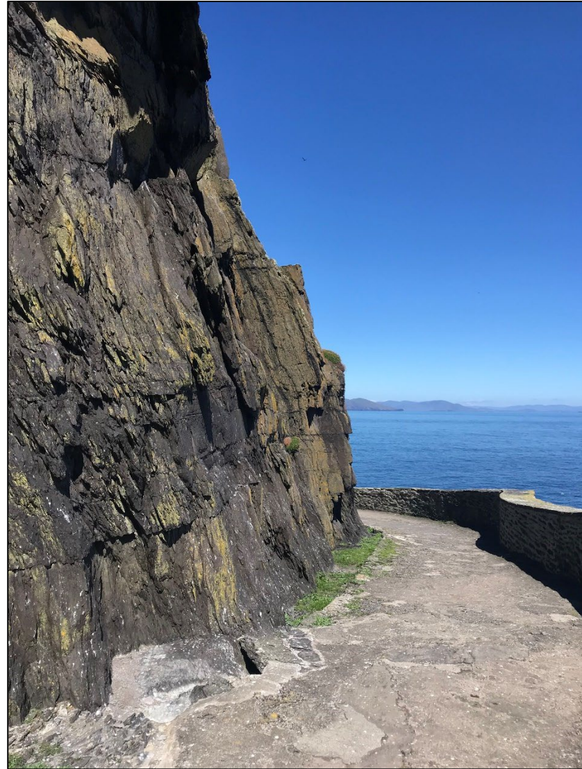
Photograph 09. Lower Lighthouse Road – Section 4.
