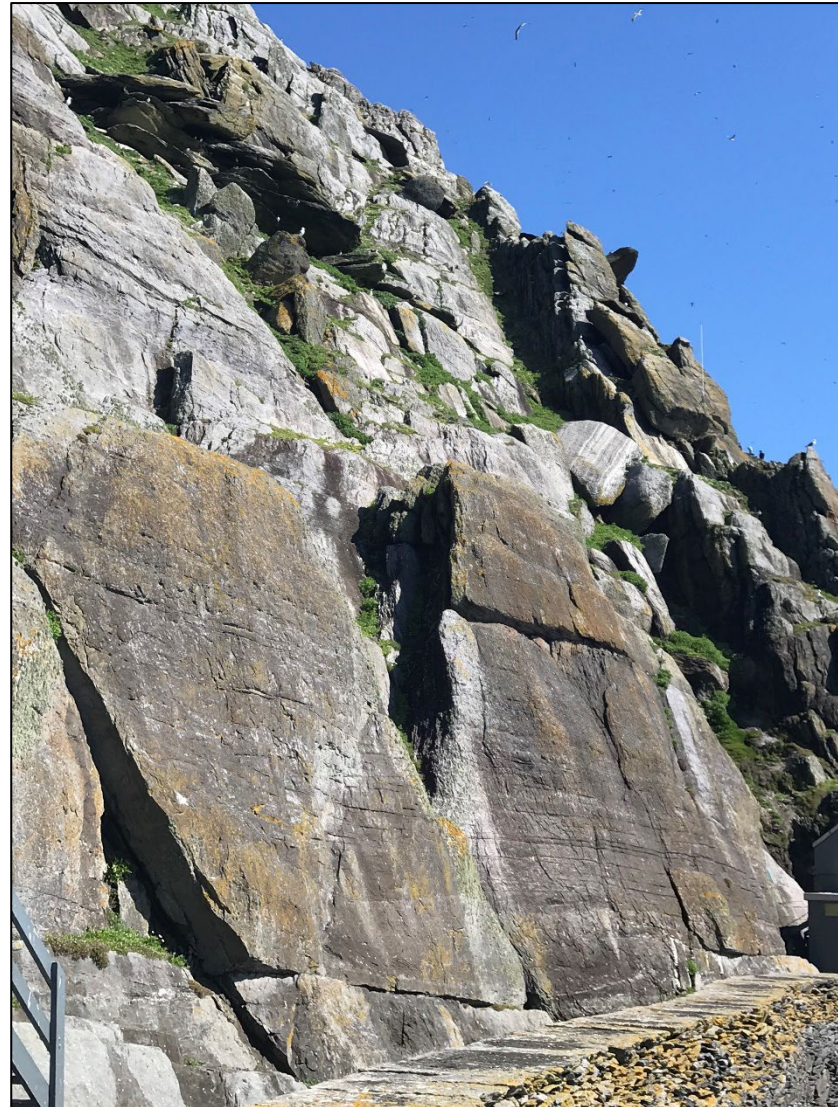
Photograph 07. Lower Lighthouse Road – Section 2.
