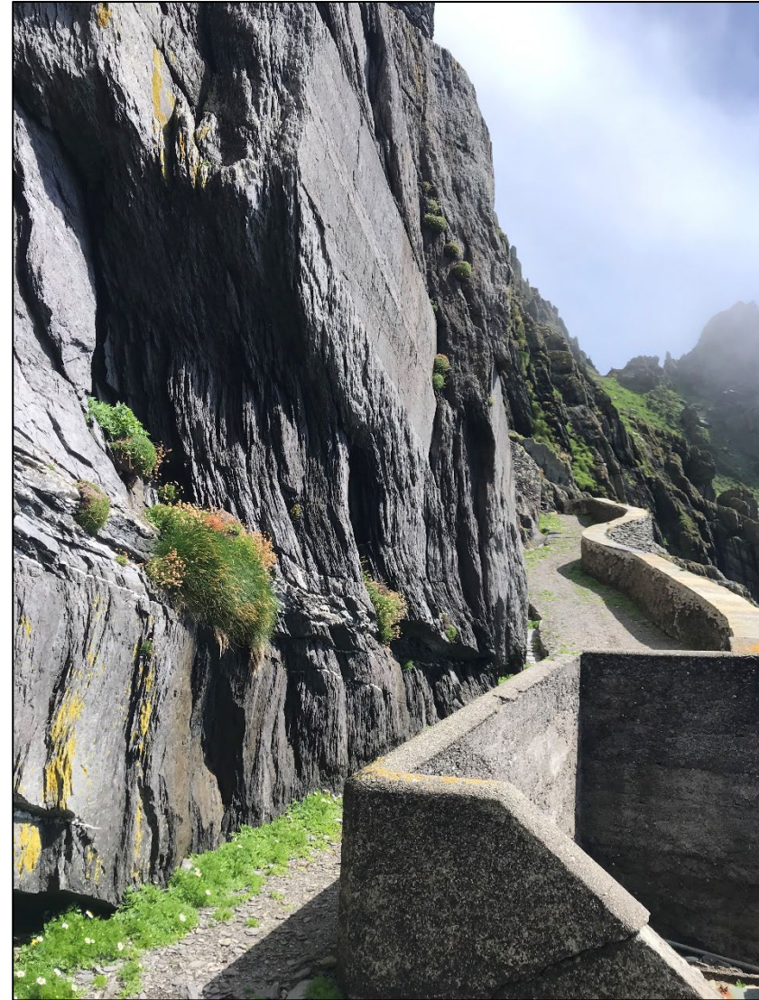
Photograph 05. Upper Lighthouse Road – Section 6.
