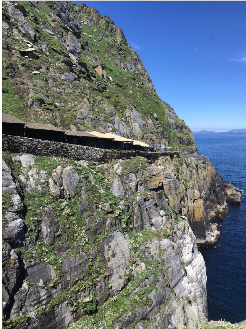
Photograph 10. Lower Lighthouse Road – Section 5.
