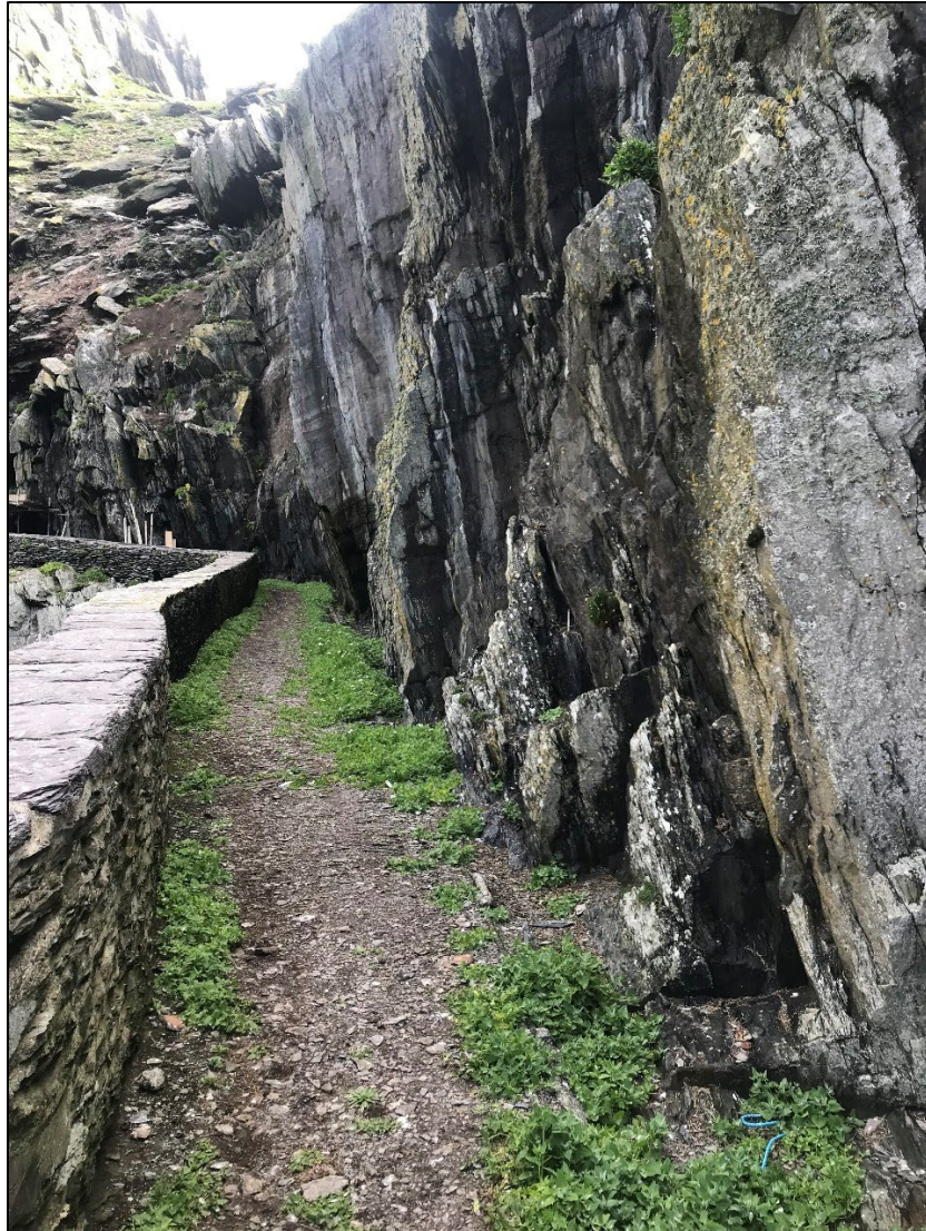
Photograph 01. Upper Lighthouse Road – Section 1.
