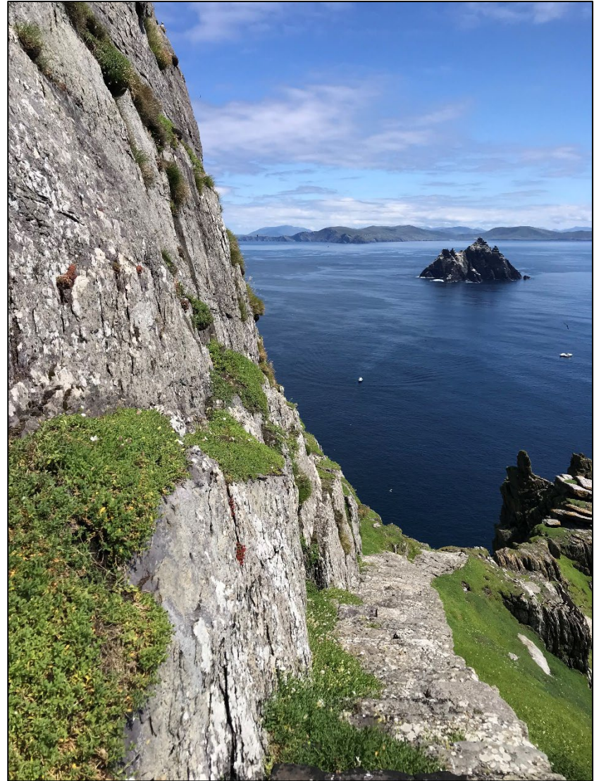
Photograph 13. East Steps – Section 1.
