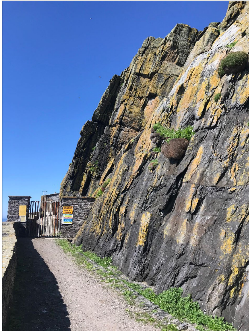
Photograph 06. Lower Lighthouse Road – Section 1.
