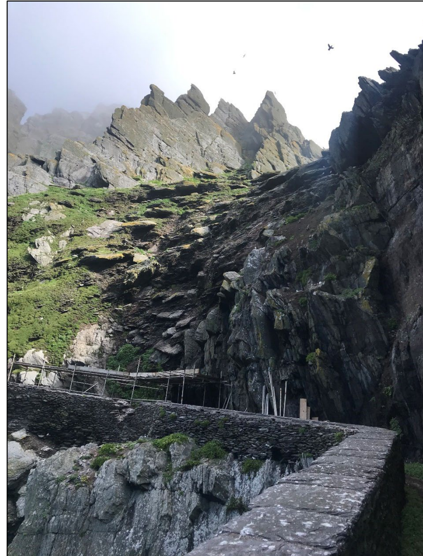
Photograph 02. Upper Lighthouse Road – Section 2.
