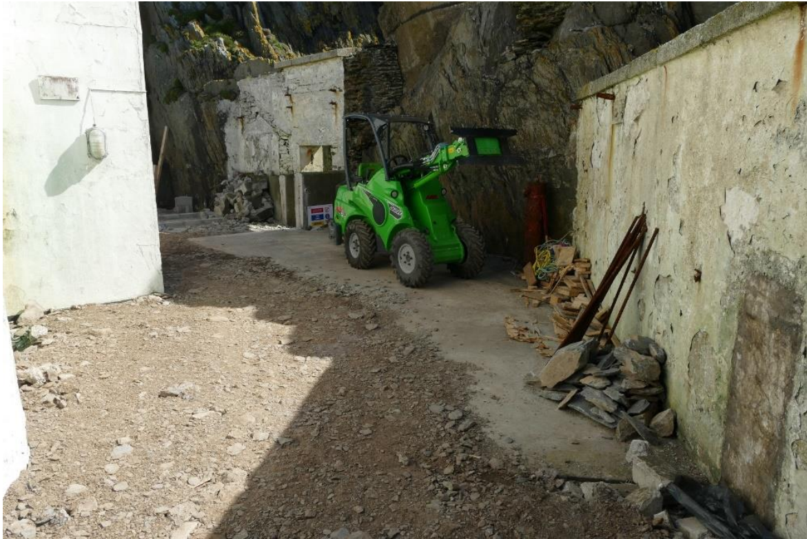
Fig. 14. - Bund wall removed at the Lower Lighthouse compound
