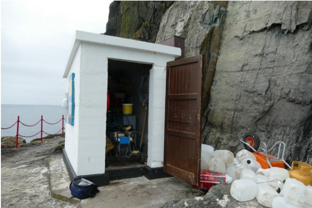
Fig. 50. - Proposed location of CCTV on the storage building adjacent to the landing pier
