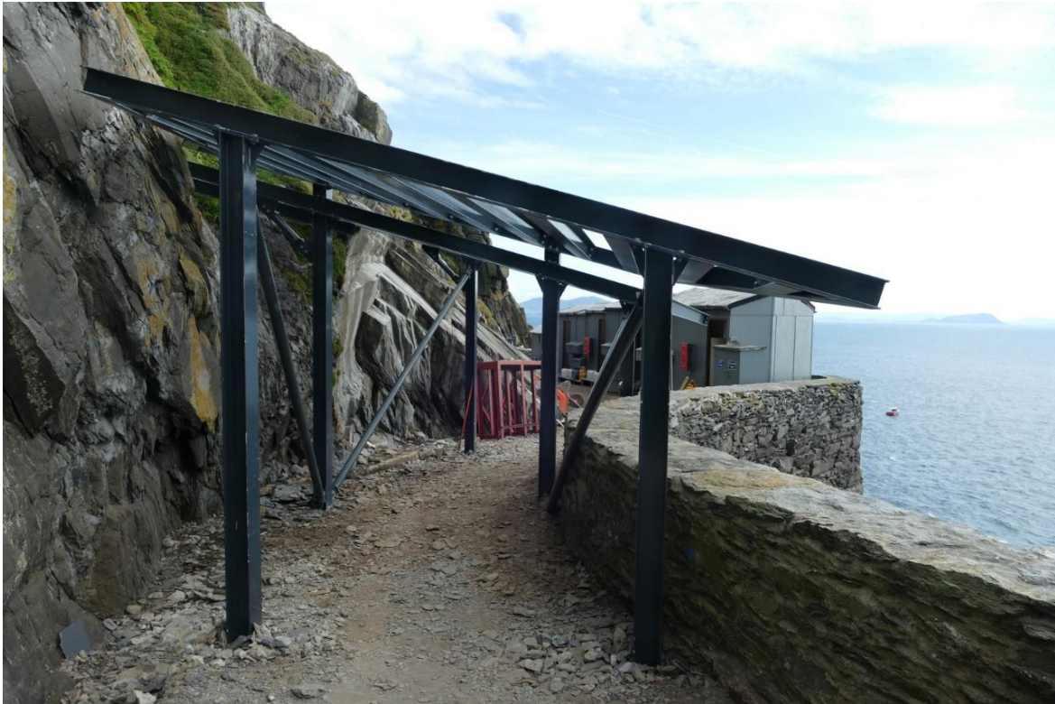
Fig. 44. - Crash Deck No. 1 – Steel structure installed on site
