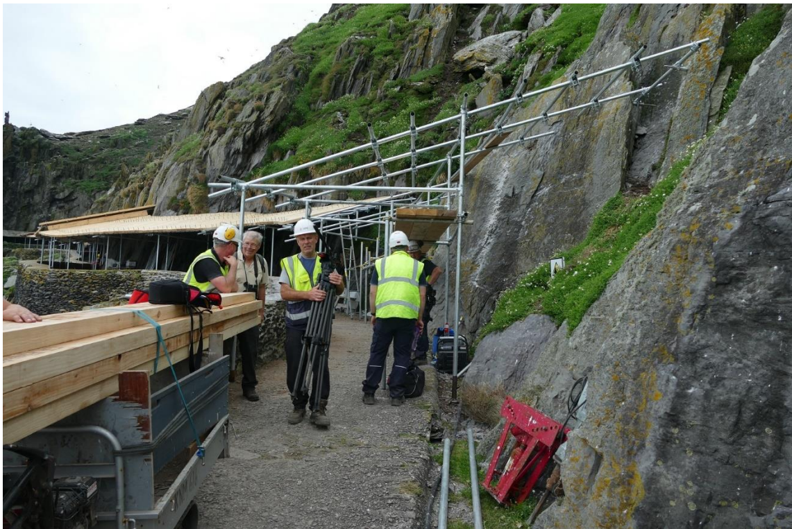
Fig. 36. - View of the canopy being installed at the Lower Lighthouse road following the rock fall that occurred on 13 th June 2022
