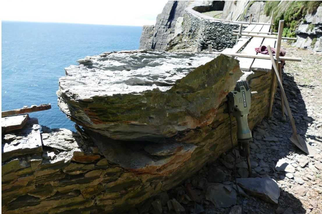
Fig. 39. - View of the rock fall in the location of crash deck no.2 on the Upper Lighthouse road
