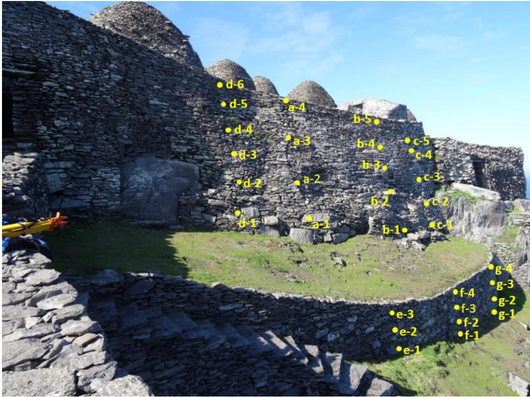
Fig. 12. - Discovery Programmed marker point locations at monastery retaining wall
