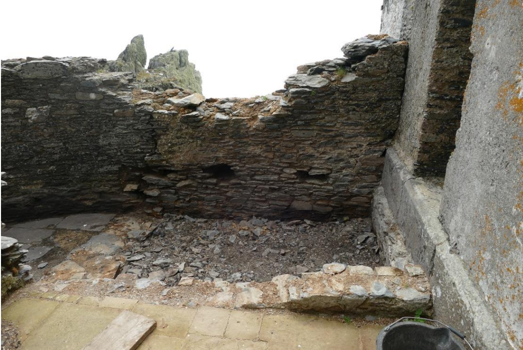
Fig. 11. - Removal of debris at the Upper Lighthouse
