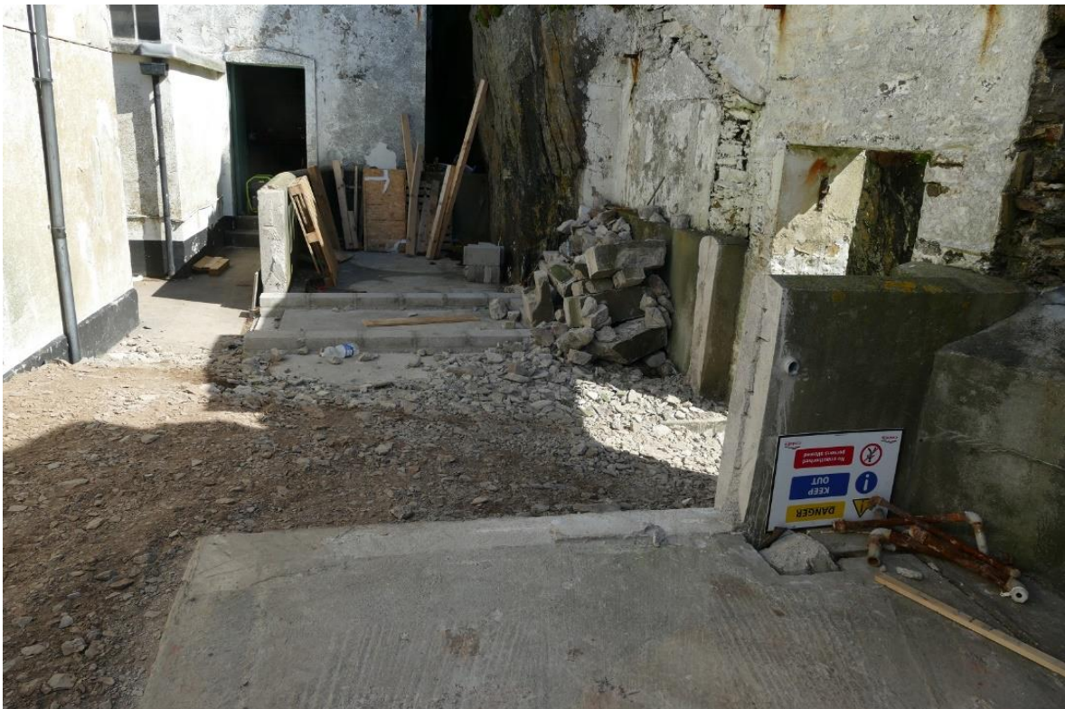
Fig. 15. - Bund wall removed at the Lower Lighthouse compound
