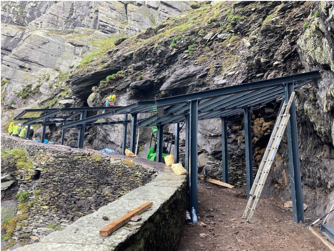
Fig. 49. - Crash Deck No. 3 – Steel structure installed on site
