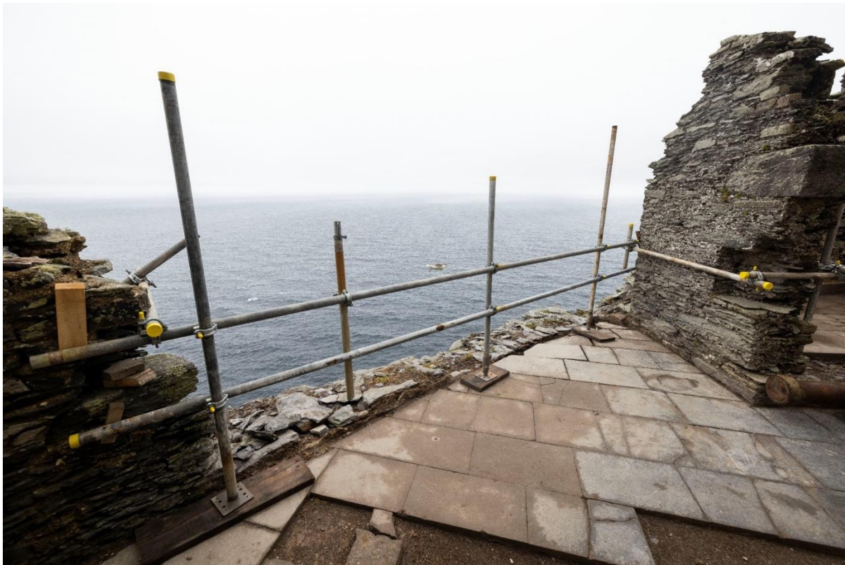
Fig. 19. - View of the existing sea wall at the Upper Lighthouse
