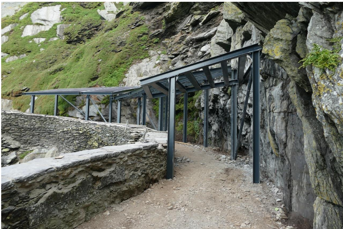
Fig. 45. - Crash Deck No. 2 – Steel structure installed on site
