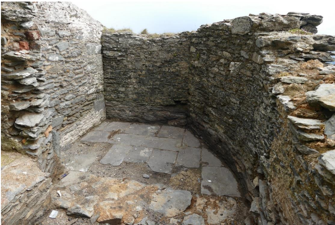
Fig. 10. - Removal of debris at the Upper Lighthouse
