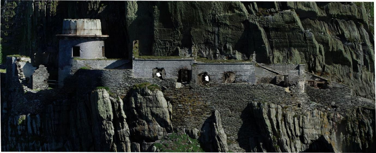
Fig. 18. - Aerial view of the Upper Lighthouse and sea wall
