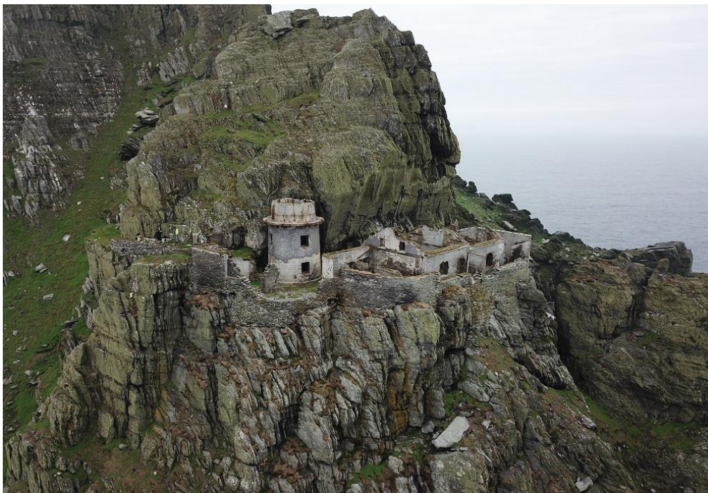
Fig. 17. - Aerial view of the Upper Lighthouse and sea wall
