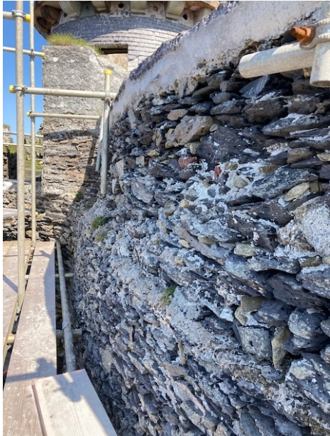
Fig. 11. Raised top of north end of south wall.
