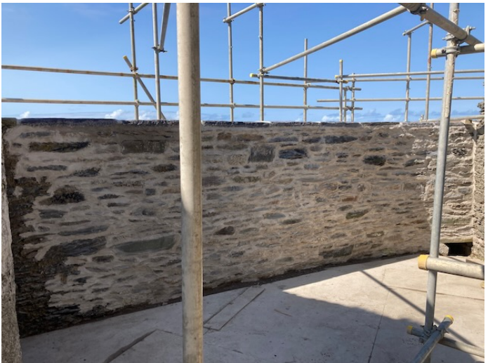
Fig. 12. Rebuilt parapet of north wall.
