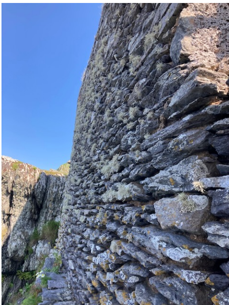
Fig. 13. North wall exterior.
