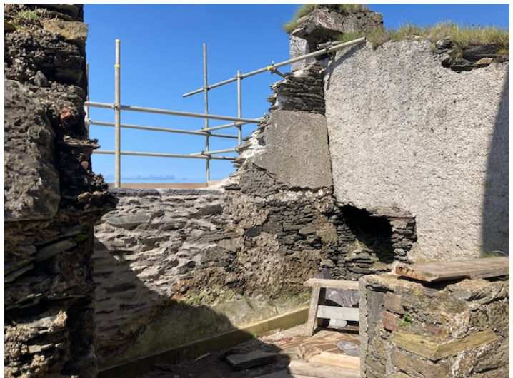
Fig. 14. Rebuilt section of wall in 'Teacher's House'.
