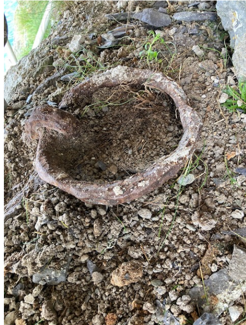
Fig. 10. Iron ring fixed to rock at base of wall.
