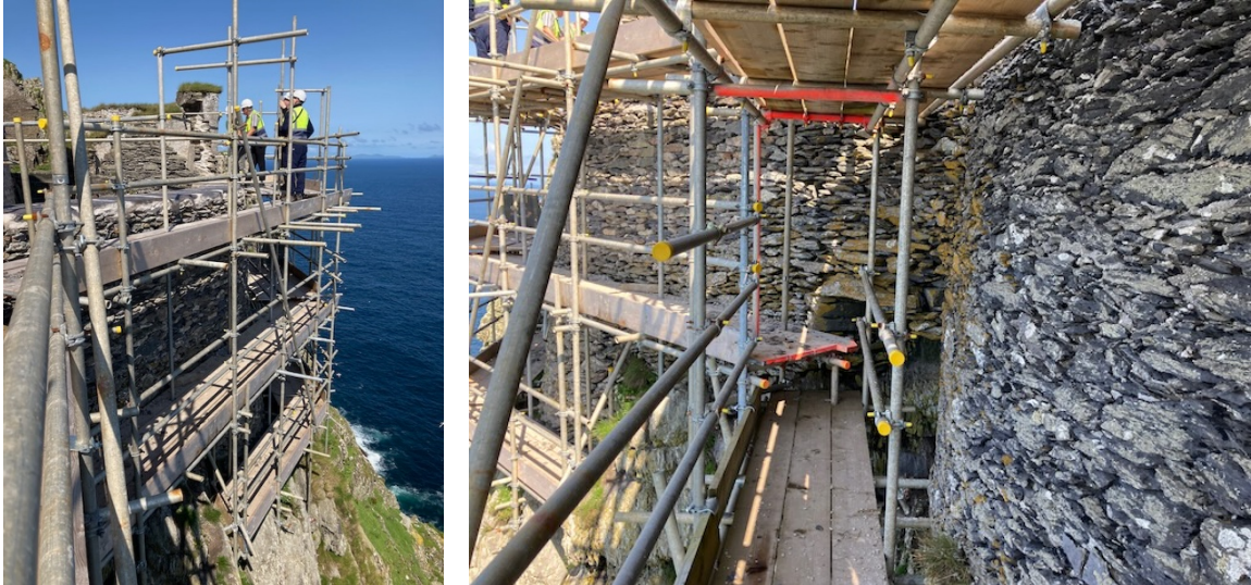
Fig. 8 North end of south wall, general views.
