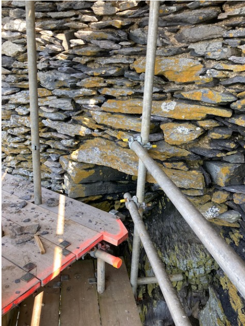
Fig. 9. Opening of drain from toilet House 2.
