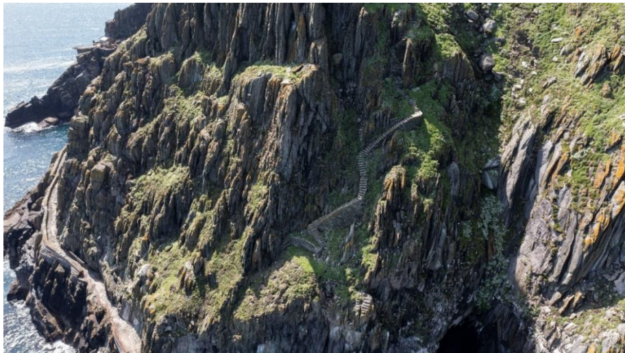
Figure 19 - View of the East Steps
