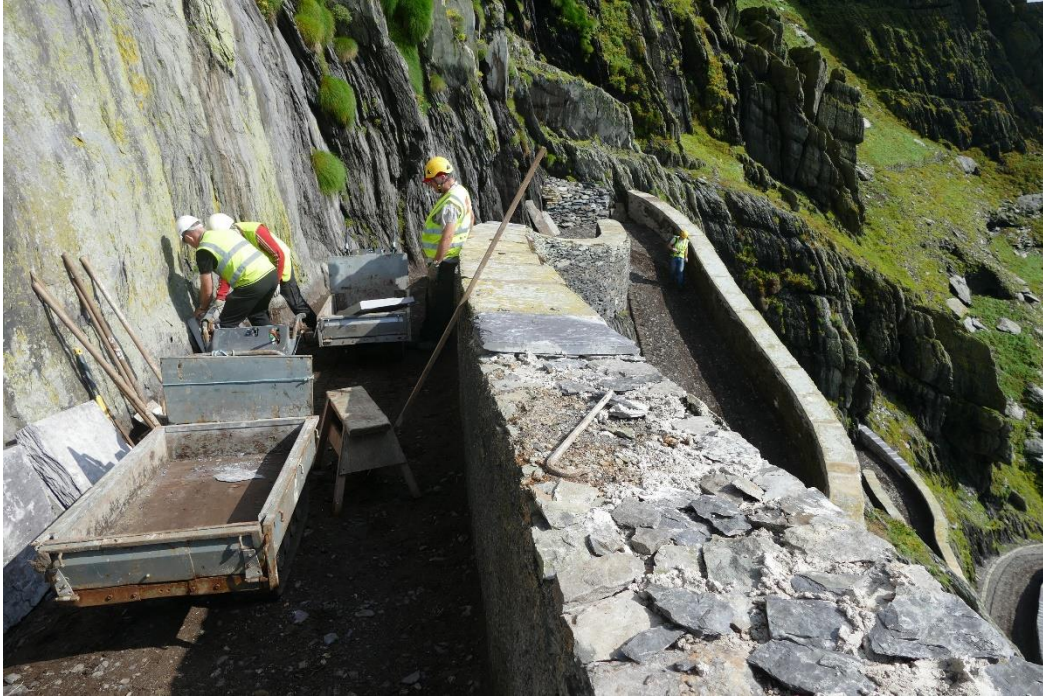
Figure 34 – Mechanical machinery on the island
