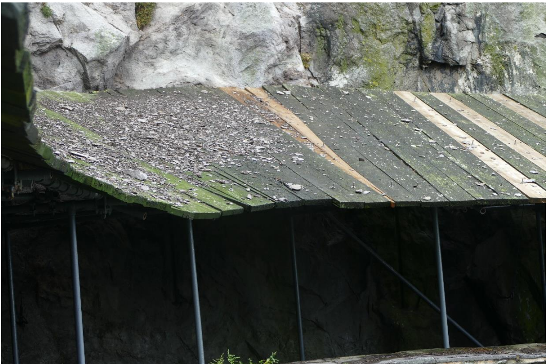
Figure 11 - View of fallen debris on the decking of the protective canopy on the Lower Lighthouse Road
