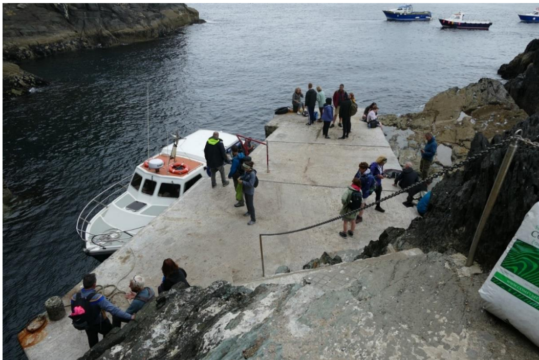
Figure 4 - View of the Landing Pier
