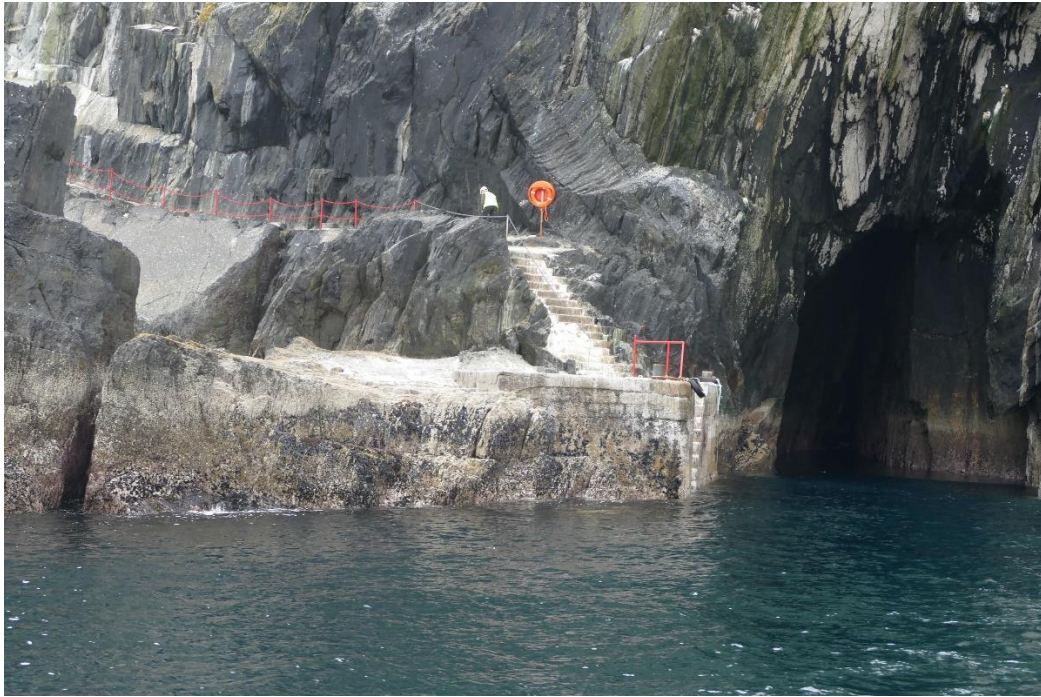
Figure 3 - View of the Landing Pier
