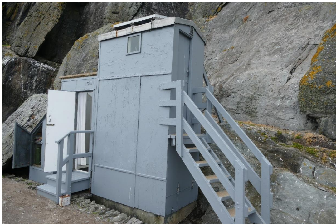
Figure 28 - View of the composting toilet used by OPW guides located on the Lower Lighthouse Road
