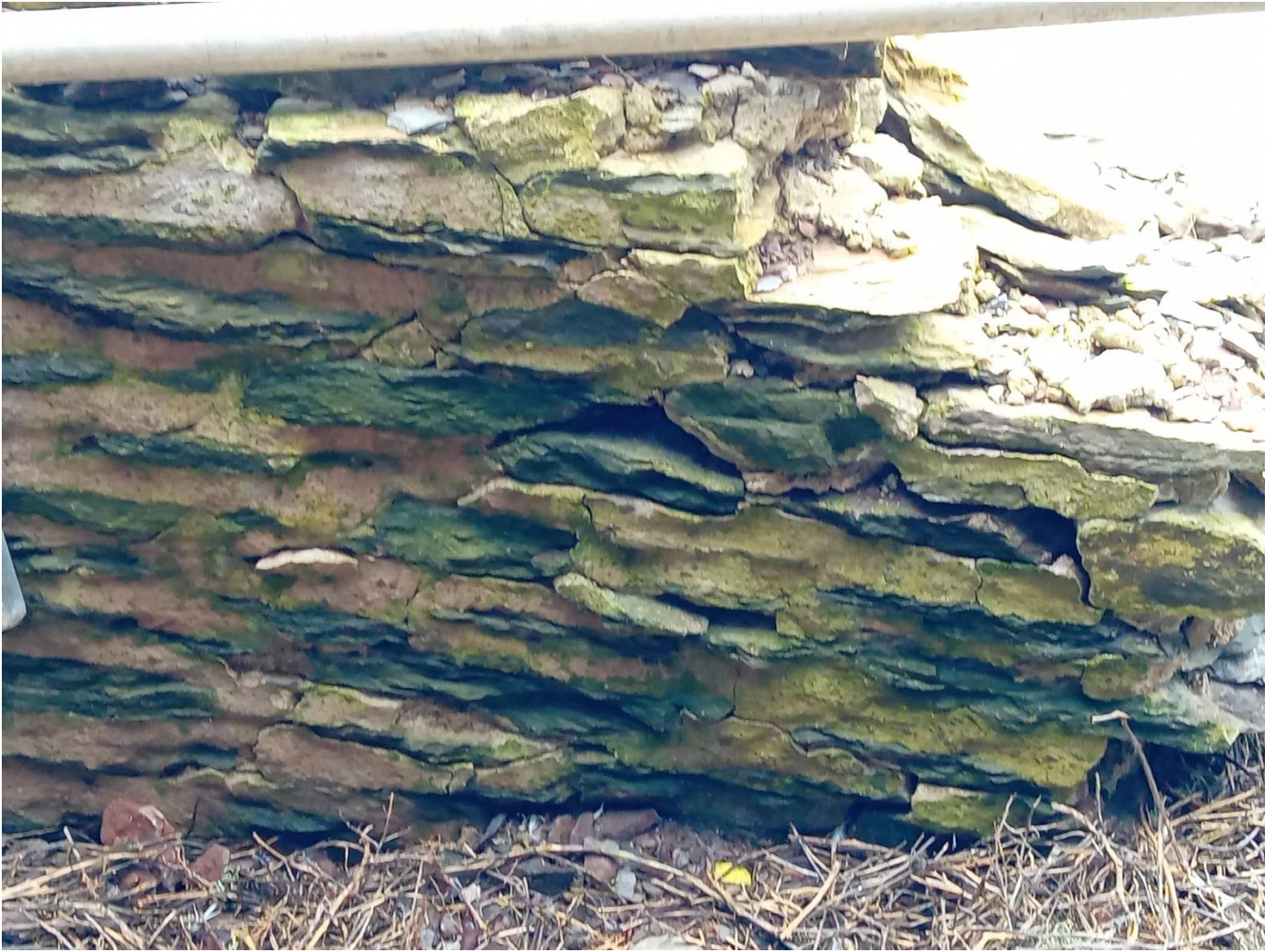
Photo 4: Tightly packed wall with lime mortar pointing at damaged wall location
