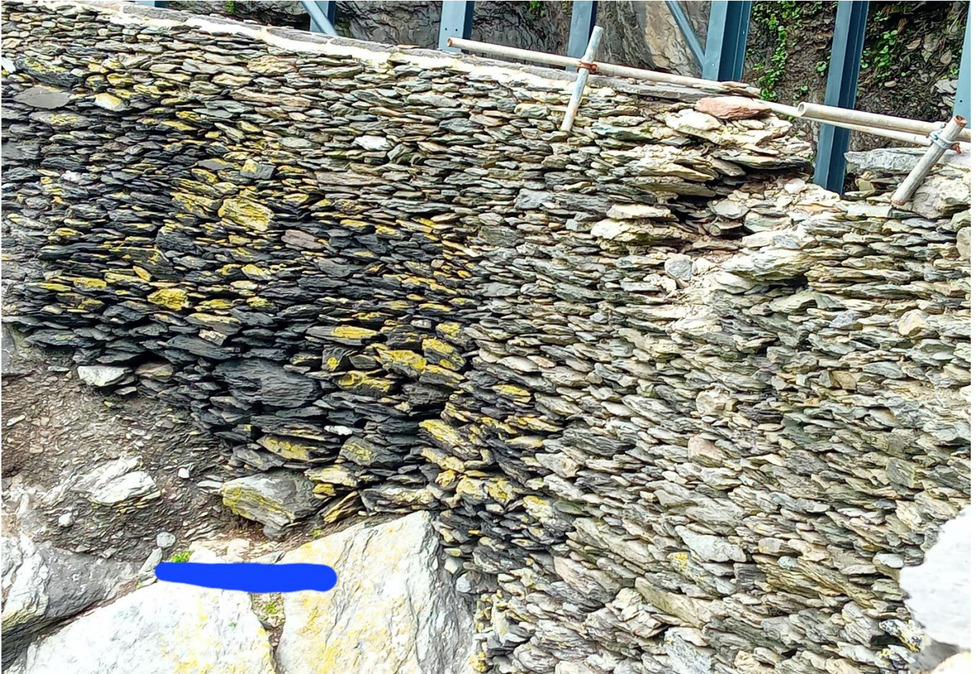
Photo 3: Damaged section of sea wall from rockfall near Crash Deck No. 2
