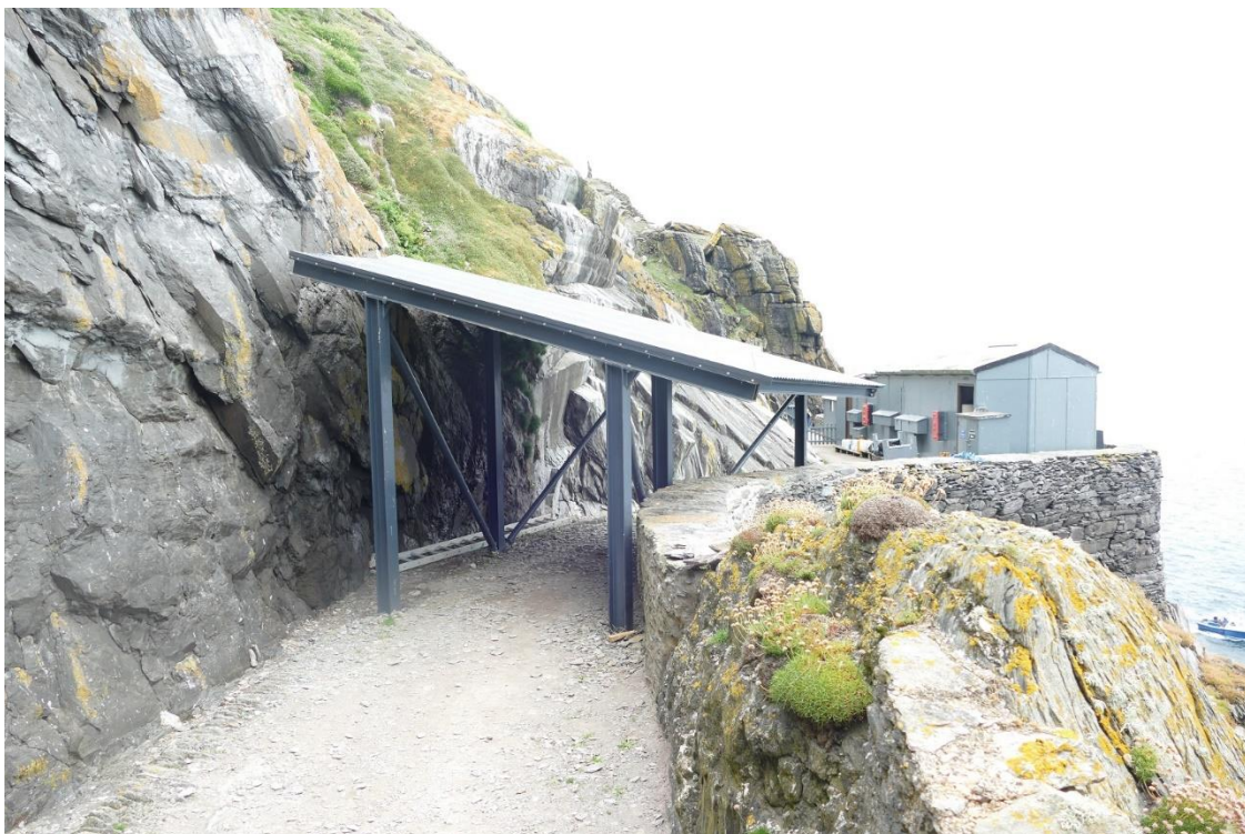
Figure 359 - Crash Deck No. 1 installed on site
