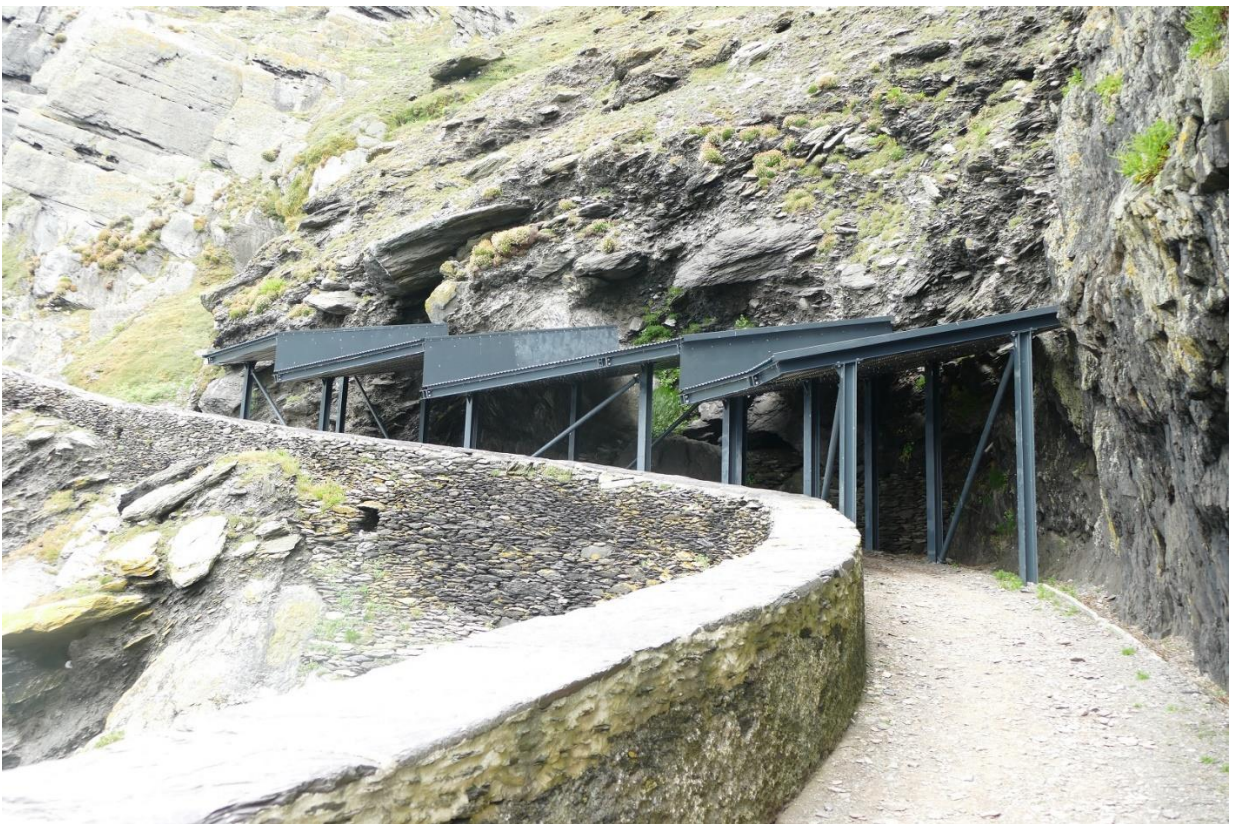
Figure 41 - Crash Deck No. 3 installed on site
