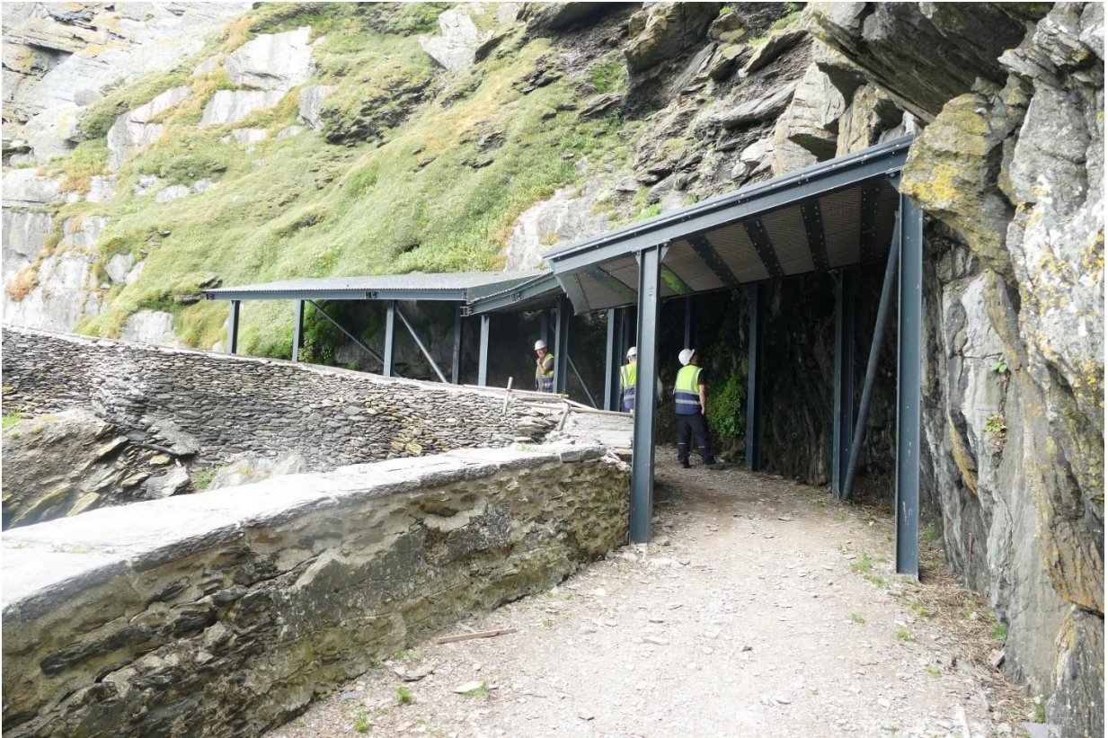
Figure 36 - Crash Deck No. 2 installed on site
