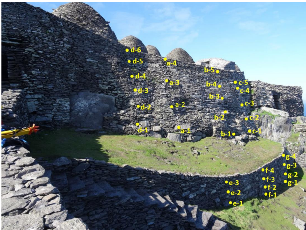
Figure 11 - Discovery Programme marker point locations at monastery retaining wall
