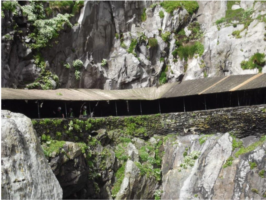
Figure 1. Upper end of walkway, showing replaced boards at right.
