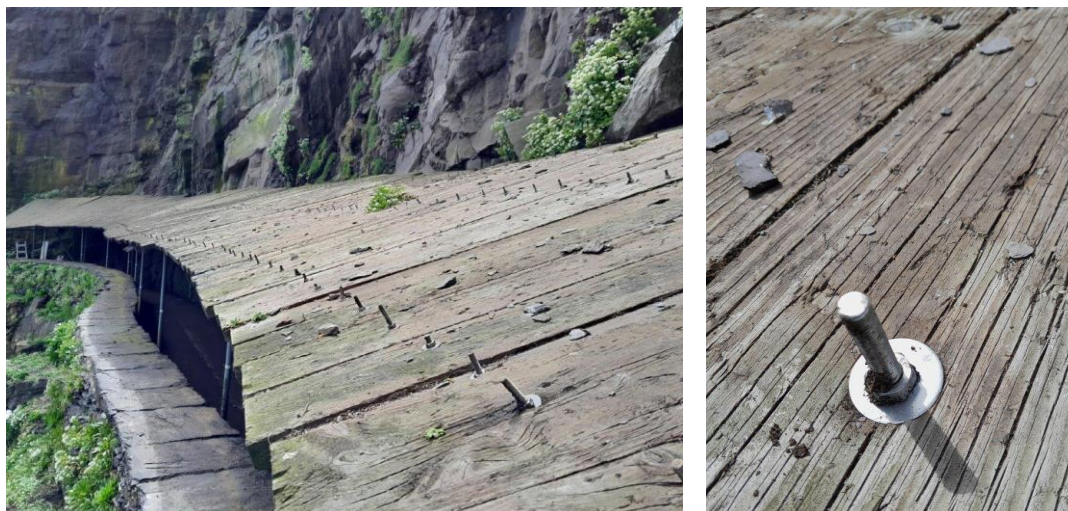
OPW Image: Context and detail of exposed 'J' Bolts
