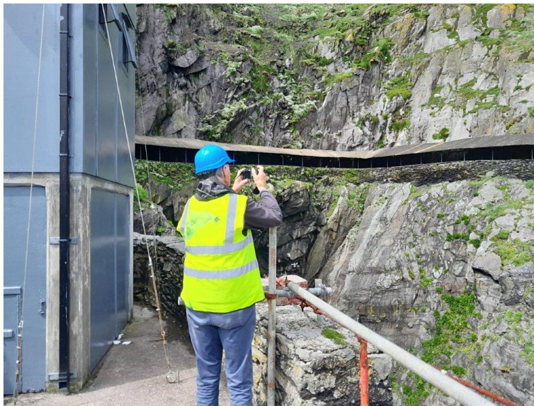
OPW Image: Survey scanning of boarding in progress on site
