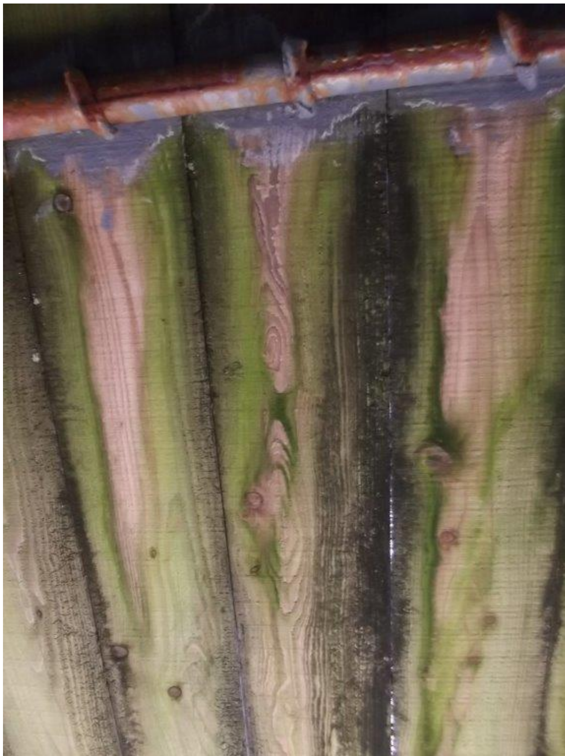
Figure 3. Underside of boards installed in 2016.
