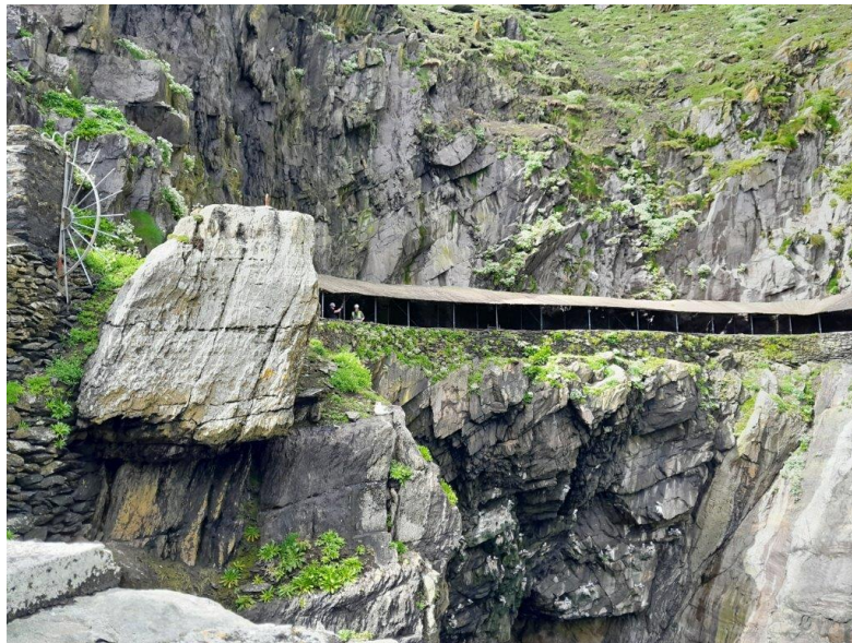
OPW Image: View from Heli-Pad Compound - Phase 1 of Cross Cove Crash Deck
