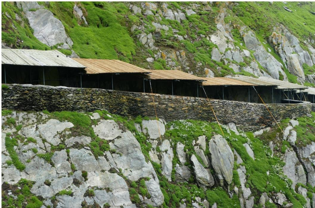
*Figure 28 - Repairs completed to the 2016 section of the timber protection canopy at Cross Cove*
