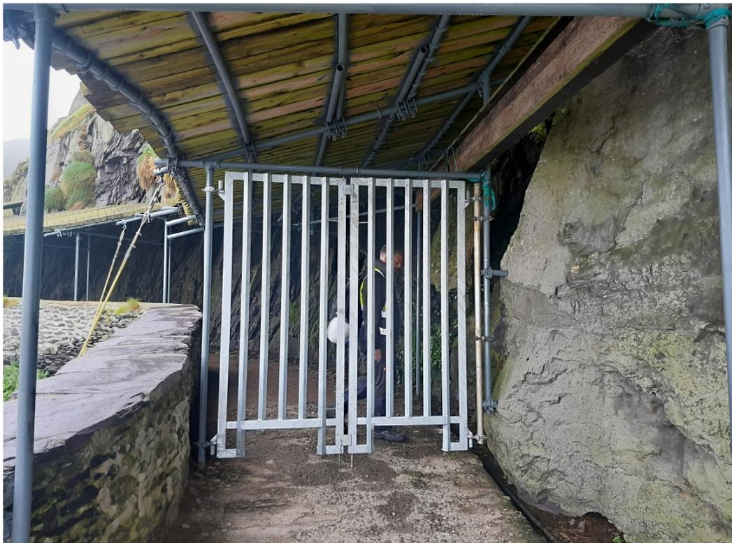
*Figure 33 - View of the new security gate installed at the end of bay of the timber protection canopy at Cross Cove*
