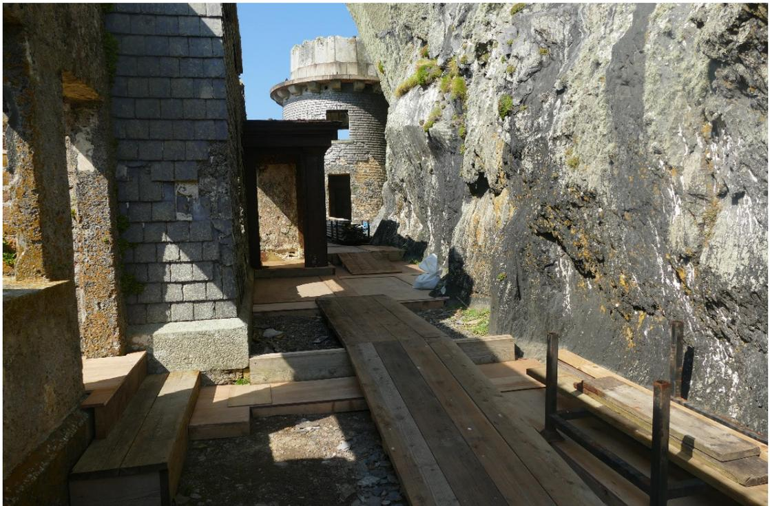
*Figure 19 - View of the new installed plywood protection to the existing floor at the upper lighthouse*
