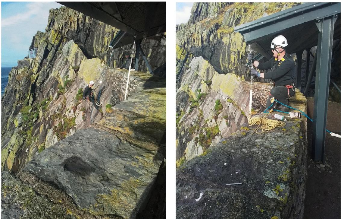
*Figure 29 - Re-instatement of the stainless steel stays to the 3 no. crash decks in September 2025*
