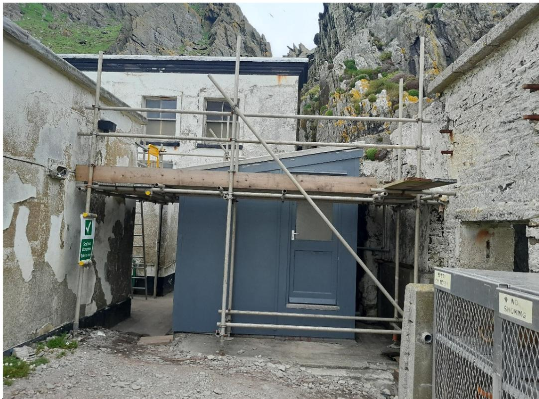
Figure 16 - Installation of the temporary workers composting toilet in the Lower Lighthouse compound
