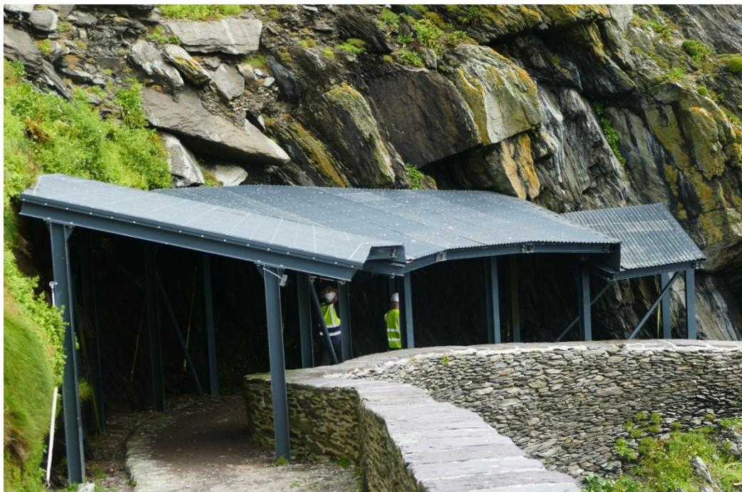
*Figure 31 - Repair and maintenance works carried out to the metal decking of the crash decks*
