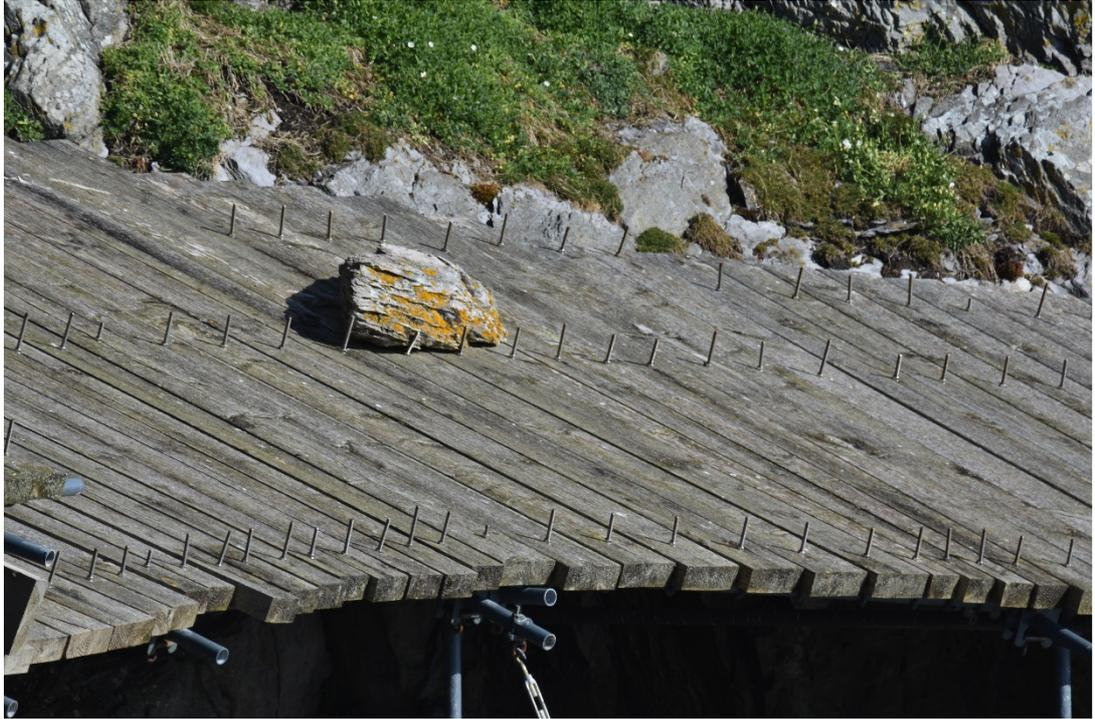
*Figure 25 - Rock fall on the timber protection canopy at Cross Cove*
