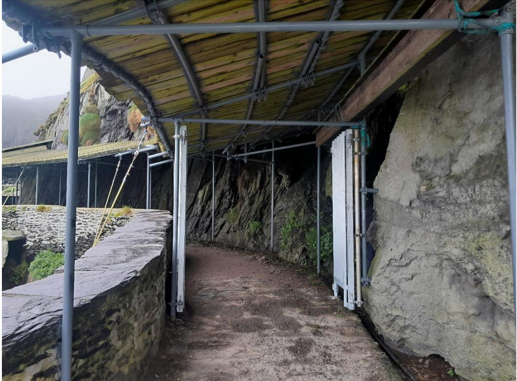
*Figure 32 - View of the new security gate installed at the end of bay of the timber protection canopy at Cross Cove*
