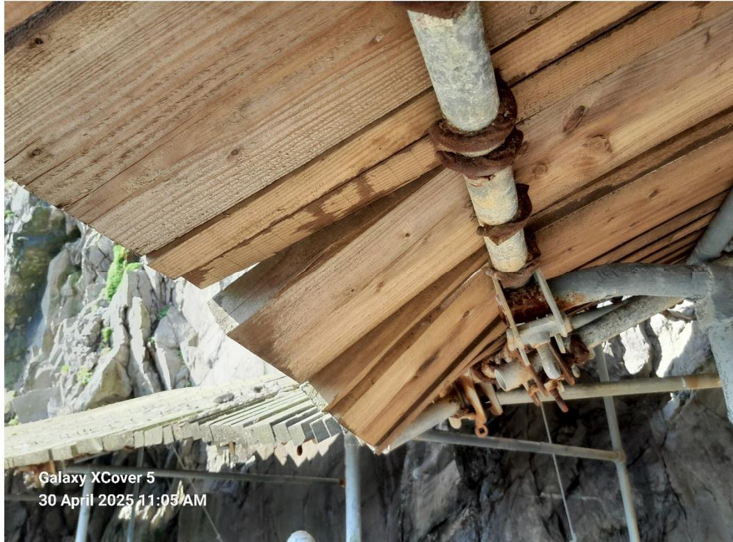
*Figure 27 - Damage from rock fall to the timber protection canopy at Cross Cove*
