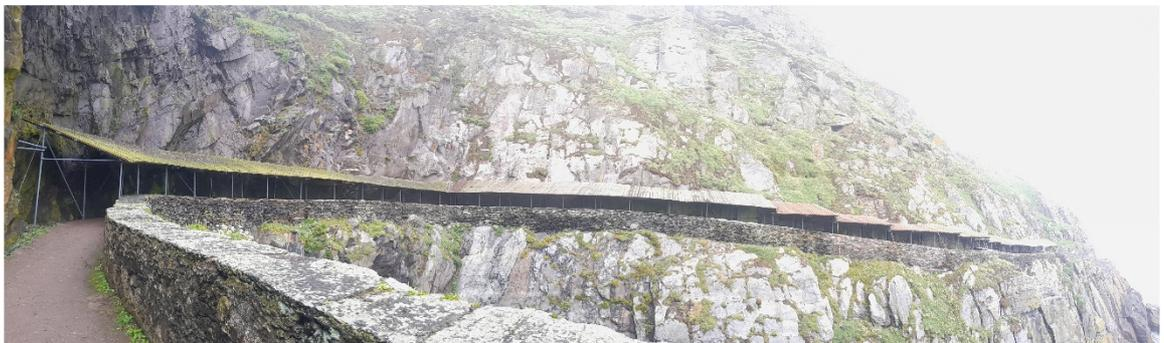
*Figure 24 - View of the protection timber canopy at Cross Cove*
